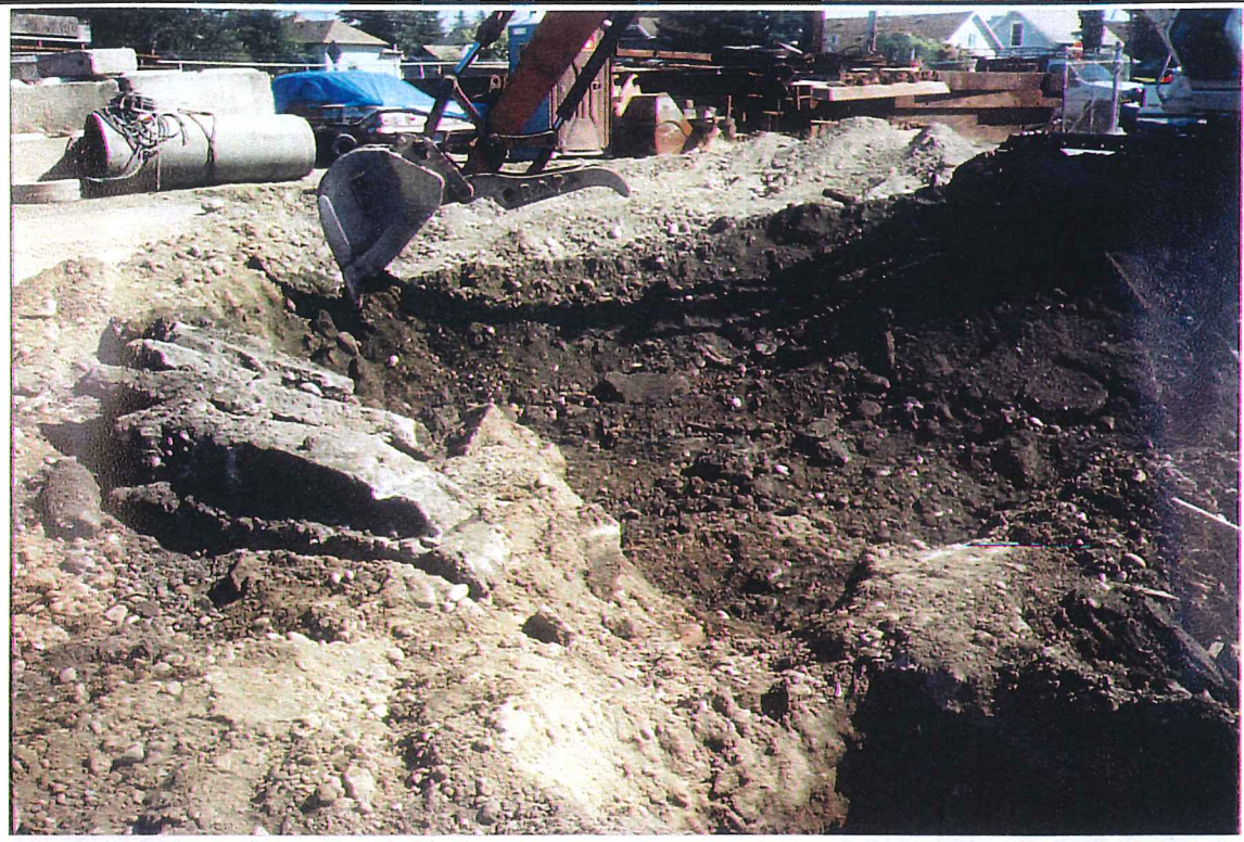
Photo #16: Photograph depicting the types of soil (fill) unearthed on the subject property, facing southwest. From the foreground; peaty soil, clean sandy gravel fill, heavy oil contaminated fill, blue-grey PAH contaminated fill, and cinders. Photo taken on 8/29/01.
