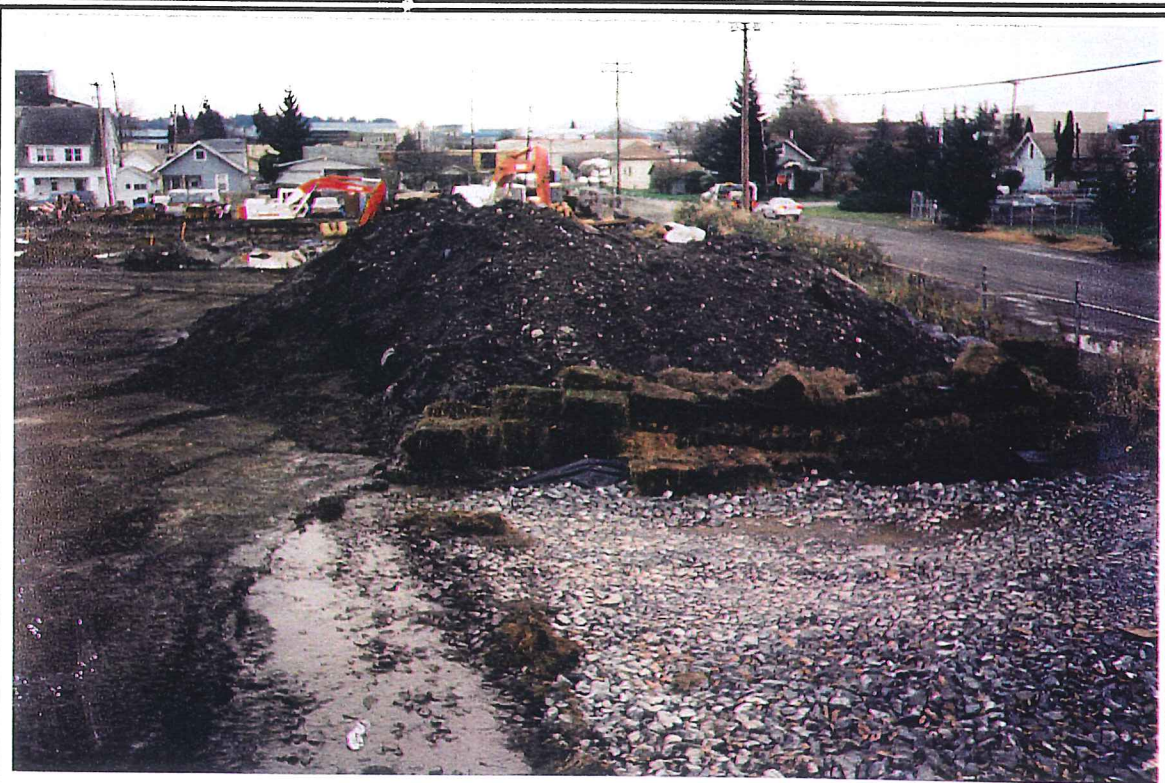
Photo #40: View of contaminated fill material in stockpile #4 prior to loading and transporting to TPS Technologies, Inc. for disposal, facing east. Photo taken on 12/20/01.
