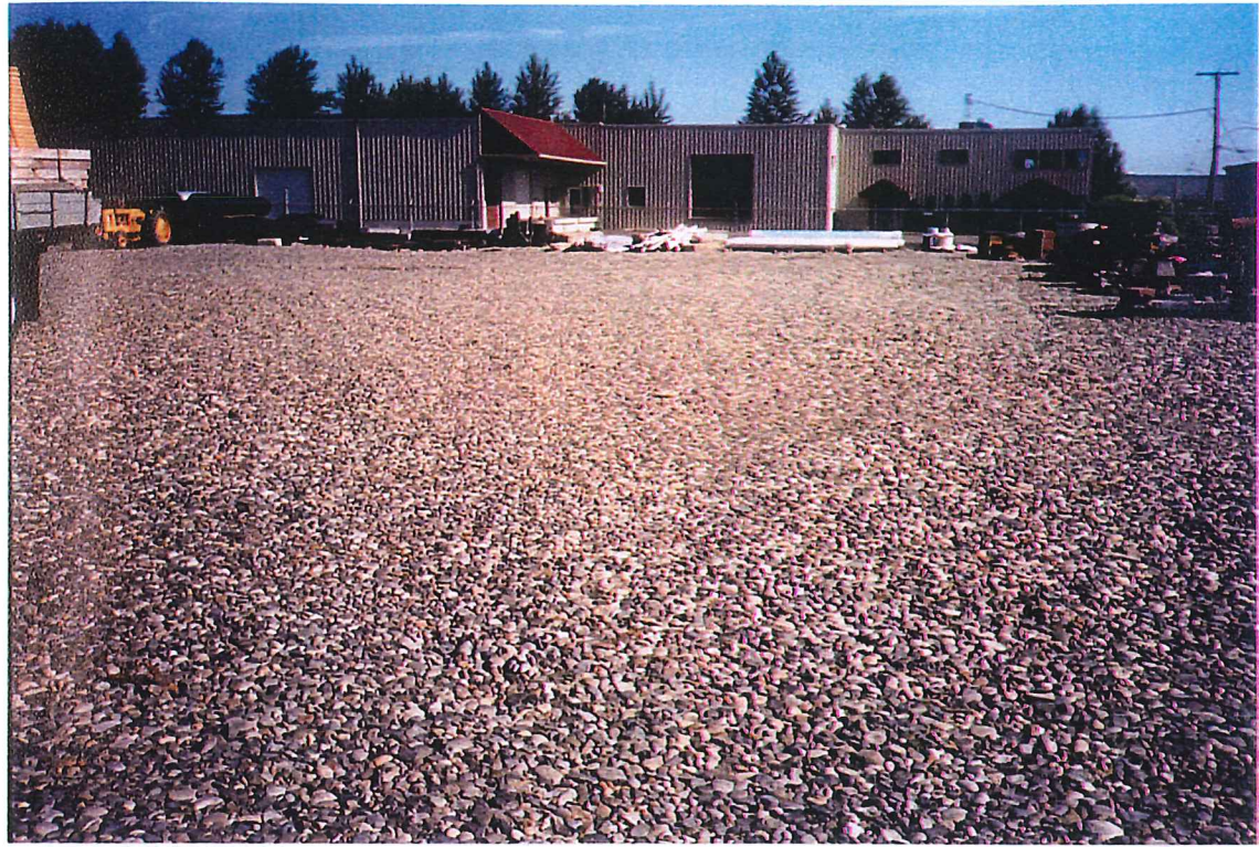
Photo #44: View of approximately 1 to 2 feet of crushed rock placed and graded over the Custom-Bilt Metals yard, facing northeast. Photo taken on 6/20/02.
