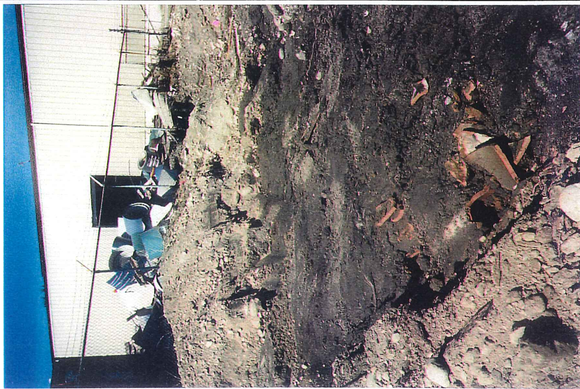
Photo #28: Clay sewer or stormwater drainage pipe unearthed near the northwest corner of the Westwater Construction site, facing northwest. Photo taken on 9/10/01.
