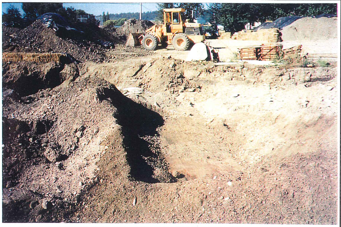
Photo #26: Photograph depicting light brown to grey cinders, facing west. The cinders were located adjacent to and beneath the two concrete slabs near the west boundary of the Westwater Construction site. The cinders were very light and porous. Photo taken on 9/10/01.
