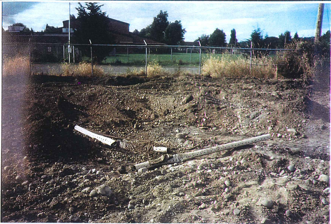
Photo #20: Unearthed industrial related debris (clay drainage pipe, brick, concrete, metal pipes), and petroleum hydrocarbon and PAH contaminated fill material located north of the removed gasoline underground storage tank on the Westwater Construction site, facing northeast. Photo taken on 8/31/01.
