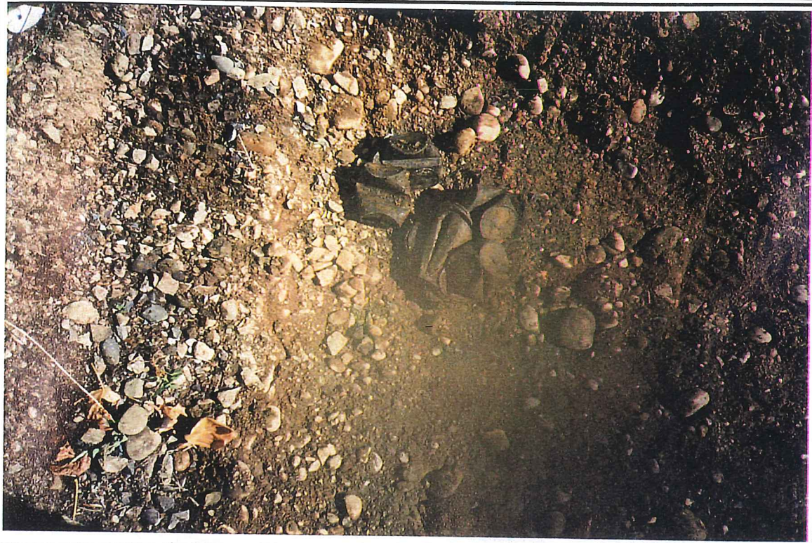
Photo #32: Photograph depicting the approximate 1 to 1-1/2 foot thick layer of clean fill material placed on top of the petroleum hydrocarbon/PAH contaminated fill, facing northwest. The clean fill was scraped off, stockpiled, tested, and used as backfill on the site. Photo taken on 9/10/01.
