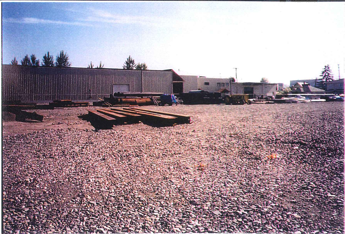
Photo #44: View of approximately 1 to 2 feet of crushed rock placed and graded over the Custom-Bilt Metals yard, facing northeast. Photo taken on 6/20/02.
