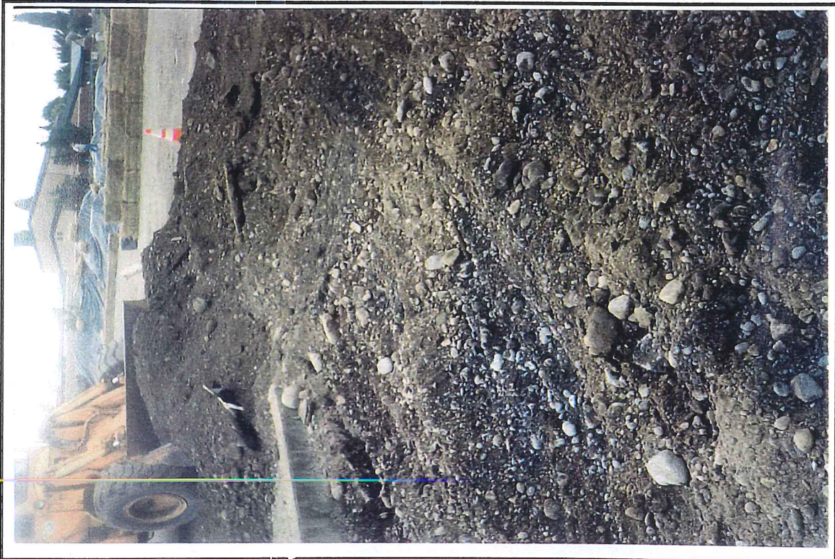
Photo #24: PAH contaminated fill material, (blue-grey color), scraped away adjacent to the west of the concrete "up ramp" located south of the Custom-Bilt Metals building, facing south. Photo taken on 9/4/01.
