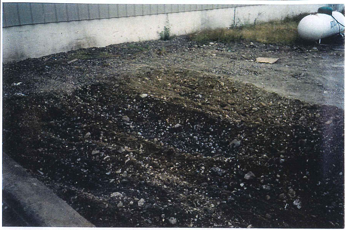
Photo #24: PAH contaminated fill material, (blue-grey color), scraped away adjacent to the west of the concrete "up ramp" located south of the Custom-Bilt Metals building, facing south. Photo taken on 9/4/01.
