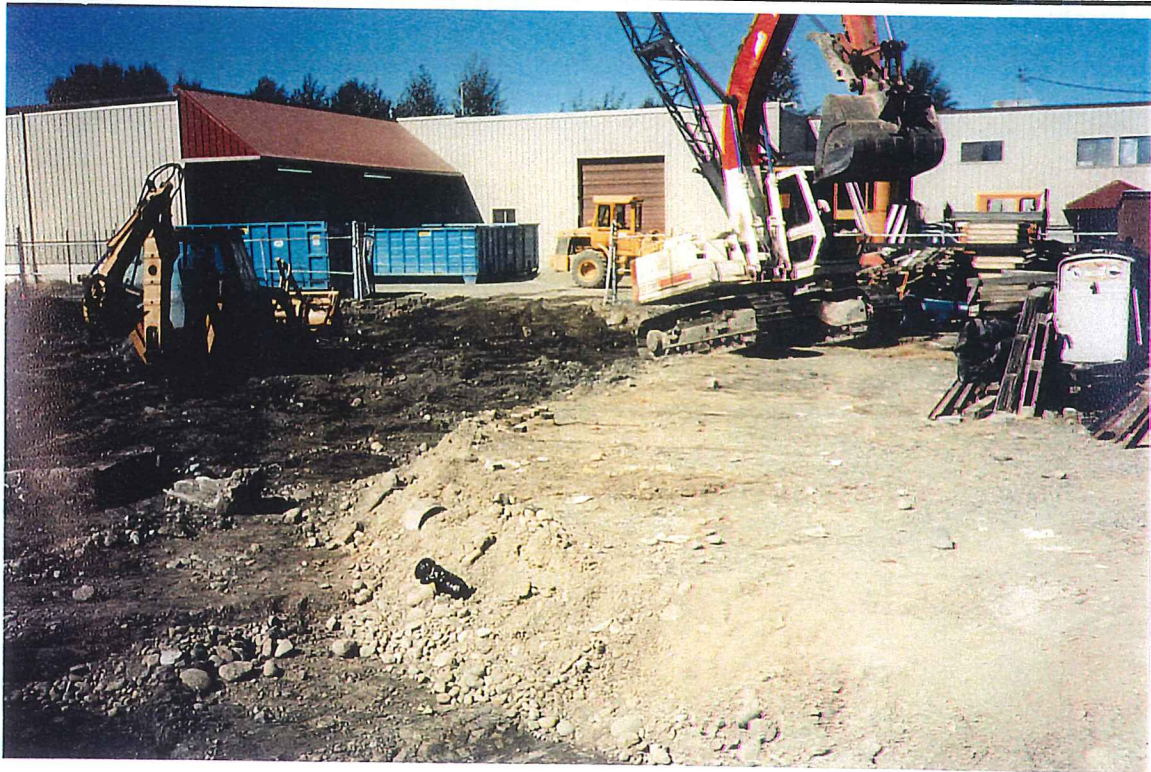
Photo #32: Photograph depicting the approximate 1 to 1-1/2 foot thick layer of clean fill material placed on top of the petroleum hydrocarbon/PAH contaminated fill, facing northwest. The clean fill was scraped off, stockpiled, tested, and used as backfill on the site. Photo taken on 9/10/01.
