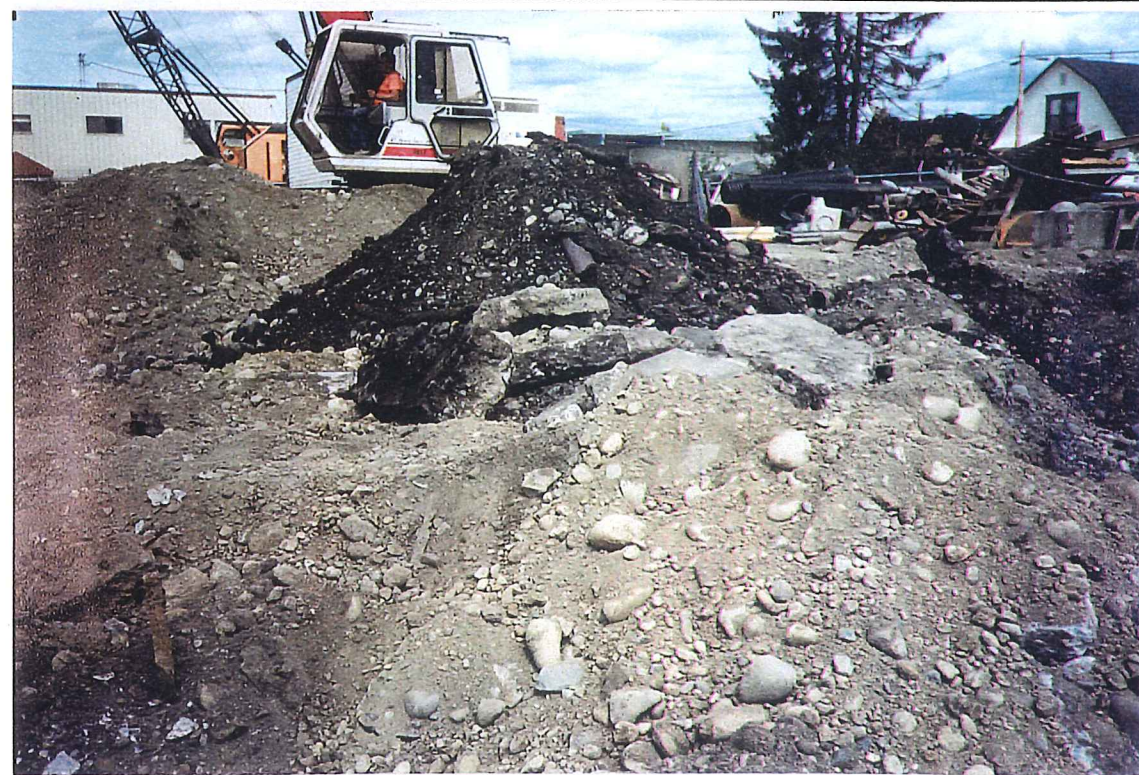
Photo #20: Unearthed industrial related debris (clay drainage pipe, brick, concrete, metal pipes), and petroleum hydrocarbon and PAH contaminated fill material located north of the removed gasoline underground storage tank on the Westwater Construction site, facing northeast. Photo taken on 8/31/01.
