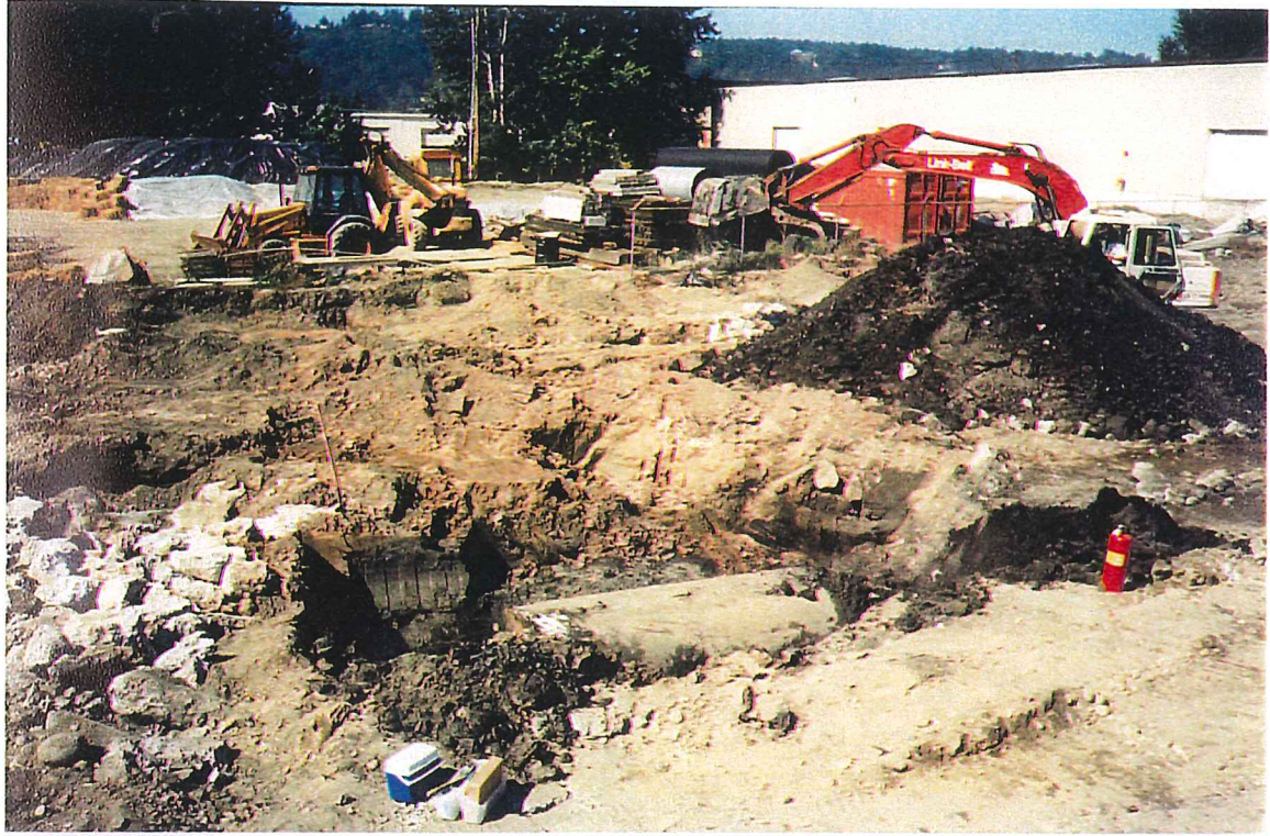
Photo #34: Photograph depicting soil/fill layer located adjacent to the foundation of the Custom-Bilt Metals building, facing west. Heavy oil contaminated soil was identified adjacent to the foundation (left of the red fire valve). Photo taken on 10/7/01.
