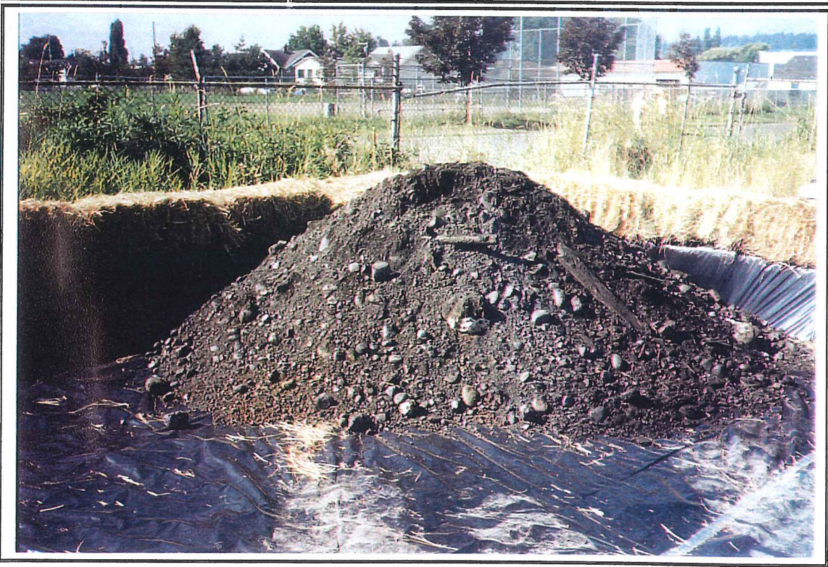
Photo #14: Photograph depicting the first load of contaminated fill material excavated from the subject property, facing southeast. This material was unearthed adjacent to the two concrete slabs on the Westwater Construction Site. Photo taken 8/29/01.
