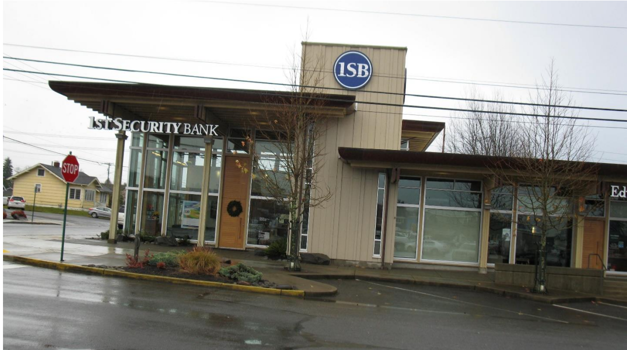
Photo 1: Current 1st Security Bank Building/Former Brumfield Twidwell – From the West.
