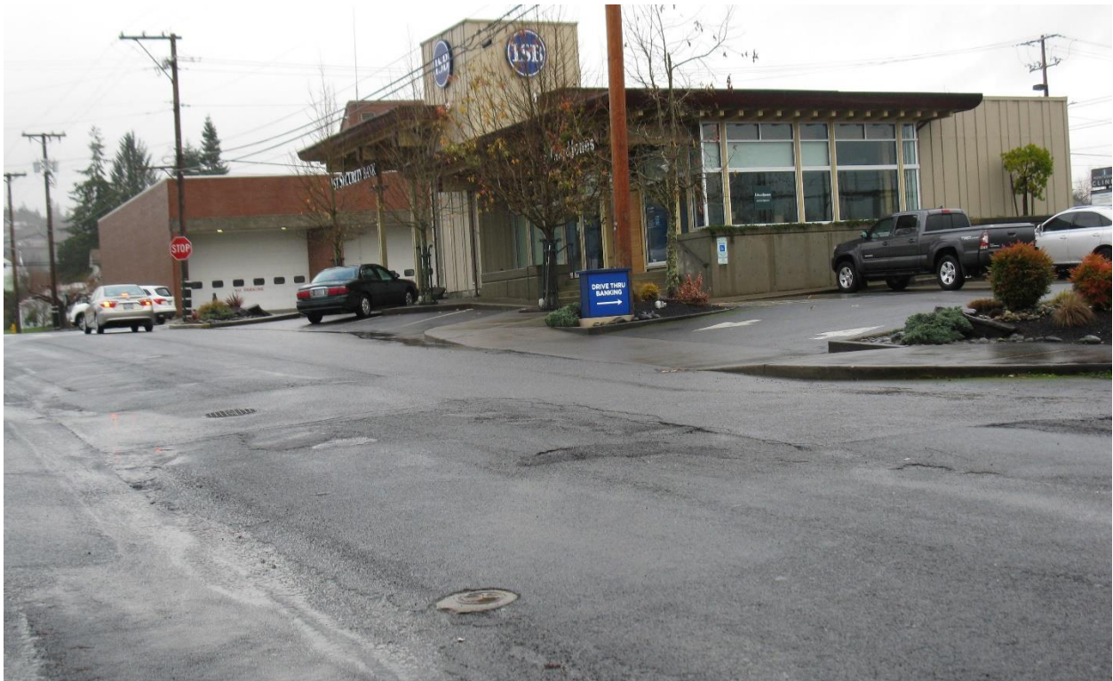
Photo 4: Current 1st Security Bank Building/Former Brumfield Twidwell and City of Montesano Fire Station (red building) and Sylvia Street – From the Southwest.
