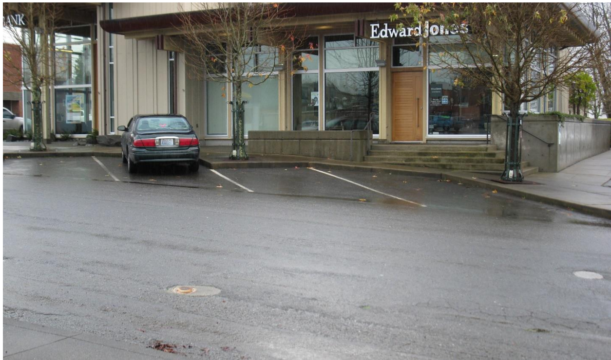
Photo 5: Abandoned Soil Boring and Groundwater Monitoring Well Locations on Sylvia Street – from the Southwest.
