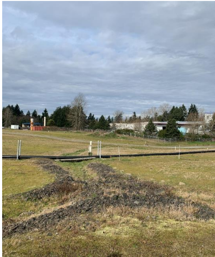
Stormwater conveyance on landfill
