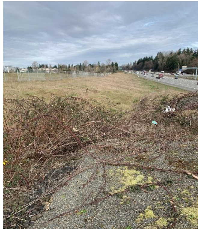
Area of settlement on landfill cap in area of future redevelopment
