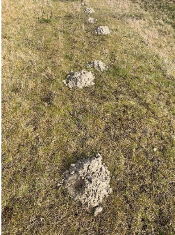
Evidence of burrowing into landfill cap by rodents
