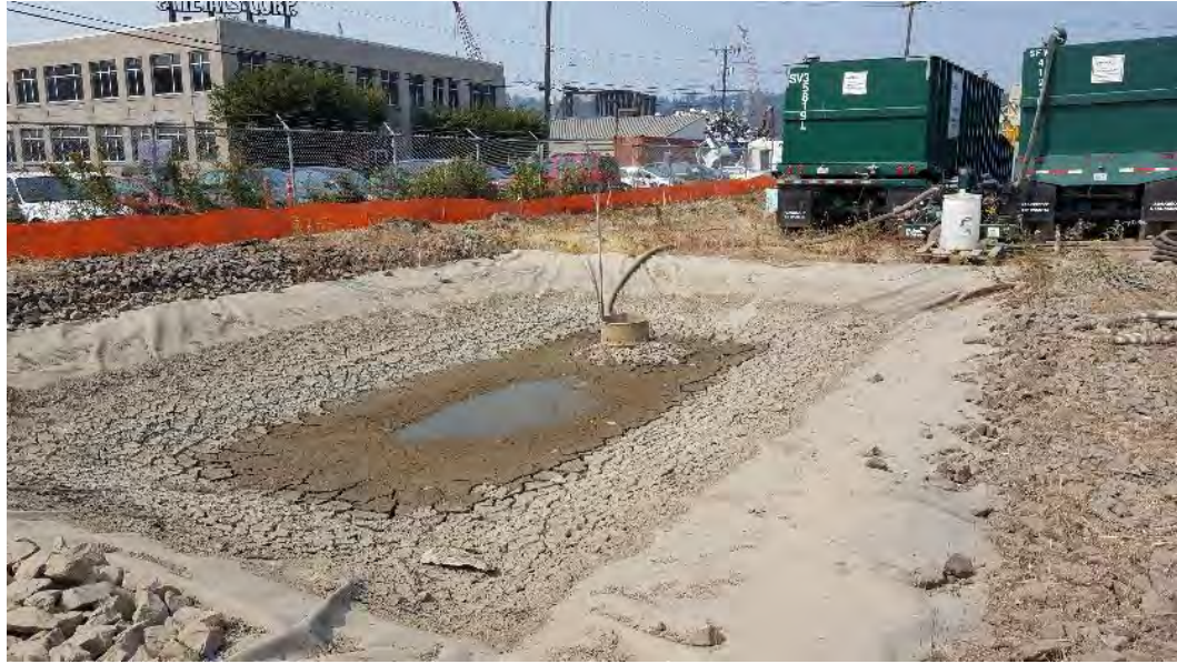
Photograph 1. Site controls: water holding tanks and silt fence
