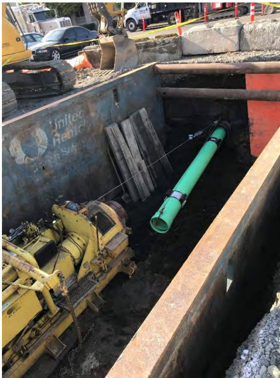
Photograph 32. Installation of pipe for final sewer connection
