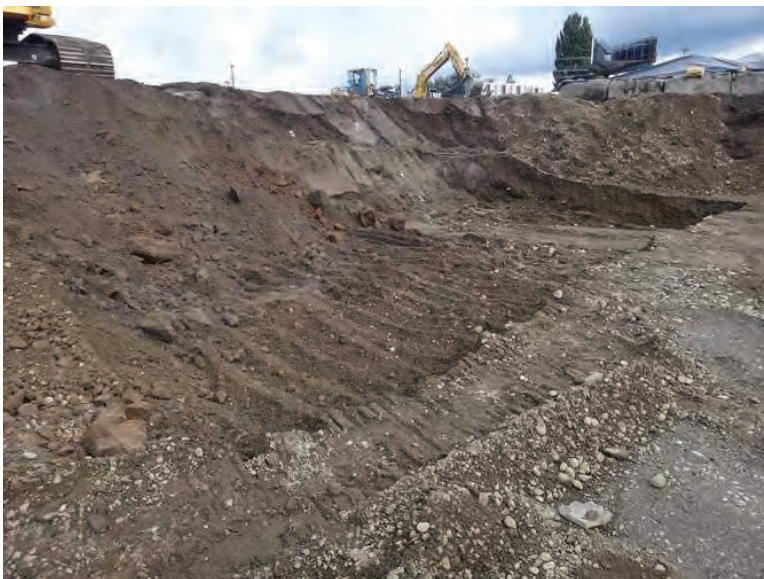
Photograph 1. Overview of Stoddard IA excavation into native sediments, looking northeast.
