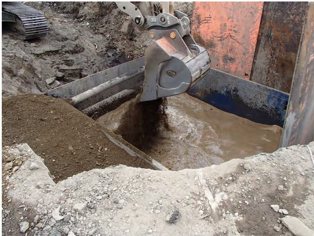
Photograph 10. Placement of import backfill below water table, Stoddard solvent excavation
