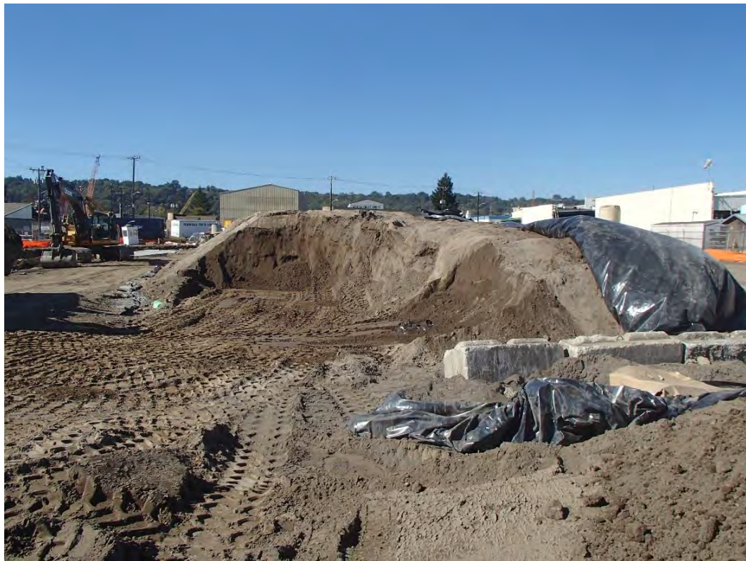
Photograph 20. Removal of portion of stockpile SP-02 for disposal
