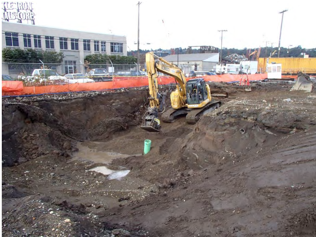
Photograph 17. Backfill compaction, Stoddard solvent excavation
