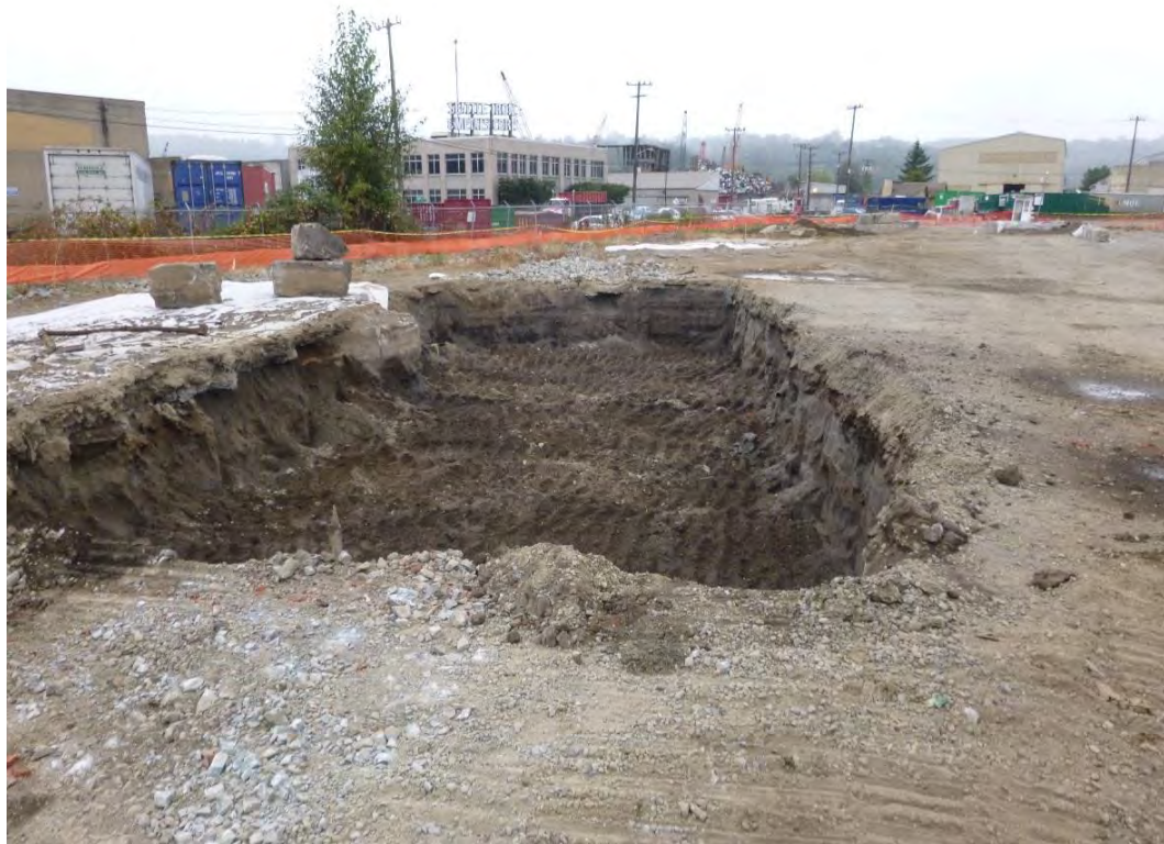
Photograph 4. Completed heavy oil-range organics focused excavation
