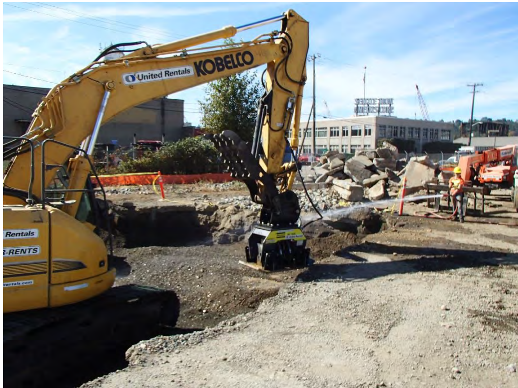
Photograph 12. Backfill compaction, heavy oil-range organics focused excavation
