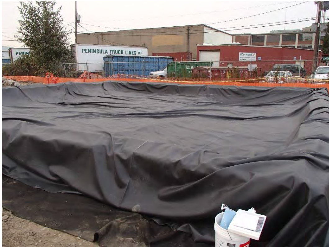
Photograph 7. Lined stockpile area for Stoddard solvent-contaminated soil
