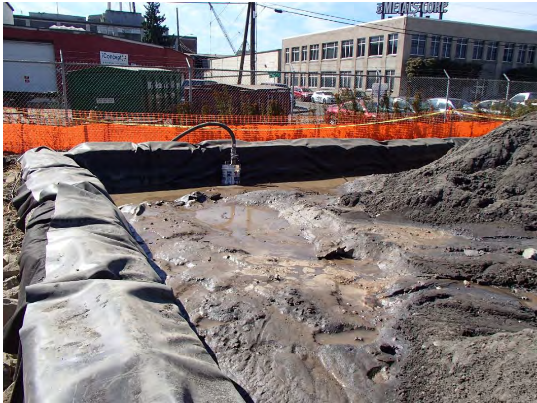
Photograph 13. Dewatering saturated Stoddard solvent-contaminated soil stockpile area
