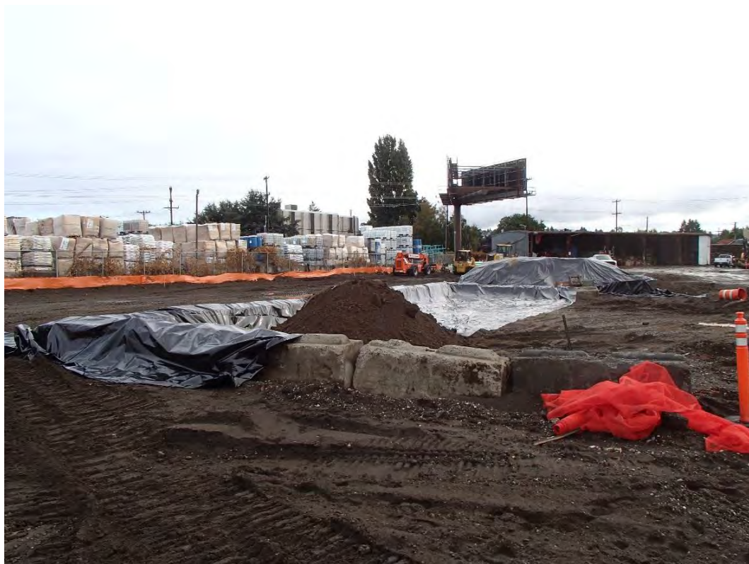
Photograph 18. Soil reuse stockpile, stormwater system trenching
