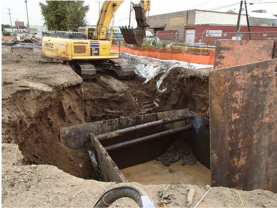
Photograph 9. Western portion of Stoddard solvent excavation
