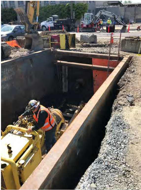
Photograph 31. Boring machine for jack-and-bore final connection to sewer
