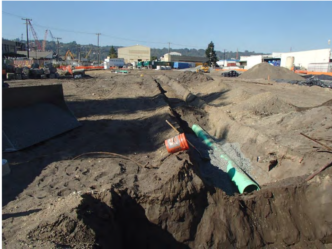
Photograph 23. Stormwater conveyance pipe trench and pipe bedding
