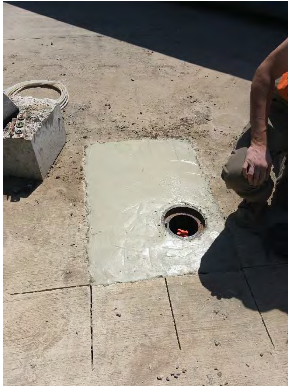
Photograph 33. Monitoring well restoration with heavy-duty monument
