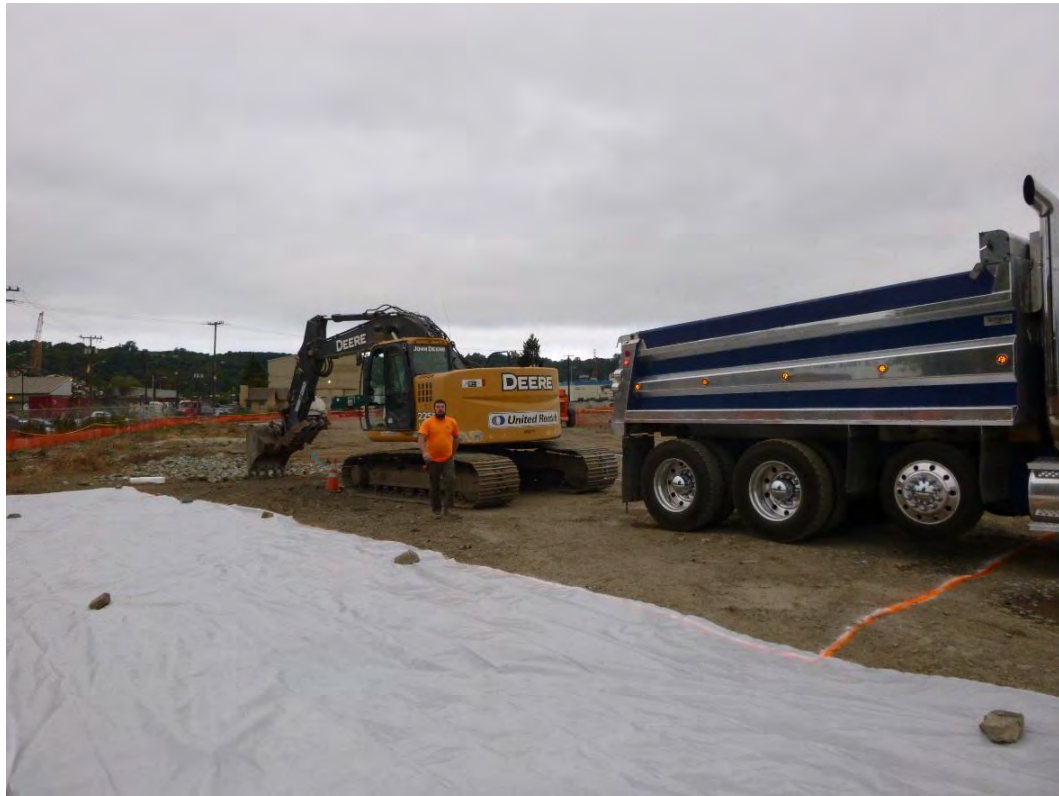
Photograph 3. Excavation and direct-loading, heavy oil-range organics focused excavation
