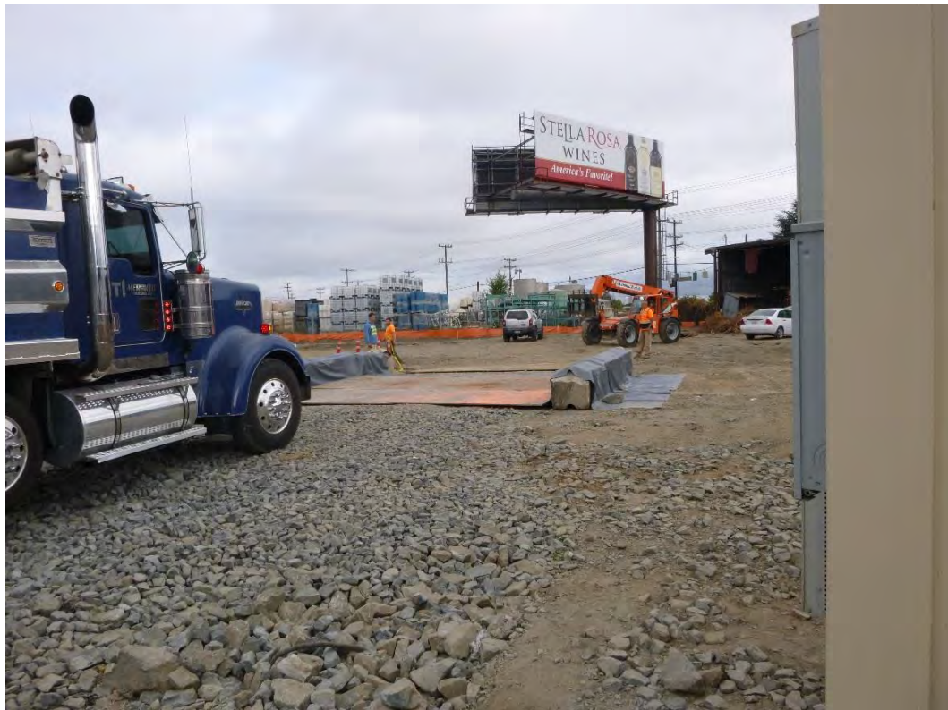
Photograph 2. Site controls: stabilized construction entrance
