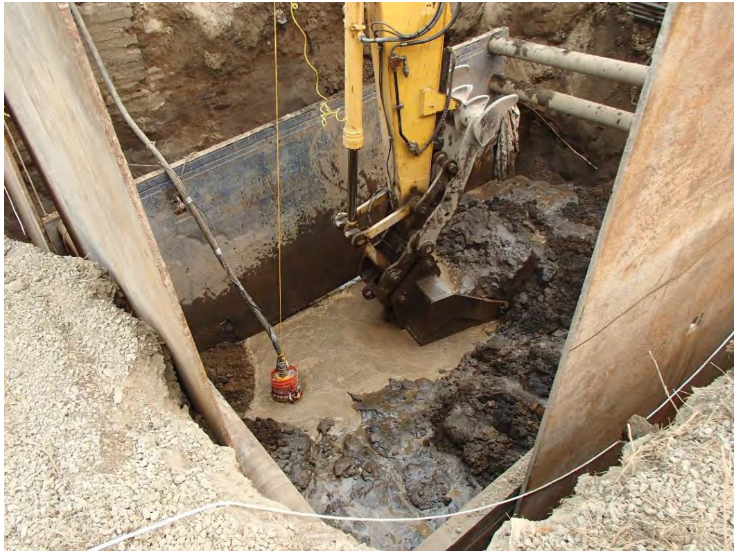
Photograph 8. Shored excavation below water table, Stoddard solvent excavation
