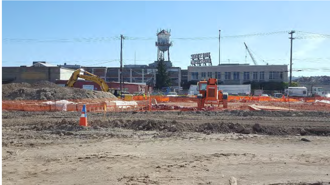
Photograph 11. View of onsite reuse stockpile and exclusion zone delineation
