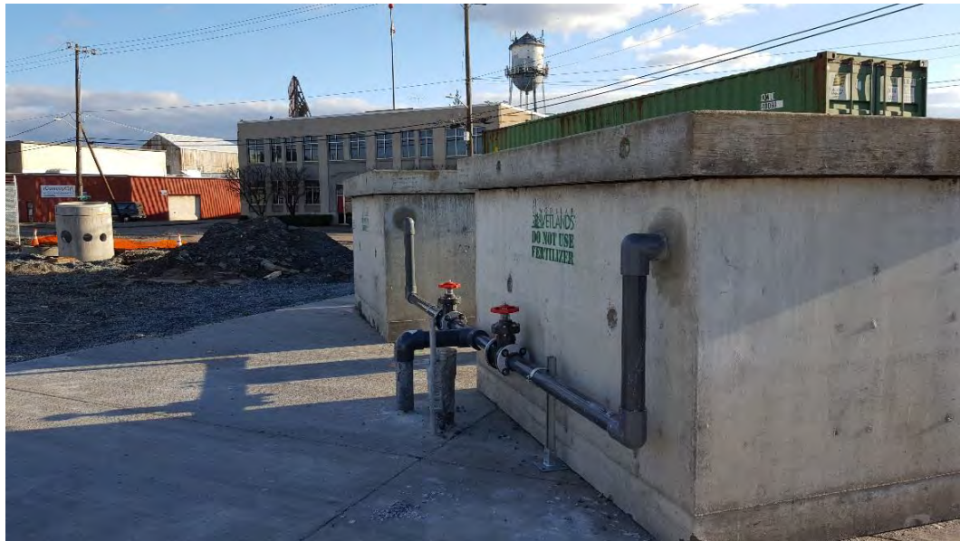
Photograph 30. Installation of modular wetlands treatment units
