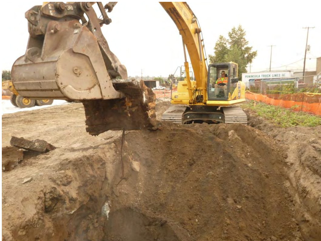
Photograph 6. Concrete foundation wall in shallow soil, Stoddard solvent excavation
