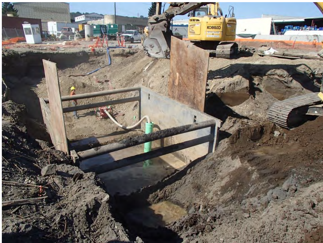
Photograph 14. Eastern portion of Stoddard solvent excavation
