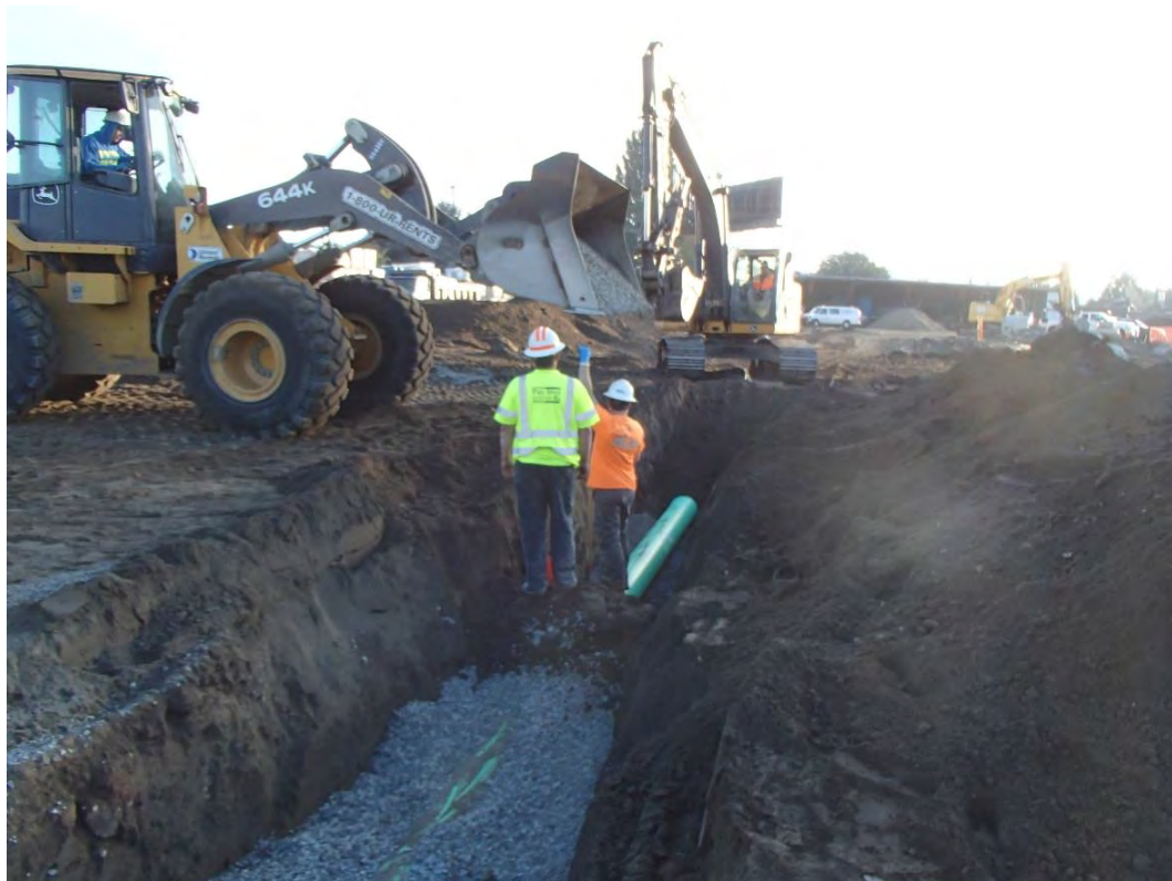
Photograph 22. Installation of stormwater conveyance pipe
