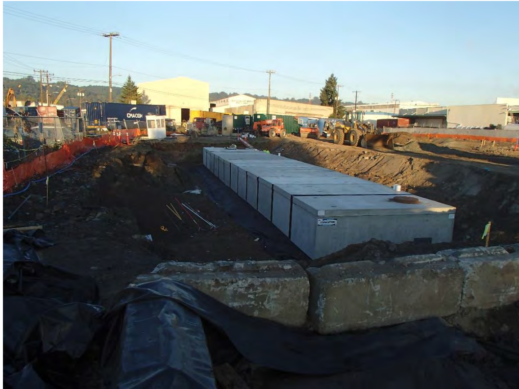
Photograph 21. Installation of StormCapture detention structure
