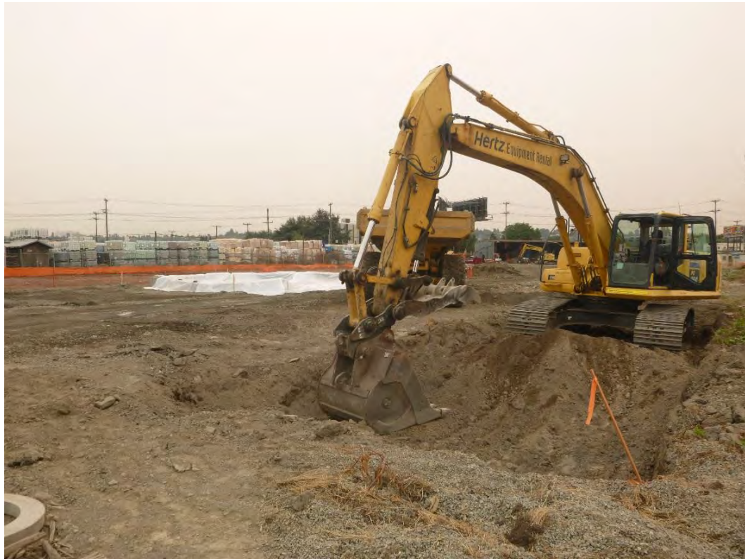
Photograph 5. Removal of clean overburden, Stoddard solvent excavation
