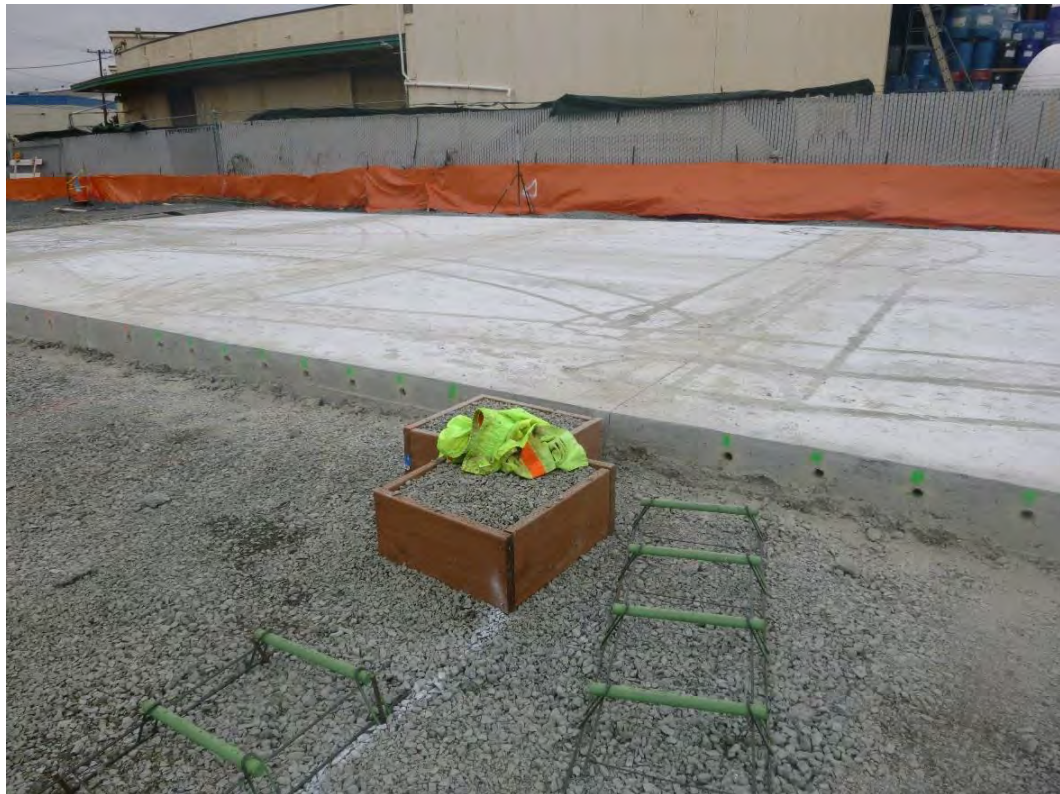
Photograph 28. Well protection during pavement
