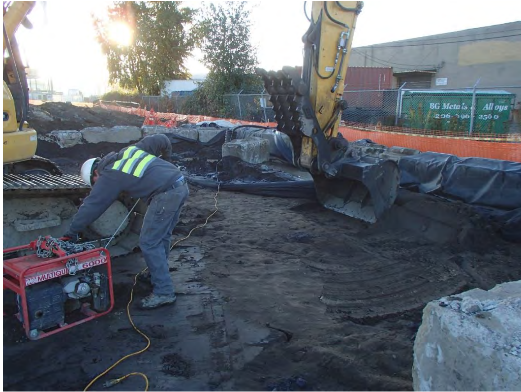
Photograph 19. Dismantling and disposal of Stoddard solvent-contaminated soil stockpile
