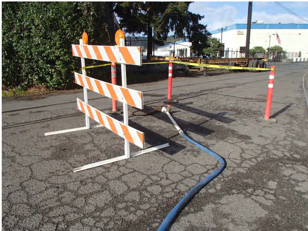
Photograph 24. Discharge of treated dewatering water to sewer
