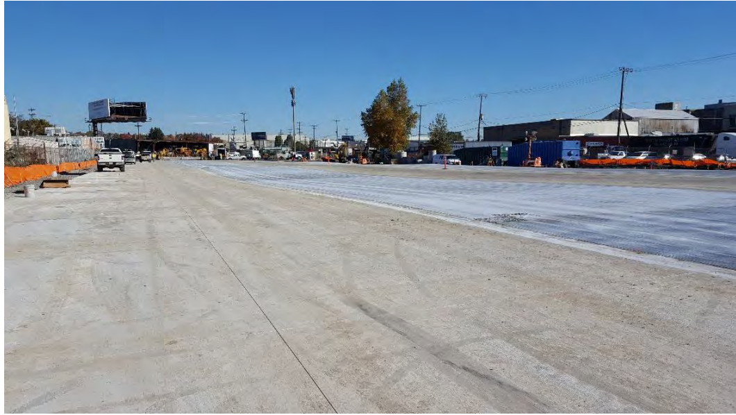
Photograph 29. Completed concrete pavement on northern portion of property
