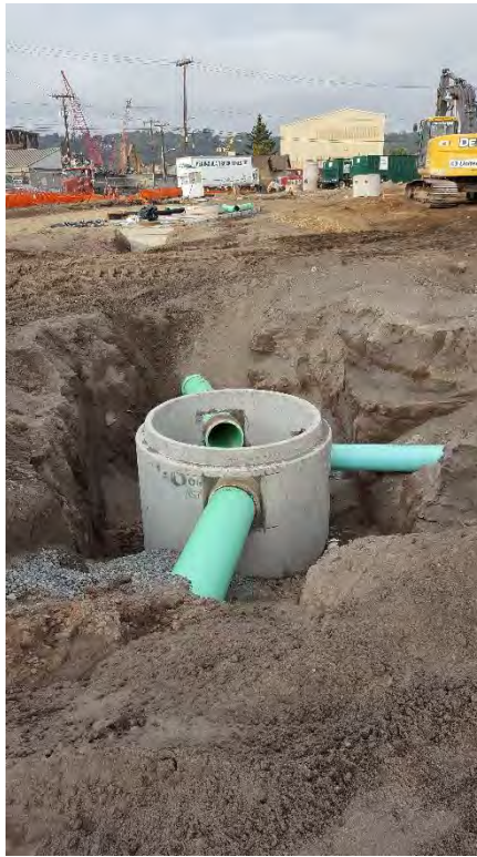
Photograph 25. Catch basin installation
