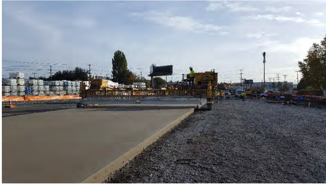
Photograph 27. Concrete pavement installation
