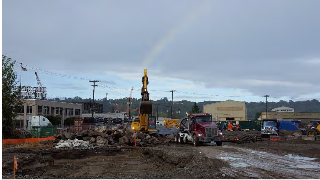
Photograph 15. Loading trucks from Stoddard solvent-contaminated soil stockpile
