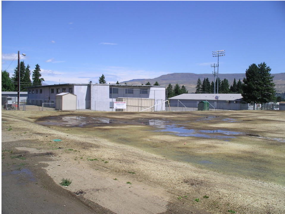
Photo D-3: West Side after remediation, grading and hydroseeding
