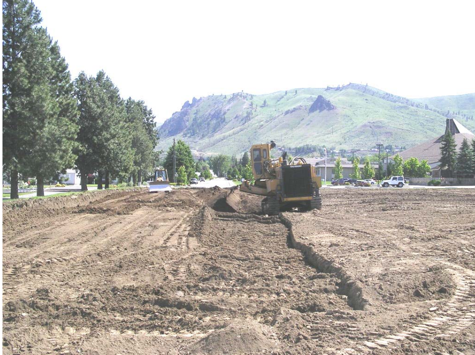
Photo D-1: Deep mixer in action at West Side
