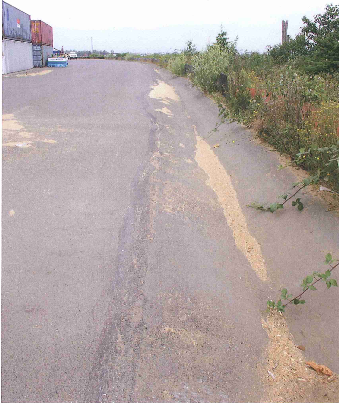
Photo 2: Sealed crack at ditch pavement overlap at east edge of cap.
