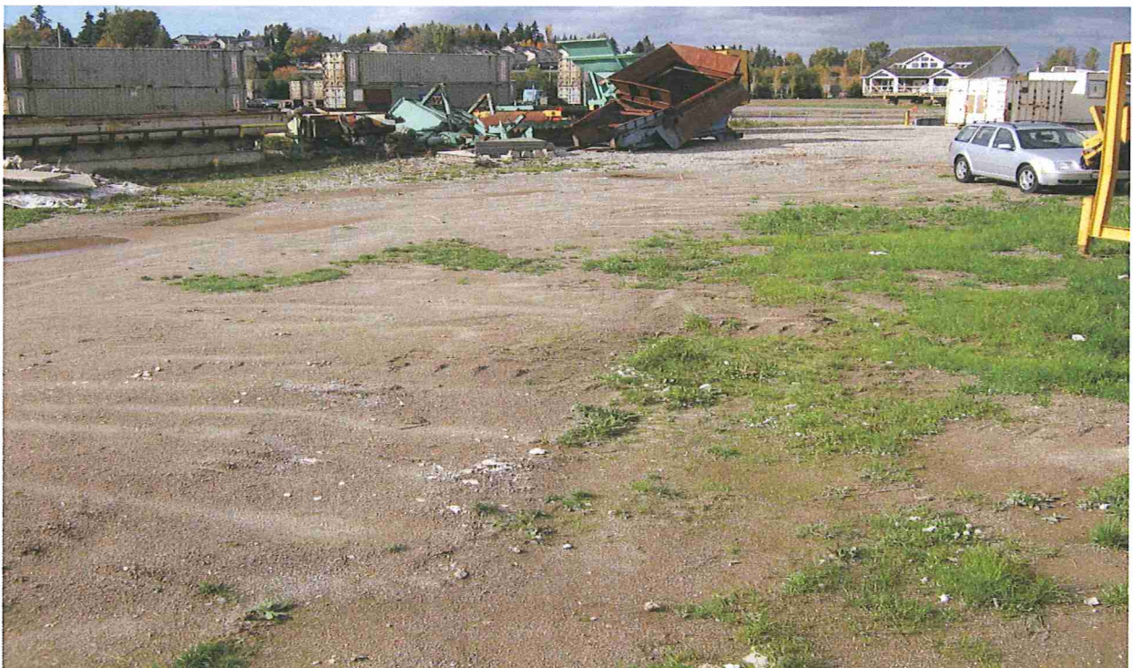
Photo 4: Soil cover area needing hydroseed
