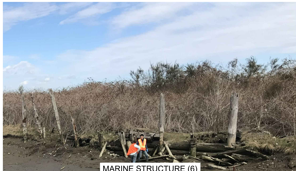
MARINE STRUCTURE (6) VIEW 1
