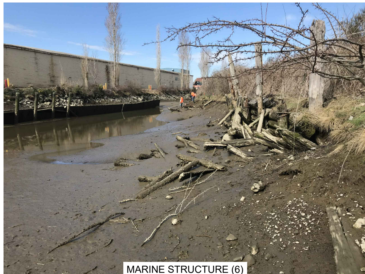
MARINE STRUCTURE (6) VIEW 2
