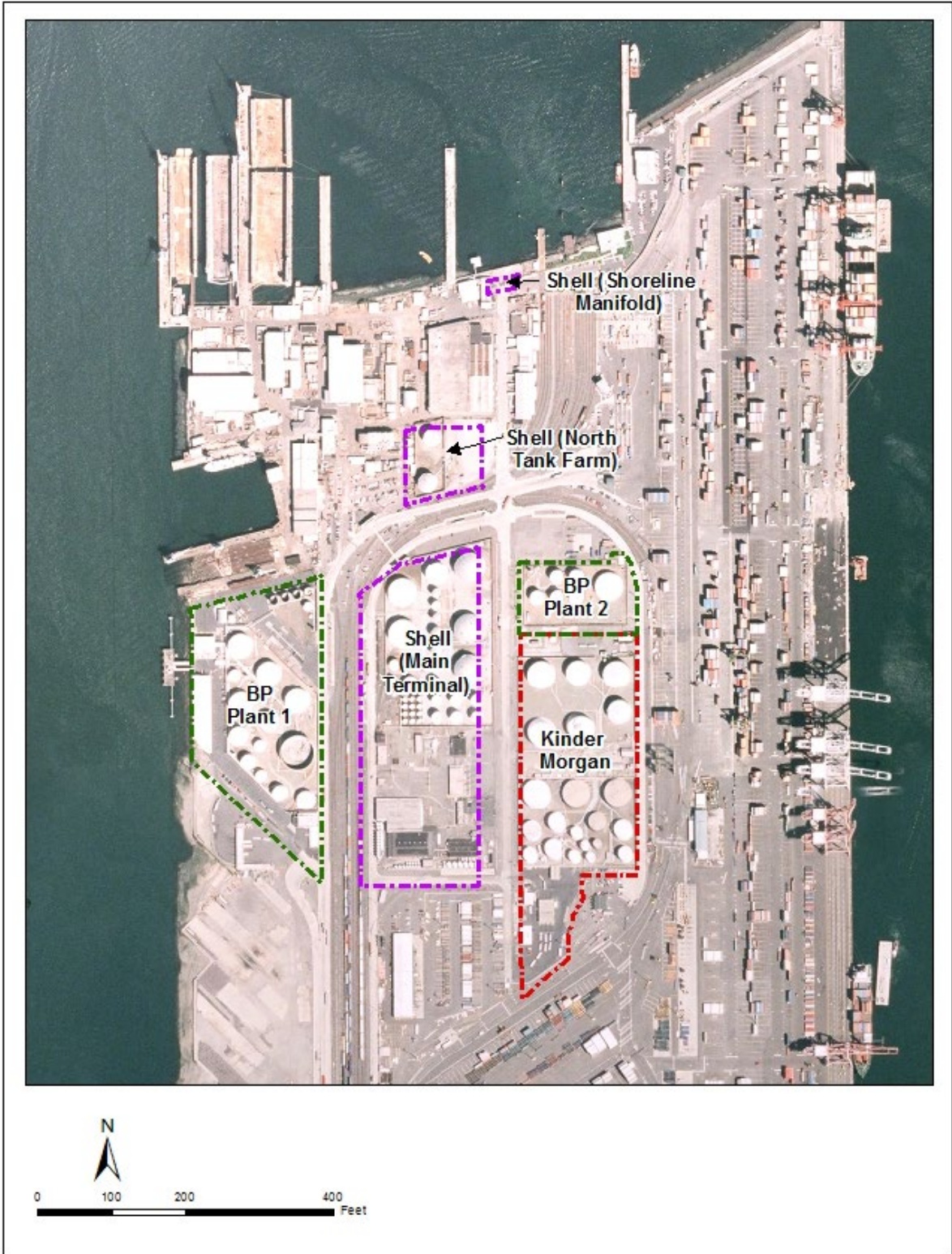
Figure 3. TF-OU2 - Tank Farm Facilities
