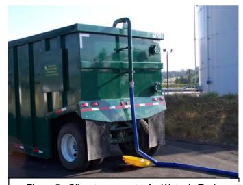
Figure 5 - Oil-water separator for Water in Tank
