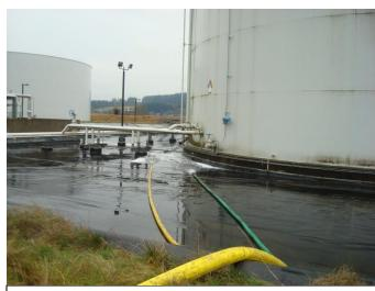
Figure 6 – Water from Stormwater Pond Pumped to Storage Tank Containment Structure
