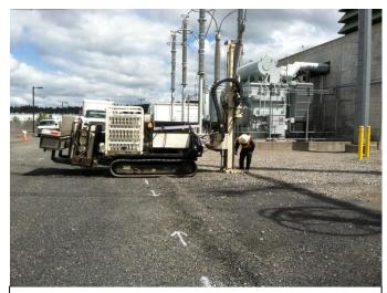
Figure 4 – Geoprobe drilling for Well GW-4 near Transformer
