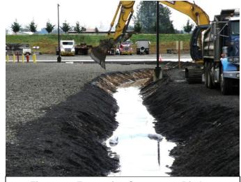
Figure 3 – Excavating Stormwater Ditches
