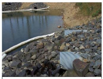
Figure 6 - Discharge of Tank Water to Stormwater Pond
