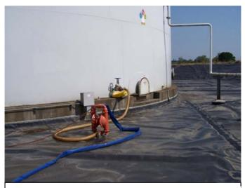
Figure 4 - Drain Connection for East Fuel Oil Tank
