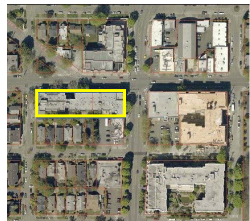
Aerial image of Stone Way Apartments.
