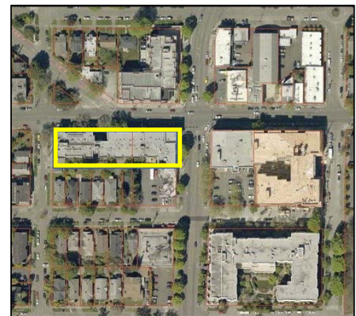
Sawirka hawada ee Stone Way Apartments.
