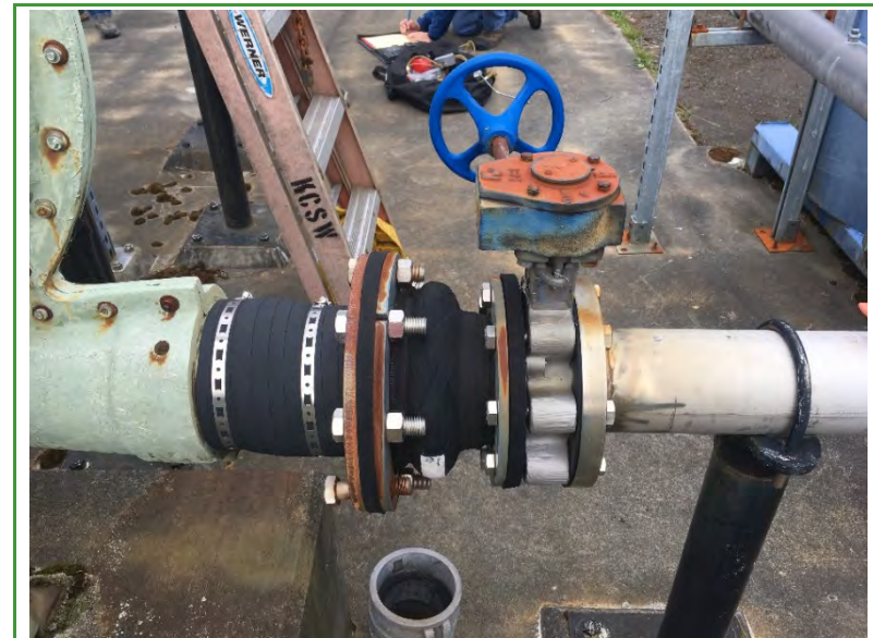
20. Discharge flex fitting
