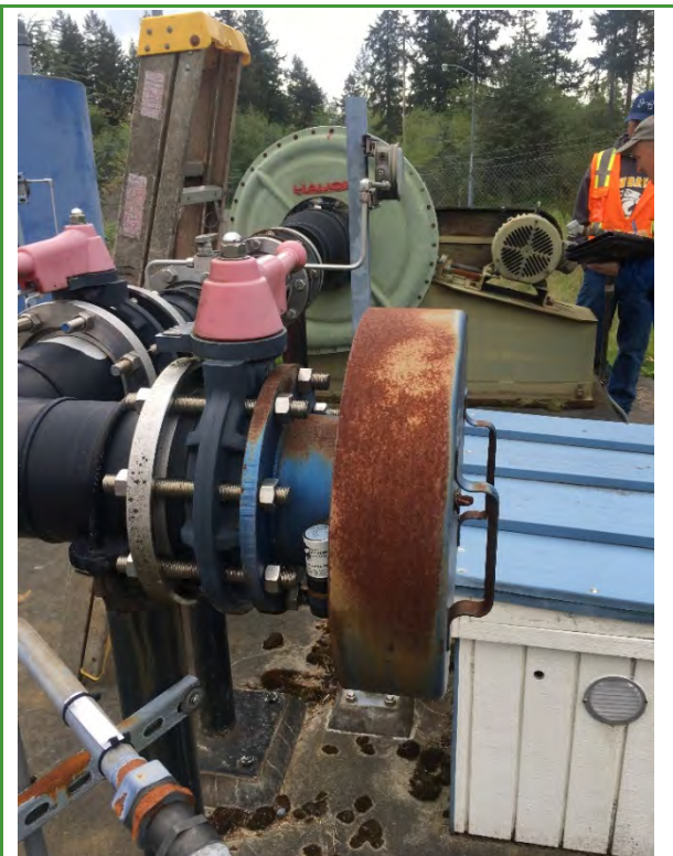
59. Diffuser valve. Fully closed
