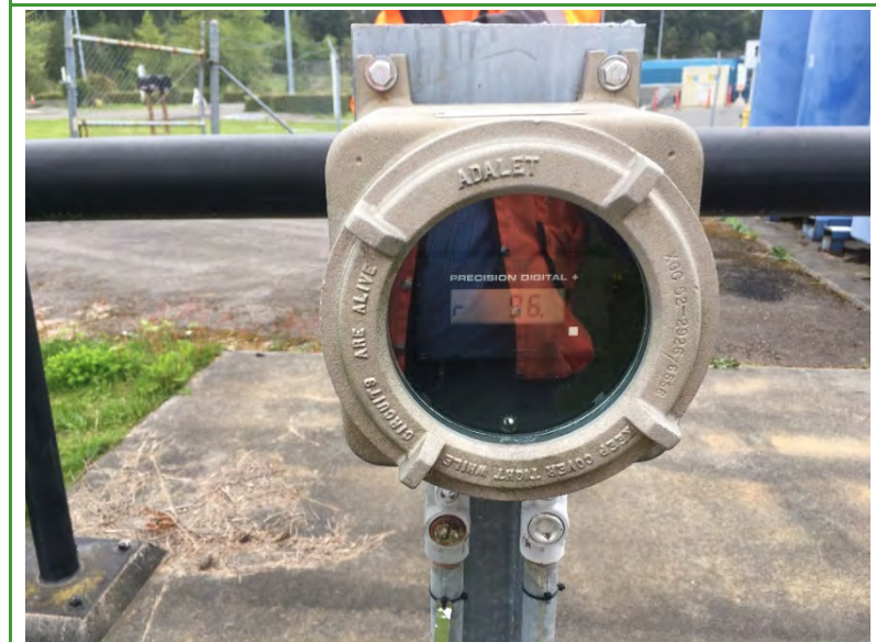
12. Flow readout, showing 96
