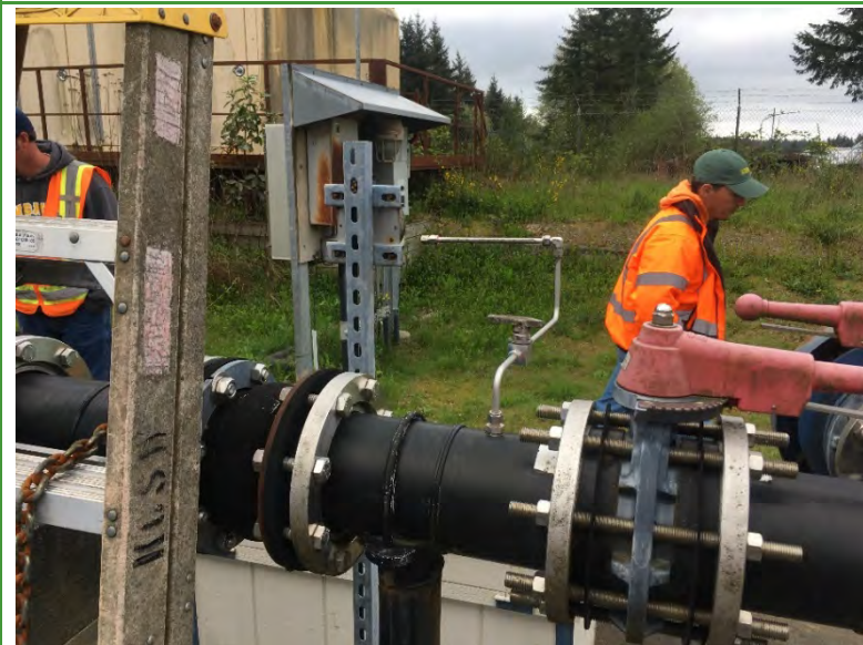
8. Flex fitting and valve
