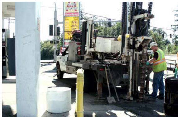
Photo #4: View of hollow stem auger drilling at Boring B-1, adjacent south of previous and current fuel underground storage tanks.
