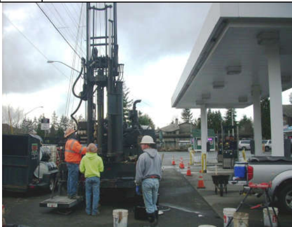
Photo #13: Setting-up drilling rig at location for monitoring well MW-2. Photo looking North
