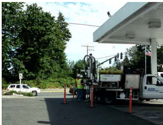
Photo #7: Direct push probe drilling at AEG Boring B-3, on the northeast side of the dispenser islands. View looking to the east.
