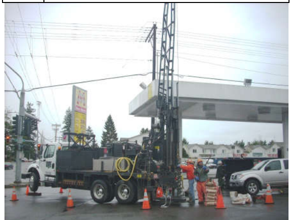
Photo #16: Installing groundwater monitoring well MW-3. Photo looking South
