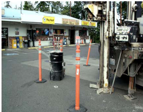
Photo #8: Direct push probe drilling at AEG Boring B-4 (note previous Envitech boring S-1 adjacent to drum). View looking to the northeast.
