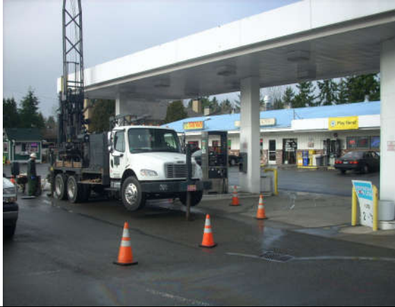
Photo #11: Installing groundwater monitoring well MW-1. Photo looking Northwest
