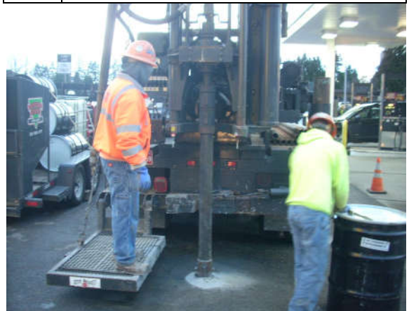
Photo #14: Drilling of borehole MW-2. Photo looking North
