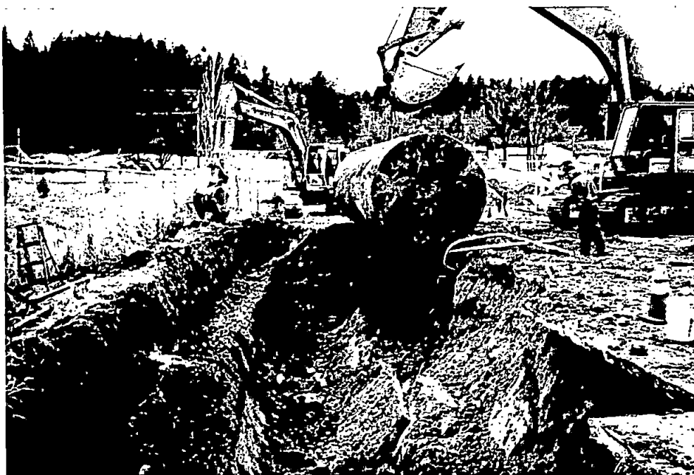
Tank T-1 (unleaded gasoline) during removal from ground.
