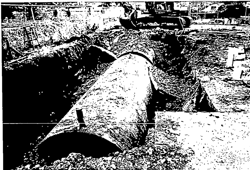
View looking west at UST's prior to removal from ground.
