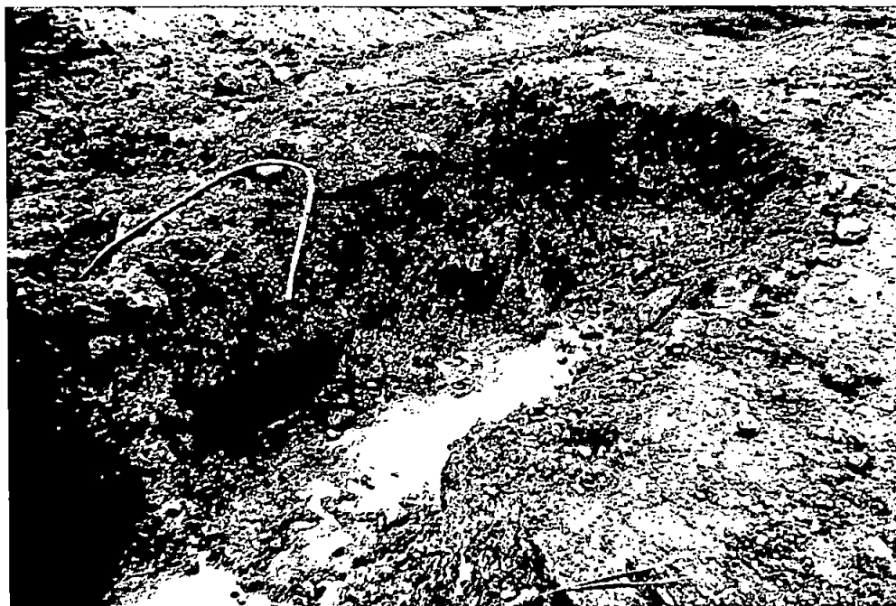
Pump-island area prior to over-excavation of contaminated soil. Note small amount of water which seeped from gravel layer directly below asphalt.
