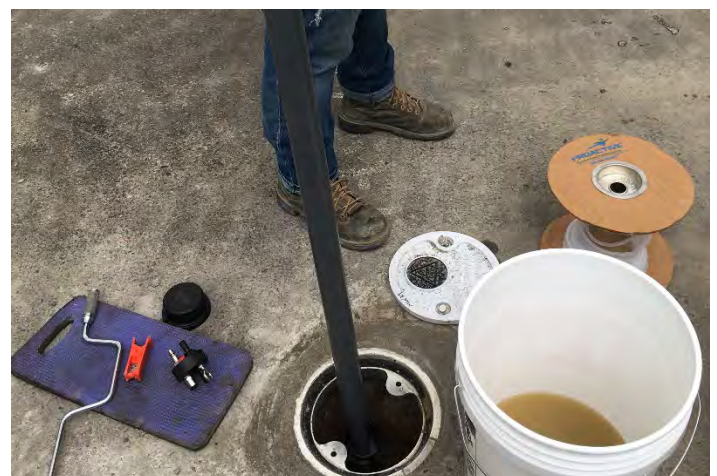
Photograph 12. Installing dedicated bladder pumps in supplemental monitoring wells; September 20, 2019.
