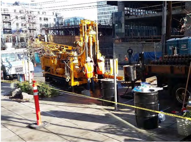
Photograph 1. Installing supplemental monitoring well MW27 in Boren Avenue North ROW; December 1, 2015.
