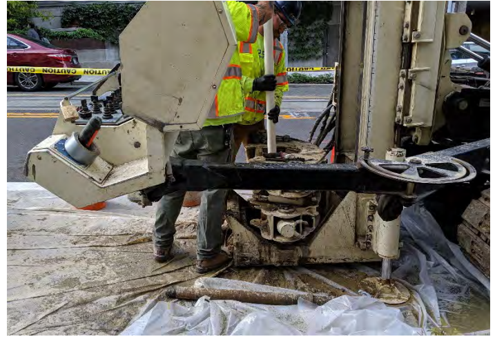
Photograph 8. Installing supplemental monitoring well MW31 in Boren Avenue North ROW; September 11, 2019.
