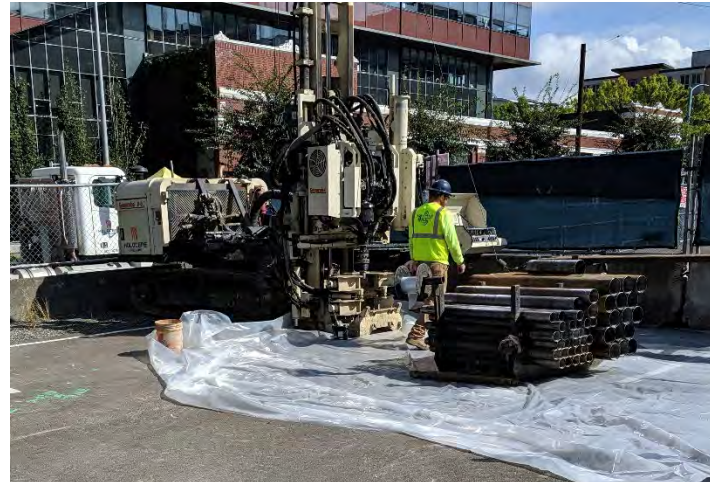
Photograph 10. Installing supplemental monitoring well MW29 on south-adjacent property; September 16, 2019.
