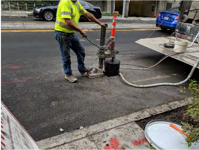
Photograph 7. Installing supplemental monitoring well MW32 in Harrison Street ROW; September 9, 2019.
