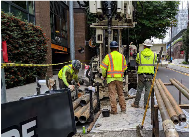
Photograph 9. Installing supplemental monitoring well MW33 in Harrison Street ROW; September 13, 2019.
