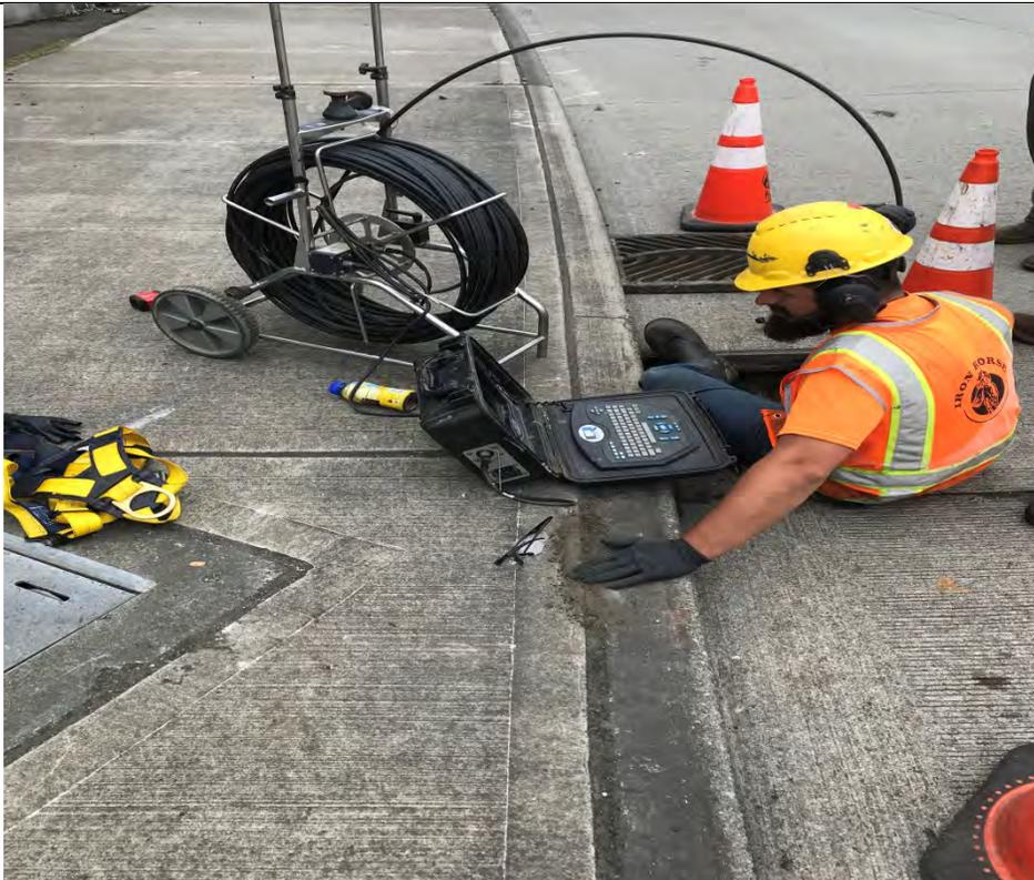
**Description:** CCTV of t-liners installed in laterals
