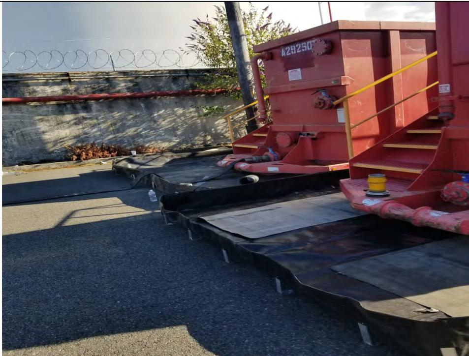
**Description:** 18,000 gallon settling tanks staged for bypass system
