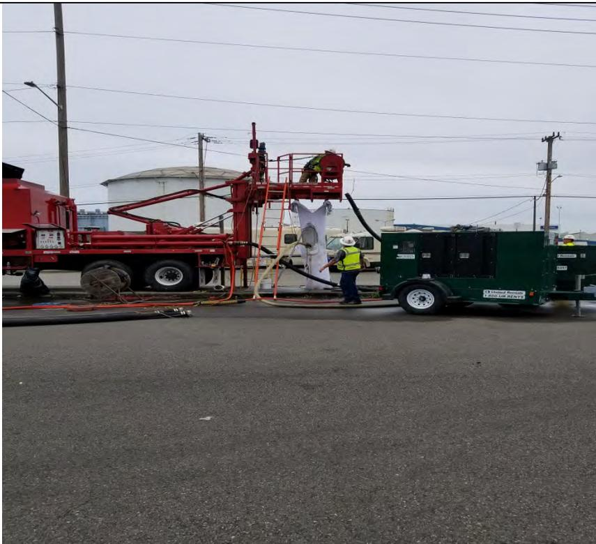
**Description:** Setup of CIPP during curing process
