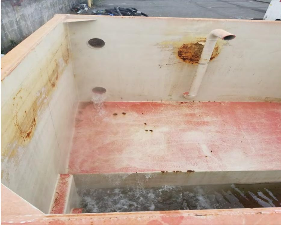
**Description:** Heated cure water pumped from CIPP liner to roll-off tank to cool for discharge
