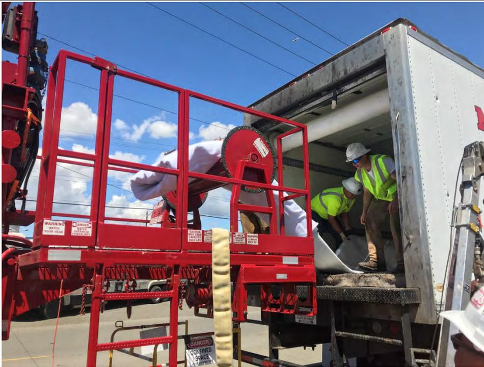
**Description:** CIPP liner removed from cold storage truck during insertion at D050-016.
