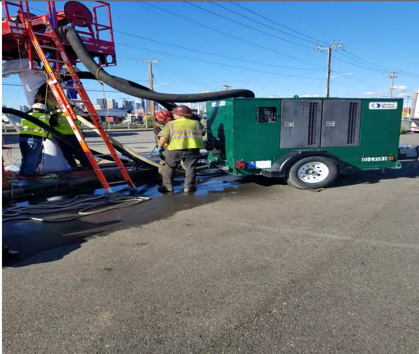
**Description:** Pump circulating water through CIPP liner
