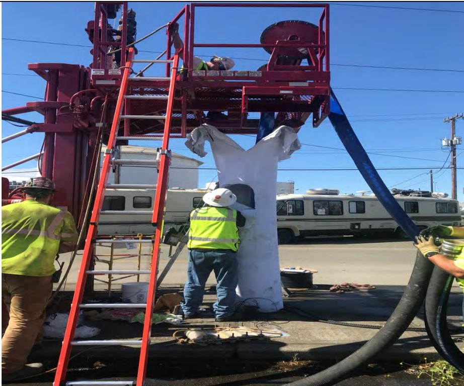
**Description:** Access point cut into liner for pump hoses to circulate heated water
