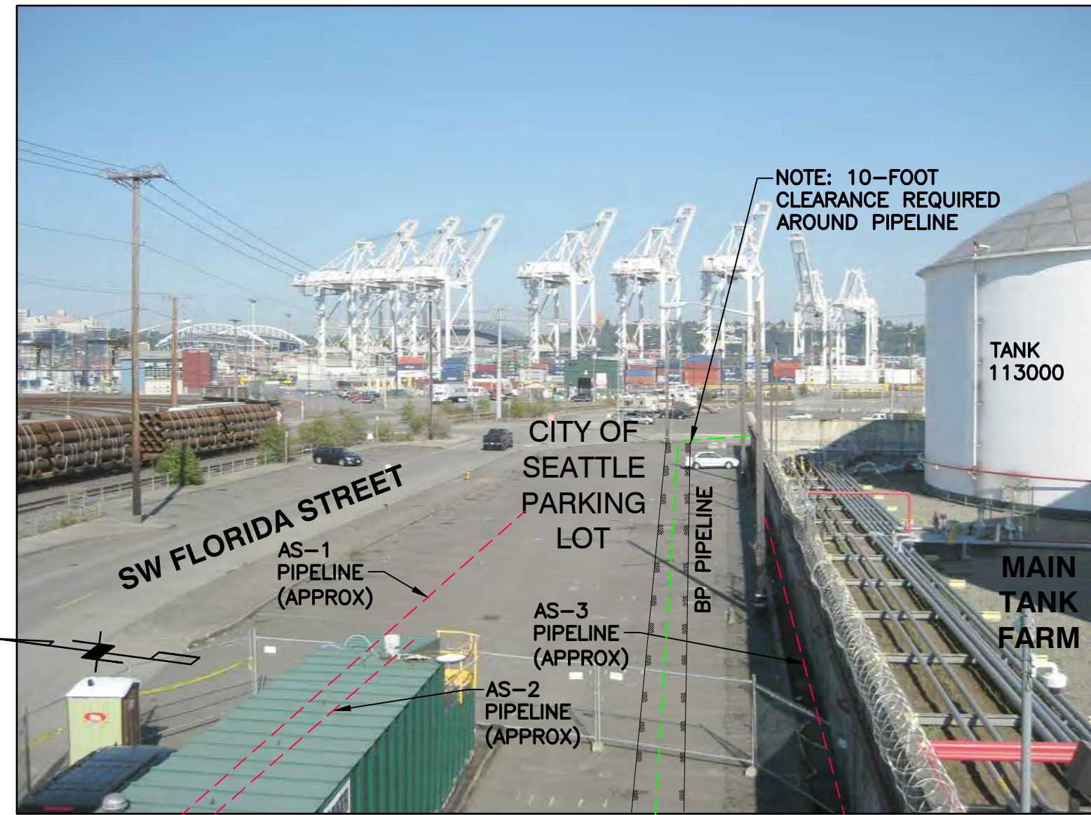
PIPING IN CITY OF SEATTLE PARKING LOT
