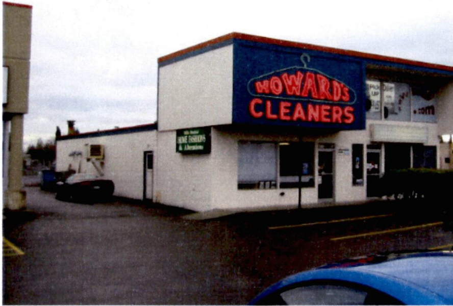
Photograph Five and Six: Based on the surface topography at the Market Square and the Howard's Cleaners' property, surface water from Howard's Cleaners flows to Market Square where the storm drain is located.
