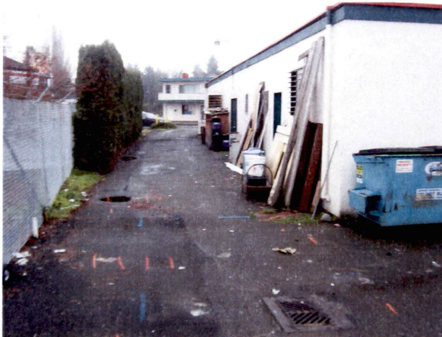
Photograph Four: A storm drain catch basin is located near the rear of Howard's Cleaners. Storm water entering the catch basin travels in subsurface piping along the alley which separates Howard's Cleaners and the Market Square property.
