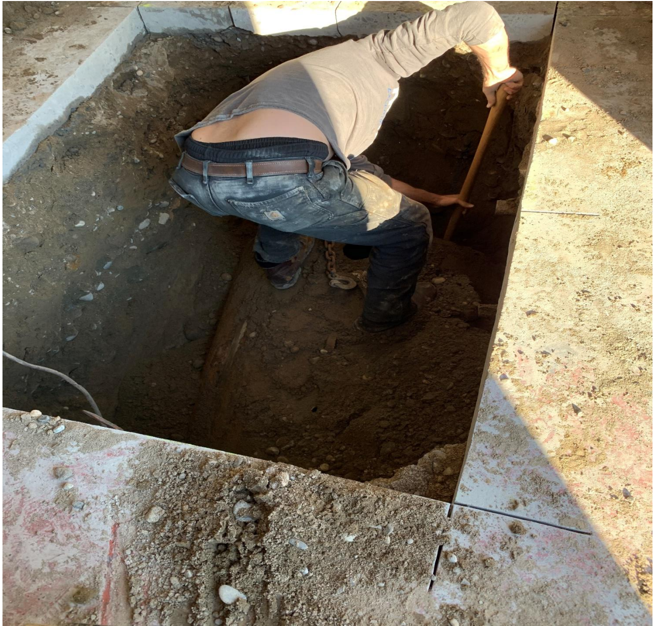
Photograph 5 – Clarke Construction employee hand digging soil from north end of HOT on November 11, 2020 (facing north).
