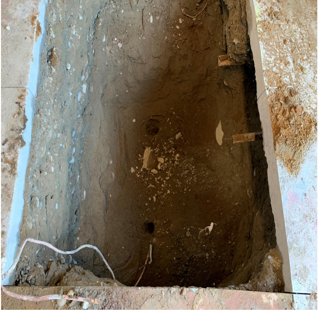
Photograph 9 – Bottom of HOT excavation with hand auger boring holes at base of former tank on November 11, 2020 (standing on south end of tank pit facing north).
