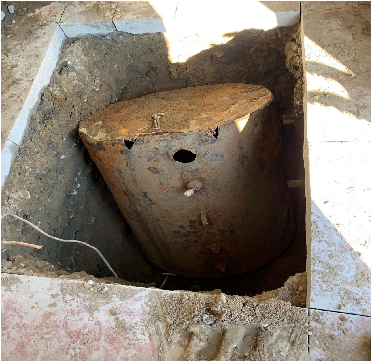
Photograph 6 – 320-gallon HOT ready for removal from excavation on November 11, 2020 (facing north).
