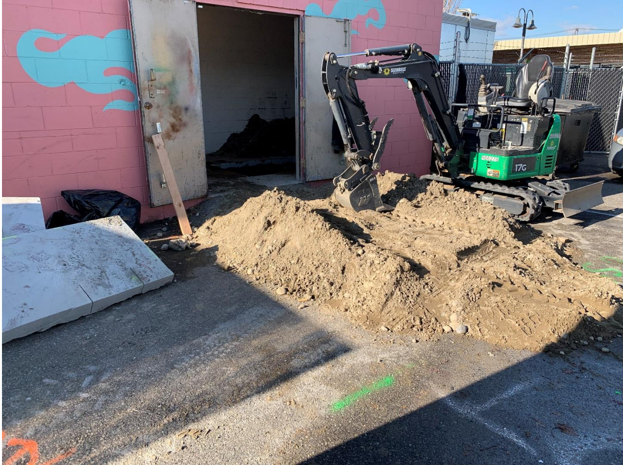
Photograph 11 – Mini-backhoe use to excavate soil and HOT on November 10 and 11, 2020 (facing NW).
