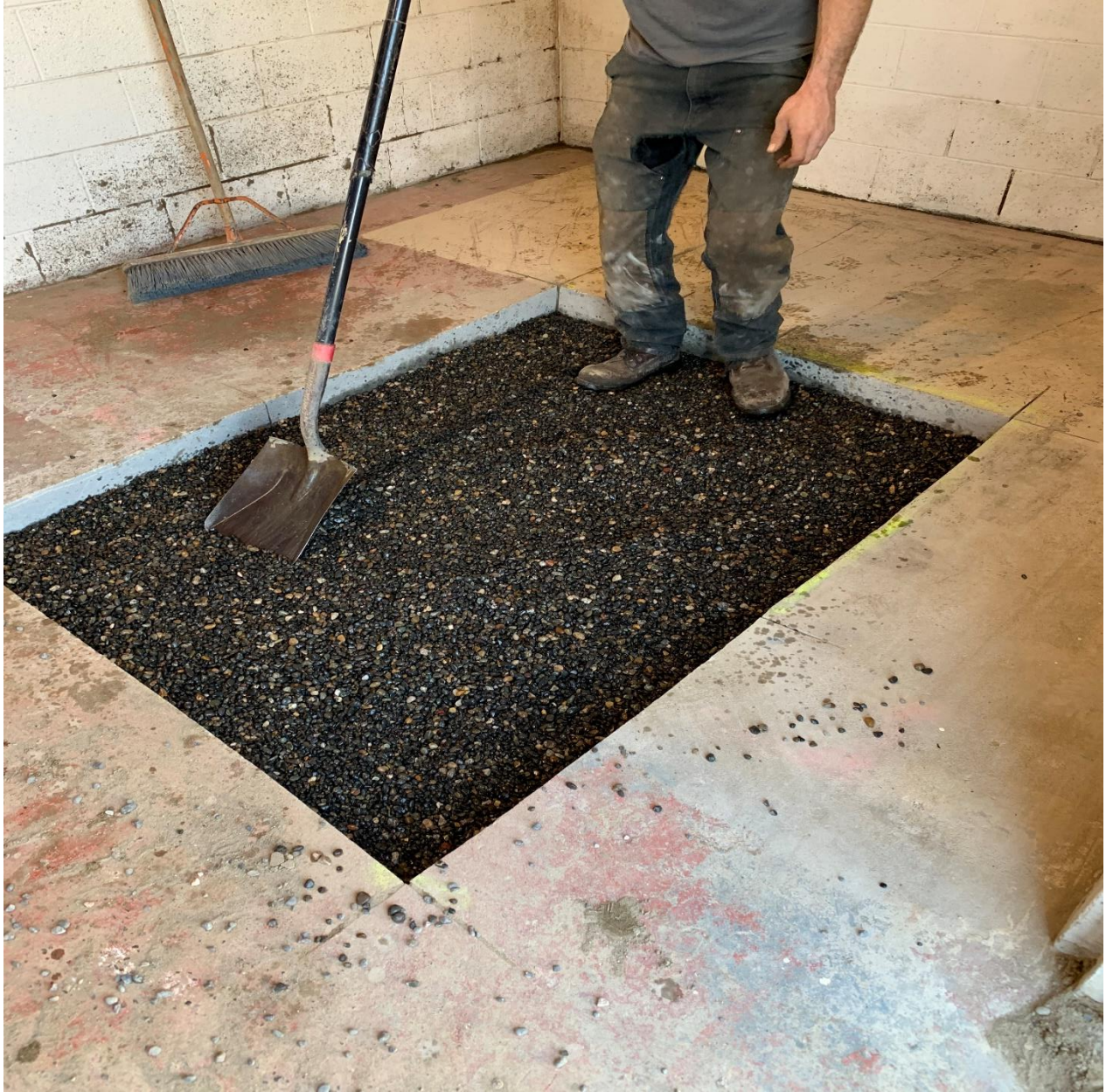
Photograph 12 – Pea gravel backfill on November 11, 2020 (facing NW).
