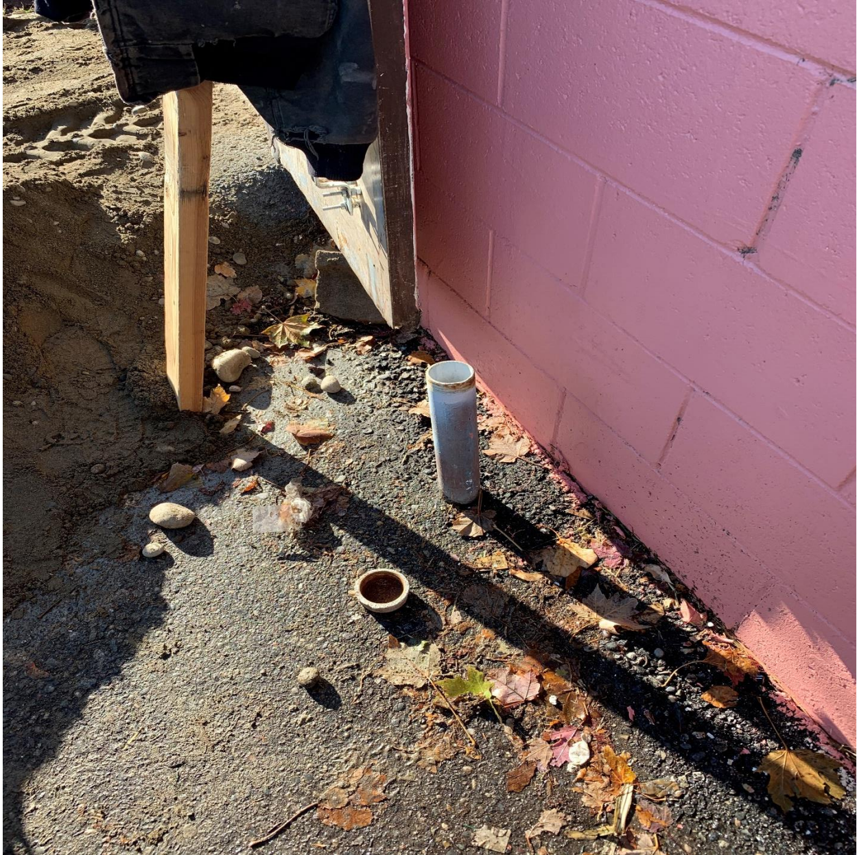
Photograph 10 – Fill port located on outside of the building did not have the cap on top of it when we arrived onsite on November 10, 2020 (facing SW).
