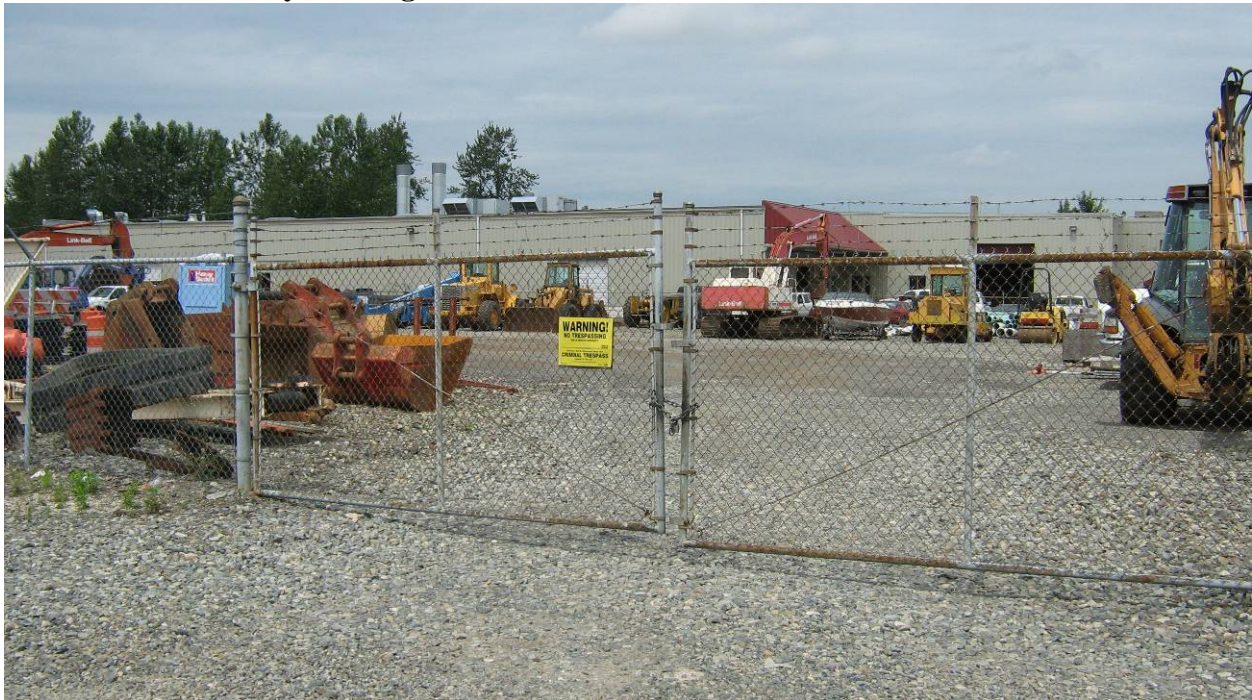
Photo 4: Site Security Fencing Around Lot 2 – from the south
