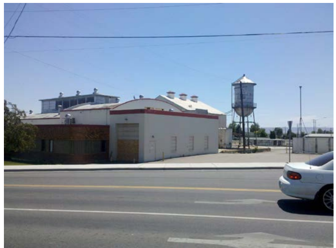
View of the Site from the North
