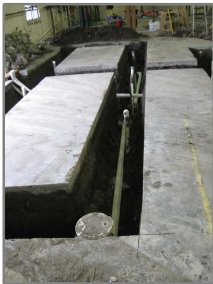
Frame 2-1: Trenches made in warehouse to install VES and water processing lines. (12/16/2009)
