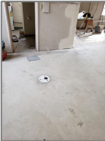
Frame 19-1: ( Looking ESE )Each grade level access point has either a monument or a custom fit steel plate covering. In total there are (27) 10" and (8) 8" monuments. (2/24/2020)
