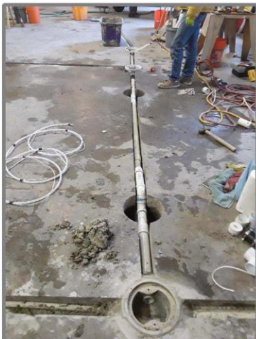
Frame 6-3: A total of eight 2" production wells were installed. Six in the warehouse and two outside. Over the next two years, seven more production wells would be installed. Four inside and three outside. (11/12/2017)
