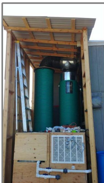
Frame 9-3: ( Looking W )South processing shed with Air Strippers 2 and 3 completed. (5/6/2018)
