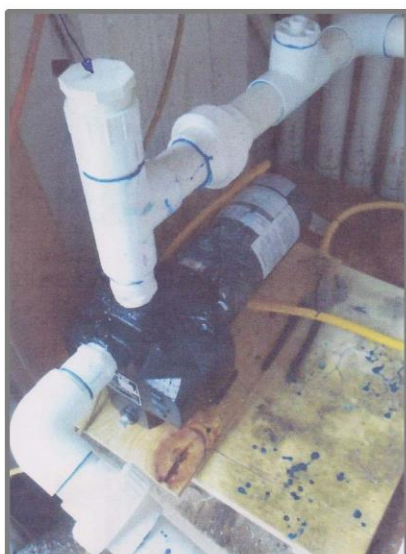
Frame 3-3: In January 2013, we began a series of hydrogen peroxide treatments. An 8% H 2 O 2 solution was further diluted with water to 0.16% and injected via a jet pump. (6/2011)
