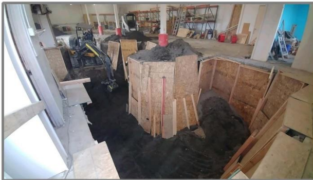
Frame 13-2: Shoring was installed along the side walls of the excavations to ensure the stability of the workspace. (8/29/2019)
