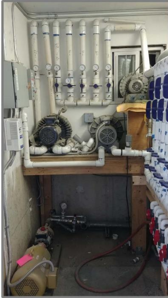
Frame 8-1: (Inside Central Processing Shed )Pumps for VES. The larger black pump on the left blows clean air into the ground through the VES plumbing. The gray pump to its right pulls vacuum from the wells and sparge lines into a carbon filtration system on the other side of the wall to the south. On the wall to the left( east wall ) are controllers for the two pumps. (8/22/2018)
