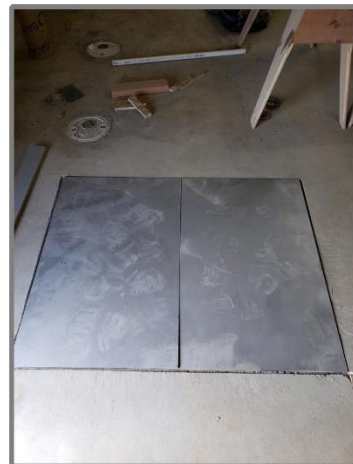
Frame 19-3: ( Looking S )This steel plate covering, located immediately southwest of the garage door in the warehouse( enclosure shown in Frame 18-2 ), is the largest of eight custom fit enclosures. (3/11/2020)
