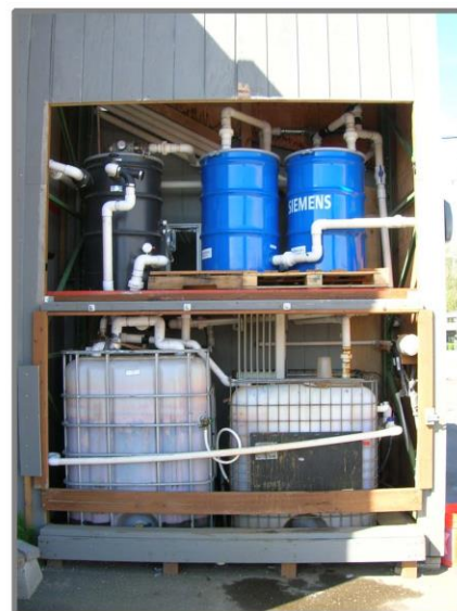
Frame 2-4: Processing Shed. Carbon filters in the steel drums and related plumbing are for the VES system. The two tank shown at the bottom are sediment tanks for processing the water from the paristaltic pumps. (1/2010)
