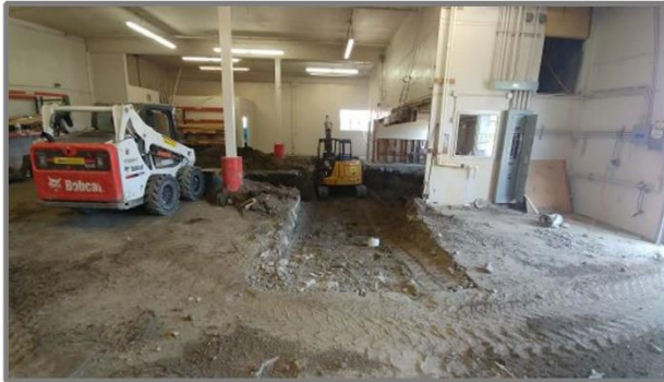
Frame 13-1: ( Looking N ) After a thorough survey to fully map out the full extent of the contaminated soil, it was determined that the best course of action was to excavate as much of the contaminated soil as possible. Within the warehouse, this was accomplished in four separate phases. Phase 1 being a roughly 20' x 12' x 10' deep area at the north end of the warehouse. Phase 2 a somewhat larger ~20' x 20' x 10' deep area just to the south and connected to Phase 1. Phase 3 being a smaller ~10' x 10' x 10' deep area to the west of the warehouse garage door. Phase 4 a ~18' x 25' x 10' deep area mostly overlapping to 2017 excavation. (8/3/2019)
