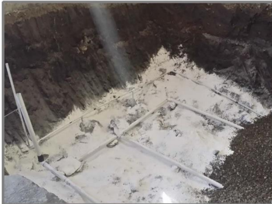
Frame 5-1: Application of lime in excavation prior to being filled with drain rock. (8/21/2107)
