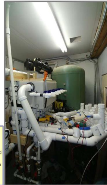
Frame 11-2: The last step prior to treated water being returned to the ground was for it enter a small holding tank where it could be mixed with a controlled amount of hydrogen peroxide and then pass through a UV bath (black apparatus shown in the photo ). (12/1/2018)
