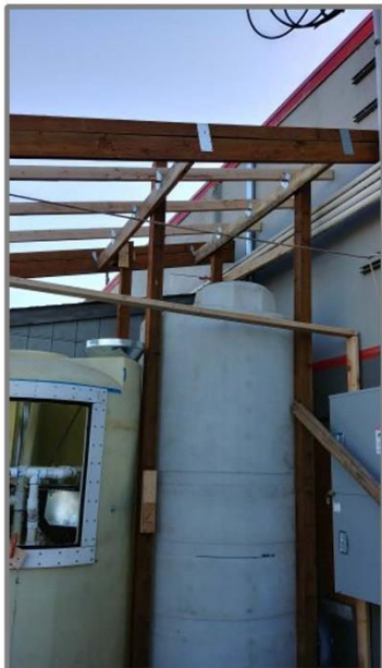
Frame 7-1: Construction of the new sediment tank( right ) and Air Stripper 1( left ). (3/31/2018)
