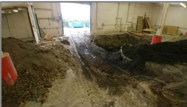
Frame 15-4: ( Looking SE ) Clean soil was stockpiled inside the warehouse( shown on the left side of the image ). Contaminated soil was mostly placed directly into boxes to be hauled away by Republic Services Inc. Small temporary stockpiles were made( see the right side of the image ) when space in the boxes ran out. (9/20/2019)
