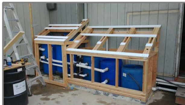
Frame 7-4: From left to right; two drums used to cycle treatment water through Air Strippers 2 & 3 to provide multiple pass throughs and overflow protection, two drums containing organoclay filter material and a return line drum that fed cleaned water back into the ground. (6/8/2018)
