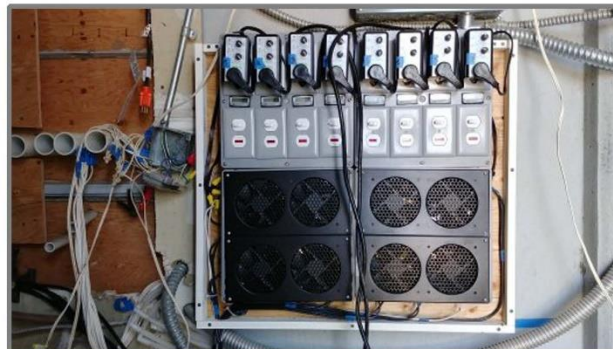
Frame 7-3: Controller panel for the production well inline pumps. Each pump was capable of pumping ~2gpm. However, to avoid overloading the treatment system and wearing out the pumps, each pump was set to run on a time cycle appropriate for each well. (5/24/2018)
