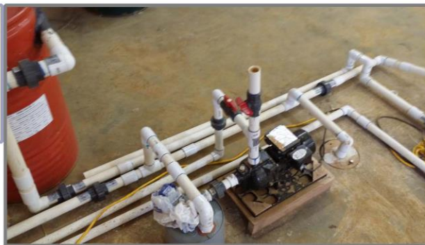
Frame 11-4: To handle the increased amount of water being pumped by the jet pumps, two additional 250 gallon sediment tanks along with 2 drums to transfer water to the rest of the system were added. (3/24/2019)
