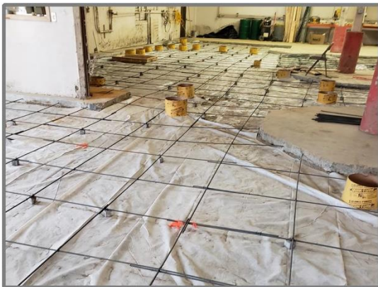
Frame 18-3: Before closing the excavation, a vapor barrier and rebar were installed. (12/17/2019)
