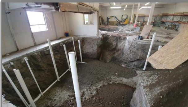
Frame 14-4: ( Looking S )As work was completed inside each excavation phase, the shoring was removed and clean soil and drain rock was used to fill in the excavated area. Phases 1 and 2 were excavated together and filled sequentially as the work inside was completed. Work then moved onto phase 4 at the south end and then to phase 3 west of the garage door. (9/4/2019)
