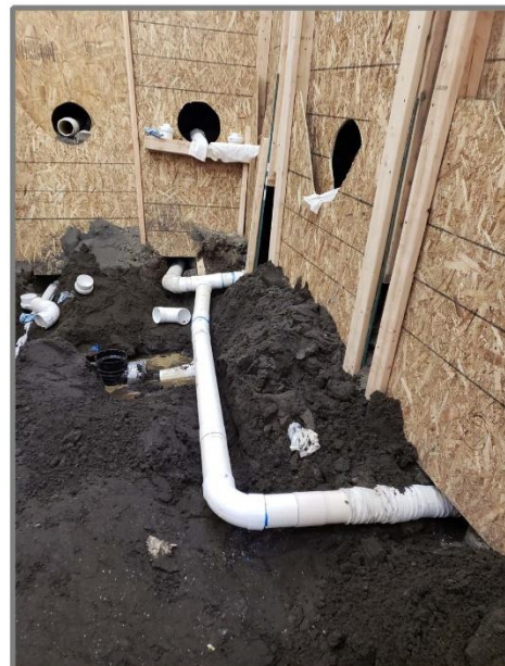
Frame 13-4: The gallery of horizontal lines at ~10'-11' depth were connected to a central collector pipe. There is one collector pipe in each of the four phases. (9/20/2019)
