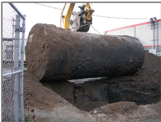
Frame 1-1: 7,500 gallon Underground storage tank(UST) removal. (3/3/2009)
