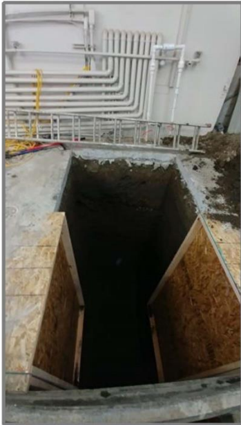
Frame 12-1: ( Looking E )5' x 10' x 10' deep exploratory excavation in the SE corner of the warehouse. Testing showed that this area was at the southernmost extent of the zone of contamination. (7/4/2019)
