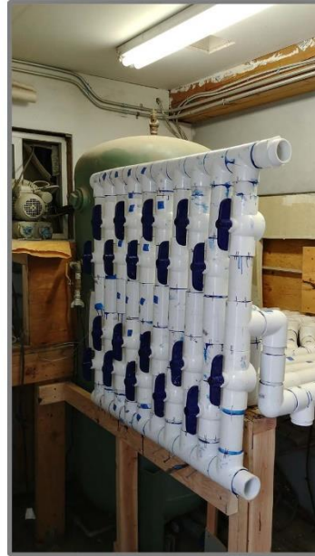
Frame 8-2: ( Inside Central Processing Shed )Upgrade of the VES system. The valves shown control whether a well is being blown into with clean air via the blower or VOCs being pulled through the vacuum pump to a carbon filtration system. (8/22/2018)
