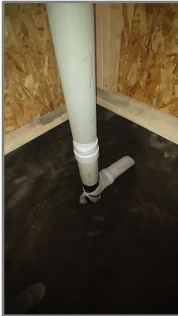
Frame 12-2: ( Looking NE )At ~10ft. below grade, this 2" perforated lines was installed horizontally to the east under warehouse wall. It was then plumbed to allow passive venting, VES extraction, and in-situ treatment injection. (8/12/2019)
