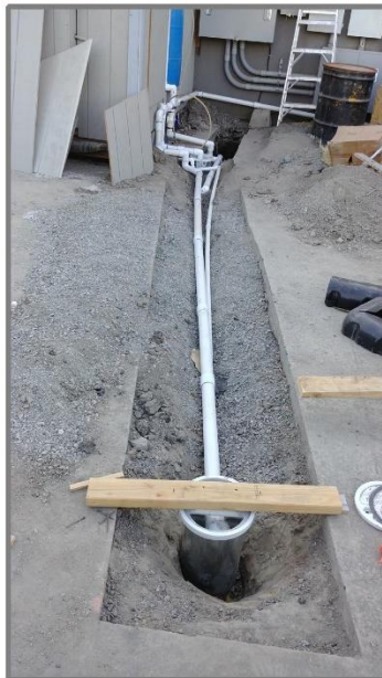
Frame 10-3: ( Looking SW ) A trench was dug in an area just south of the location of the UST southwest to the north processing shed. VES lines and two processing wells were installed at that time. (9/4/2018)
