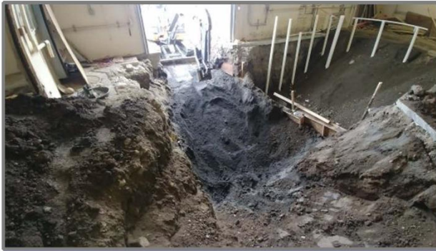
Frame 16-1: ( Looking ESE )Phase 3 of the excavation was completed last as it's location necessitated a pathway for equipment to drive through while completing the other three phases. (9/27/2019)
