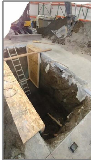
Frame 12-3: ( Looking SW )5' x 10' x 10' deep exploratory excavation ~30' north of the warehouse's south wall and ~20' east of the warehouse's west wall. Testing showed that only the northeast corner of the excavation contained contaminated soil. (7/2/2019)
