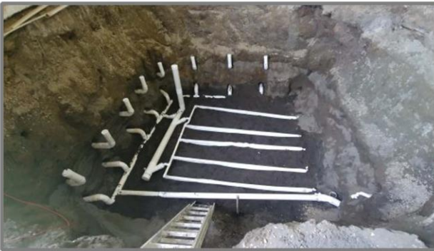
Frame 15-3: ( Looking S ) The horizontal borings for the irrigation gallery were mostly aimed to access the contaminated soil that we weren't able to directly excavated. This was mostly under walls, support columns and other structural elements of the warehouse. (9/23/2019)
