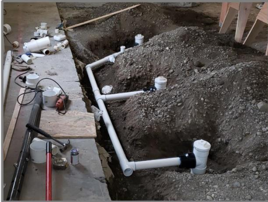
Frame 18-1: ( Looking SWS )At grade plumbing for the irrigation/VES gallery. Each of the horizontal lines at ~8' below grade has it's own access point at grade and the collector lines for the ~10'-11' below grade gallery from each phase have a 6" access point at grade as well. (11/9/2019)
