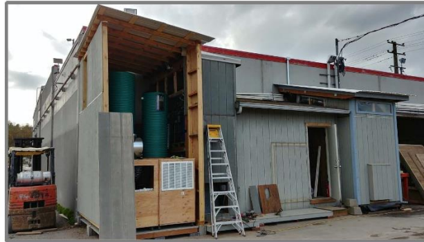
Frame 7-2: Construction of the upgraded processing system included a 750-gallon sediment tank and Air Stripper 1 in the shed on the right of the image and Air Strippers 2 and 3 in the shed on the left. (4/21/2018)
