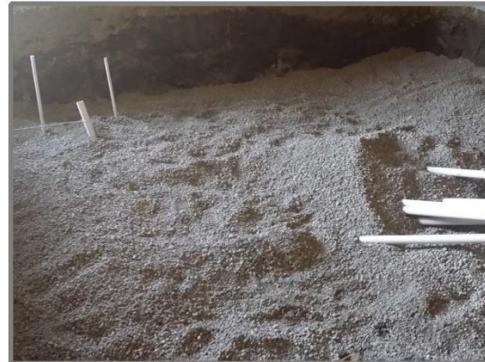
Frame 5-2: (Looking ESE )Excavation partially filled with drain rock. (8/21/2017)
