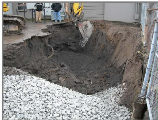
Frame 1-2: Soil was excavated to ~10ft. below grade around the location of the UST and along the feed line from the UST to the warehouse. (3/5/2009)
