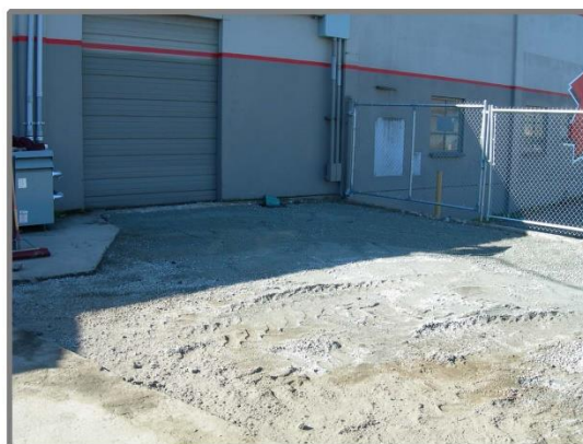
Frame 1-4: Excavation was filled with drain rock and closed. (3/6/2009)
