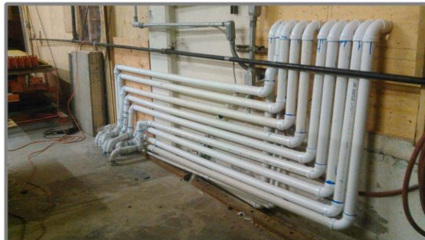
Frame 6-4: Water treatment and new VES lines from the six warehouse production as well as the two outdoor lines converge at the processing sheds on the other side of this wall. (11/28/2017)
