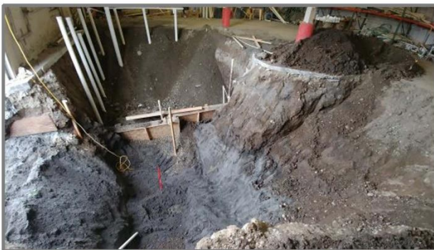
Frame 16-2: ( Looking S )Due to logistical constraints, phase 3 wasn't able to be excavated as fully as the other phases. A depth of ~10'-11' was still reached, but the footprint was smaller. (9/27/2019)
