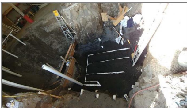
16-4: ( Looking WSW )As with the other phases, phase 3's irrigation gallery consisted of: 4" pull/vent lines bored 8'-10' out horizontally from the perimeter of the excavation at ~10'-11' below grade, a gallery of sparge lines located ~10' below grade and 4" vent/treatment lines at ~8' below grade. (10/2/2019)
