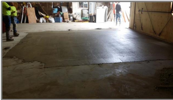
Frame 6-1: Excavation closed with vapor barrier and reinforced concrete. (8/24/2017)
