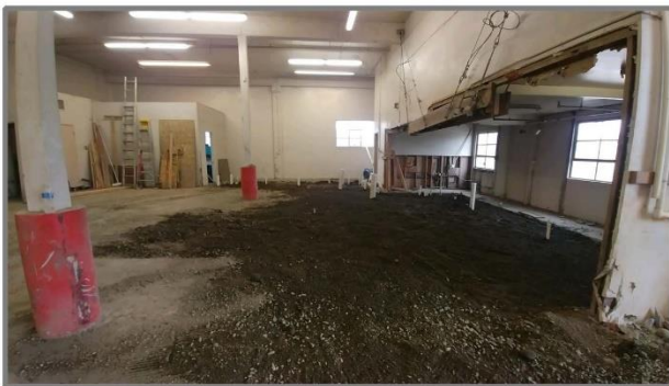
Frame 17-2: ( Looking South )Drain rock was used to fill the bottom several feet with the other material( mostly pit run ) overlain on top to grade. (9/20/2019)
