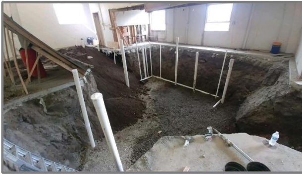
Frame 17-1: ( Looking NE )The excavation were filled in with a mix of clean soil, 3/8 minus drain rock, pit run and gravel borrow. (9/20/2019)
