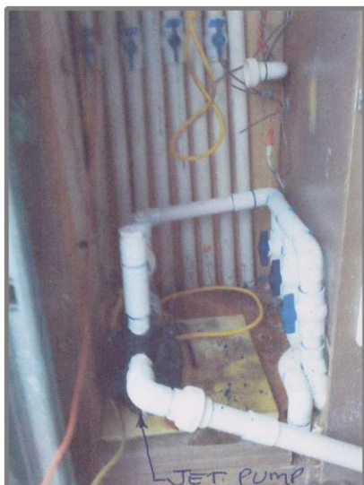
Frame 3-1: Inside the processing cabinet. The jet pump was used to push RegenOx ORC or alternatively hydrogen peroxide treatment to a drain field under the warehouse. (6/2011)
