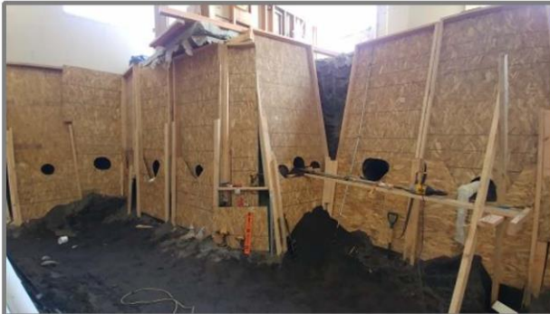
Frame 14-1: ( Looking NE )A 1 1/2" drill was used to create 6" diameter x 10' long borings for the 1 1/2" and 4" gallery of lines going under the walls of the warehouse. (8/24/2019)
