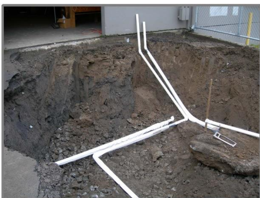
Frame 1-3: A vacuum extraction system(VES) was installed to pull vapor from the remaining contaminated soil surrounding the excavation. (3/5/2009)
