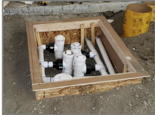
Frame 18-2: ( Looking ESE )Some grade-level access points for the irrigation/VES gallery were too tightly clustered together for each to have their own monument. In situations like that shown above, a box form was built with the intention of an enclosure with a custom fitted steel plate covering to be made for each one. (11/28/2019)
