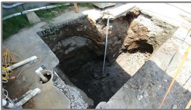
Frame 12-4: ( Looking NW )This 10' deep excavation was in an area known to still be contaminated. Located just north of the the north processing shed, the main purpose of this excavation was to remove what was thought to be some of the most contaminated remaining soil left and to install a gallery of horizontal treatment lines to the east under the warehouse wall and to the south under the processing sheds. (7/2/2019)
