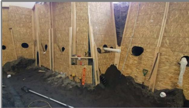
Frame 14-2: ( Looking NE )Between the four phases, the gallery of horizontal lines totals 62: (8) 1 1/2" lines at 8' below grade, (30) 4" lines at 8' below grade and (24) 4" lines at ~10'-11' below grade. Additionally, there is (1) 4" line at ~10'-11' below grade in the south exploratory trench and (1) 1 1/2" and (2) 4" lines at ~11' below grade, (1) 1 1/2" and (1) 4" line at 8' below grade and (1) 1 1/2" line at 6' below grade in the outdoor trench north of the north processing shed. (8/24/2019)
