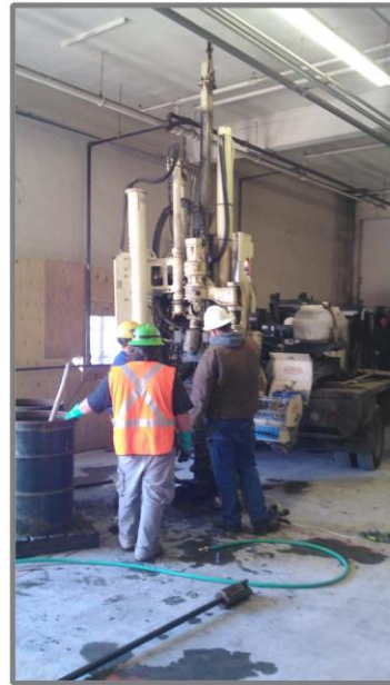
Frame 6-2: Borings for new well installation. Installation performed by ESN Northwest Inc. (11/6/2017)
