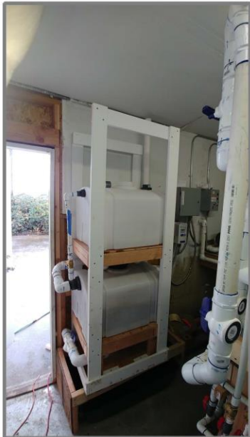
Frame 11-3: Replaced several inline pumps with jet pumps to increase the processing throughput by ~100%. (5/20/2019)
