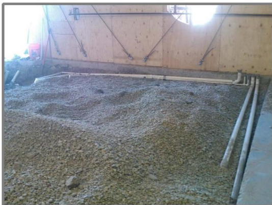
Frame 5-3: ( Looking ENE )Excavation filled to grade with grade-level VES plumbing shown. (8/22/2017)
