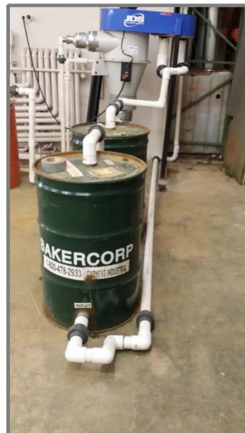
Frame 8-4: ( Looking E ) Additional vacuum pumps and carbon filters( black steel drums ) added to the VES system. (5/20/2019)
