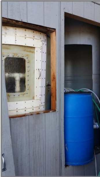
Frame 10-1: ( Looking SW ) North processing shed completed with blue inflow drum collecting water from wells. The water then feeds into a 7,500 gallon sediment tank( shown behind the inflow drum ) before feeding into Air Stripper 1( shown on left ). (5/11/2018)
