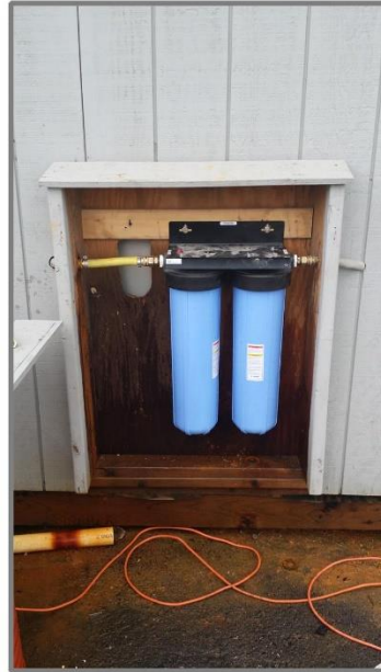
Frame 10-2: ( Looking W ) Water from the sediment tank is sent through these water filters before entering Air Stripper 1. (2/19/2019)
