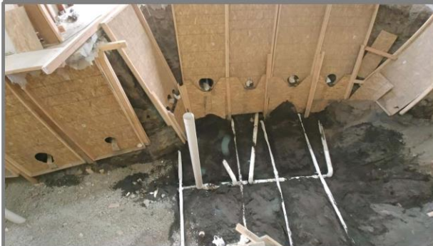
Frame 14-3: ( Looking E )In addition to the horizontal lines in each phase, a network of 1 1/2" sparge lines sitting at bottom of the excavation ~10'-11' below grade and connected to the phase's collector line was installed. (8/31/2019)
