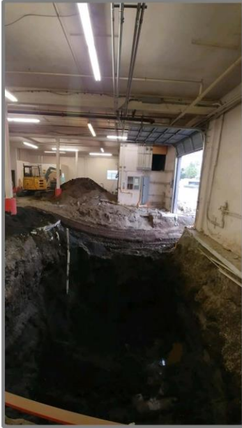
Frame 15-1: ( Looking S ) Due to access restrictions, Phase 4 was excavated, worked in and partially filled prior Phase 3 being excavated. (9/20/19)
