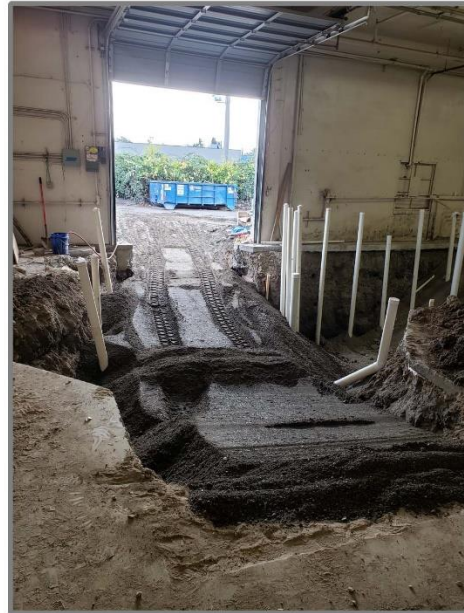
Frame 17-3: ( Looking ESE )The plumbing in phase 3 had to be routed in such a way to allow equipment to pass through the area during the excavatiop infill. (10/4/2019)
