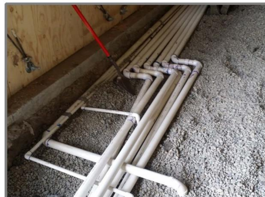
Frame 5-4: (Looking SE )Grade-level VES plumbing network leading south along the east wall of the warehouse to the processing shed. (8/23/2017)
