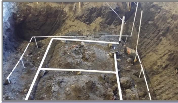
Frame 4-2: ( Looking North )Warehouse excavation at 7' below grade with VES plumbing installed. (8/20/2017)
