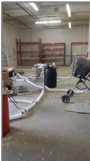
Frame 8-3: ( Looking S ) Additional VES lines added for each production well that was installed in the warehouse in 2017. (12/21/2018)
