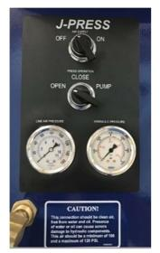
Figure 1. Filter press control panel for hydraulic cylinder operation.
