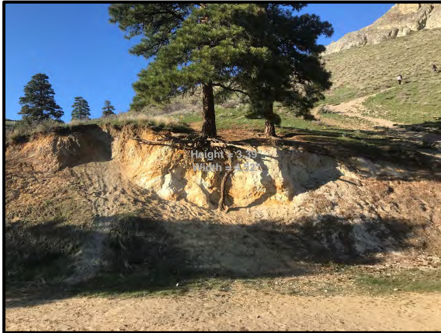
Photograph 31. Road cut at SR06 (view northeast)
