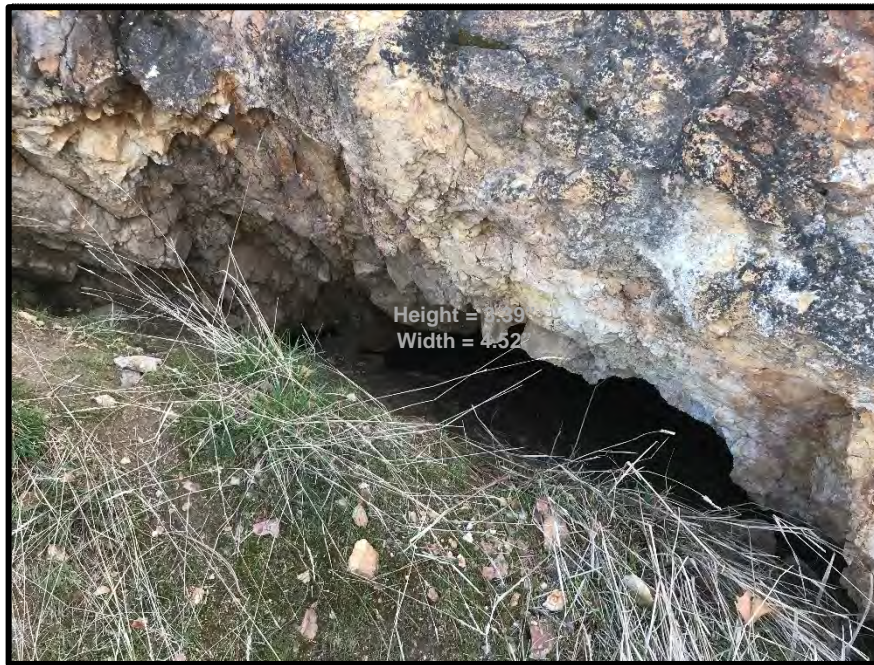
Photograph 40. Adit at SR08
