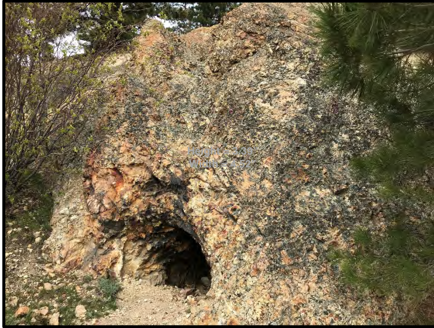
Photograph 39. View southwest at the portal area at SR07. The adit is situated on a mineralized outcrop. Total arsenic was identified with the XRF as high as 489 ppm just upslope from this location.
