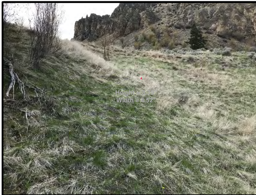
Photograph 16. Downslope berm vegetated with bunchgrass below waste rock pile at SR03 (looking west)
