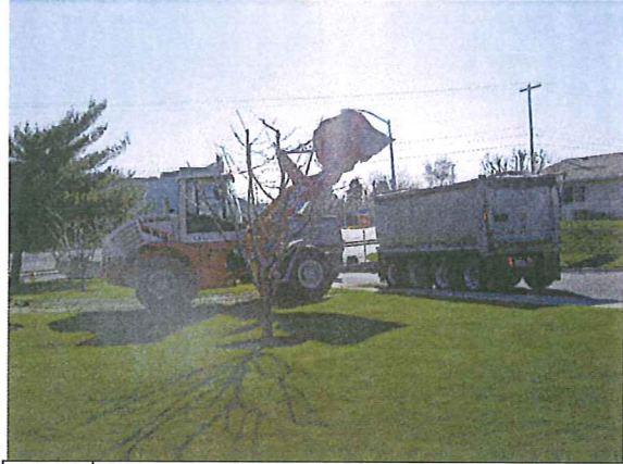
Photo #14: Excavated soil being loaded into truck and pup for transportation to waste facility. Truck is parked on Fairbanks Ave. which intersects 34 th Ave N.
