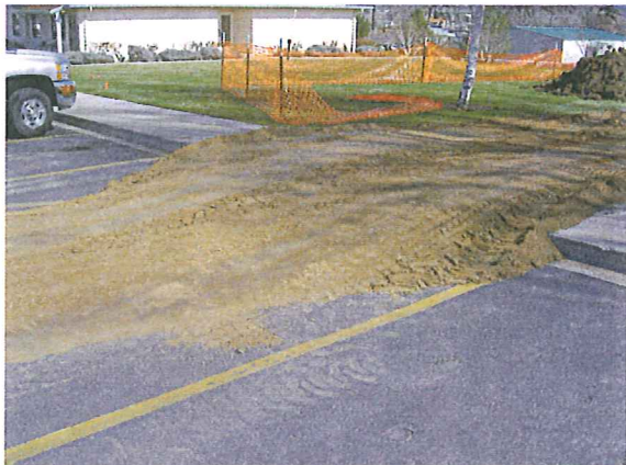
Photo #12: Entrance point to Zones 2 and 3. Ramp created to allow access of excavation equipment.
