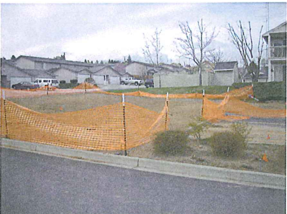
Photo #11: View of Zone 4, looking to the southwest, after clean imported soil has been brought in and raked into place.
