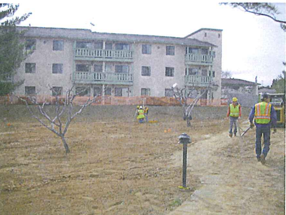
Photo #5: View of Zone 1, looking at the northwestern portion of the facility building, with the clean imported topsoil being raked into place.
