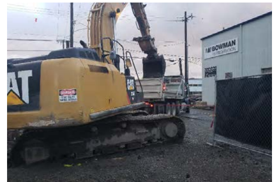
Removing contaminated soil from the site.
