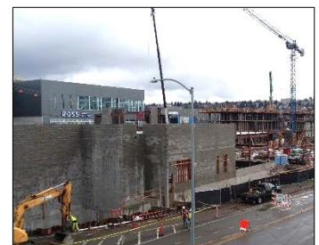
Development begins after cleanup was conducted.
