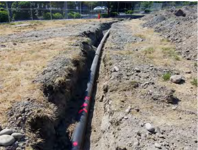
STA 2+20 LOOKING WEST
