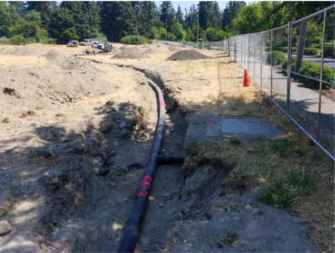
STA 1+50 LOOKING EAST
