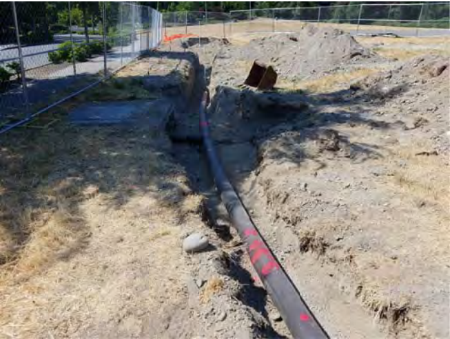
STA 1+65 LOOKING WEST
