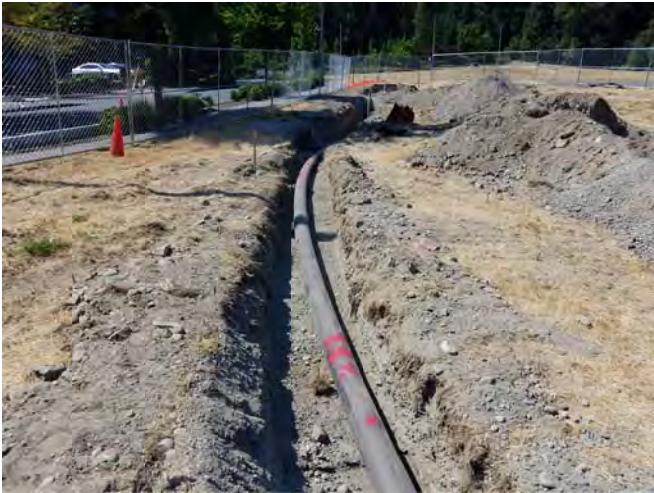
STA 1+78 LOOKING WEST
