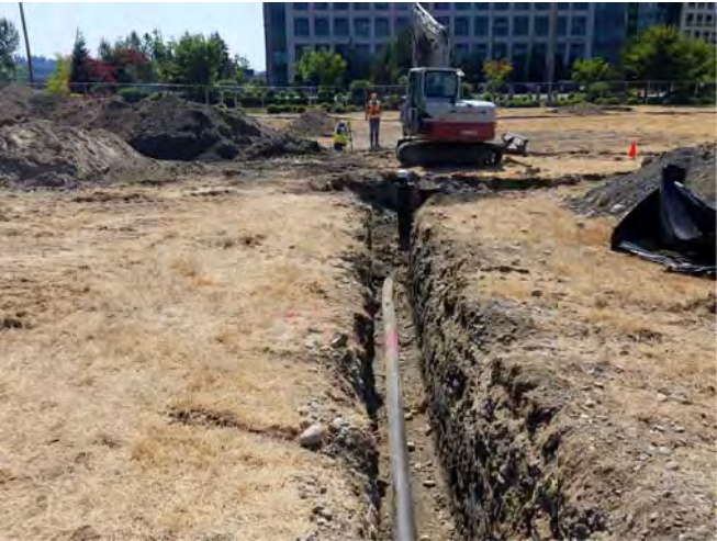
STA 4+15 LOOKING SOUTHWEST
