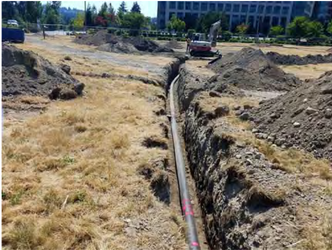
STA 4+75 LOOKING SOUTHWEST
