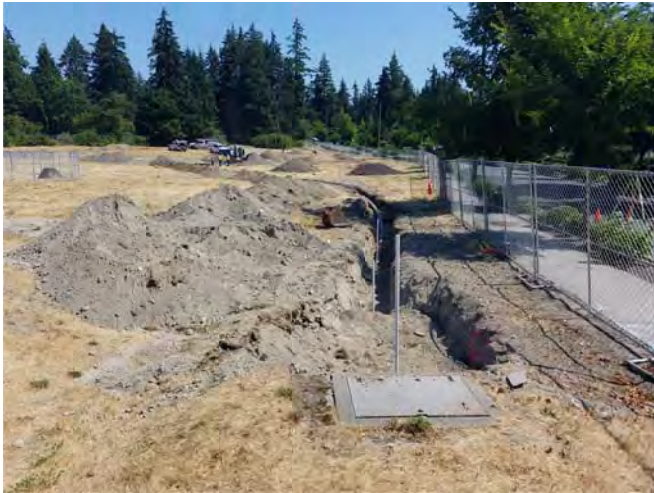
STA 0+80 LOOKING EAST TO CT-6R
