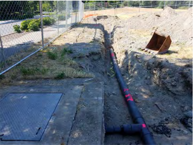
STA 1+57 LOOKING WEST TO CT-6R
