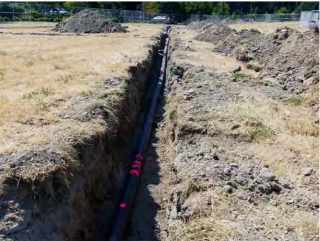
STA 3+20 LOOKING WEST
