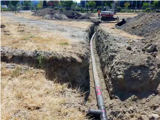
STA 4+55 LOOKING SOUTHWEST
