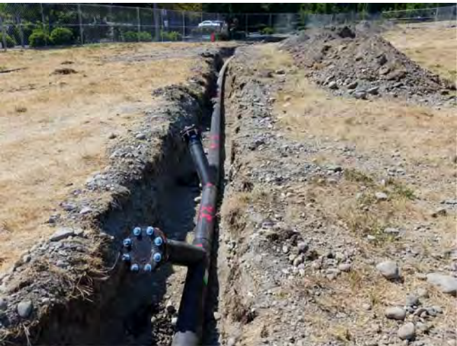
STA 2+50 LOOKING WEST
