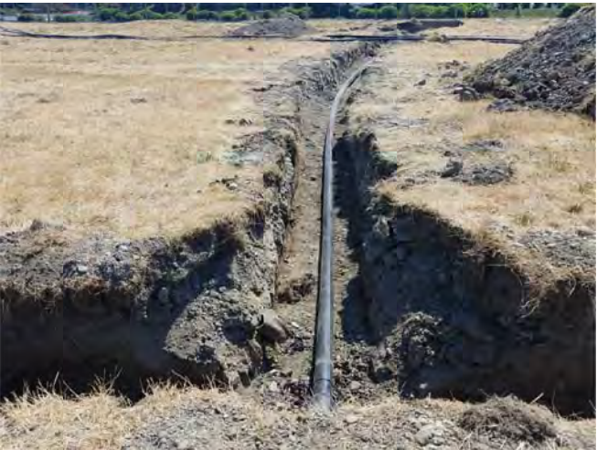
STA 2+82 LOOKING SOUTH TO EW-3R
