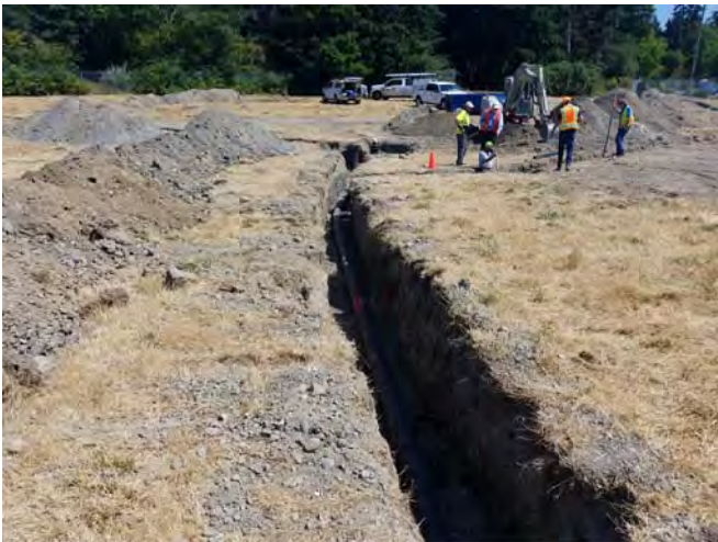
STA 3+20 LOOKING EAST
