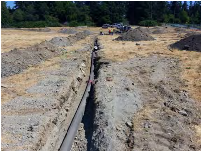
STA 2+25 LOOKING EAST
