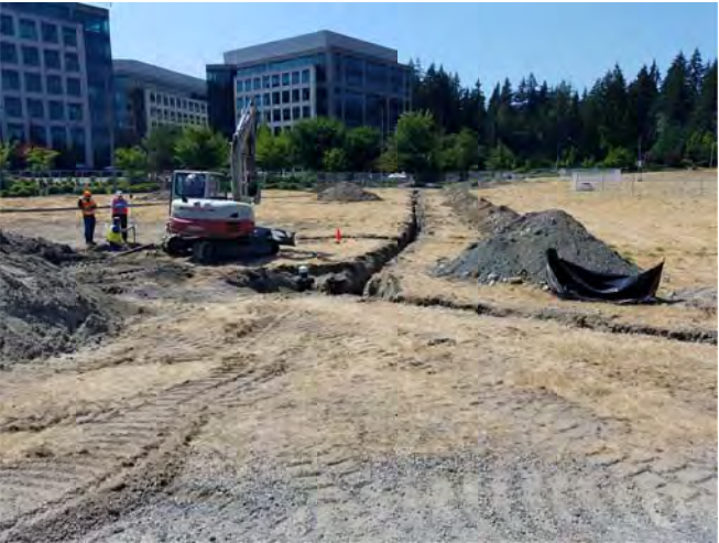
VIEW LOOKING WEST TO CT-5R2
