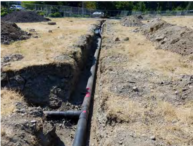
STA 2+85 LOOKING WEST
