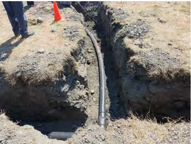
STA 3+50 LOOKING SOUTH TO EW-2R & EW-18
