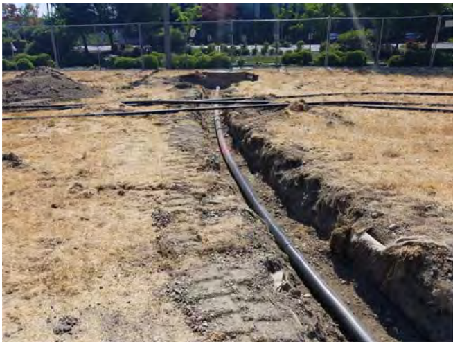
BRANCH PIPE TO EW-3R LOOKING SOUTH
