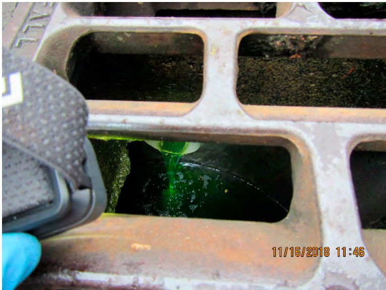
Photograph 12: Visual confirmation of dye solution discharging to catch basin CB-10 immediately following the initiation of dye pumping into the roof drain located at the northwest corner of the SPTF Shop.
