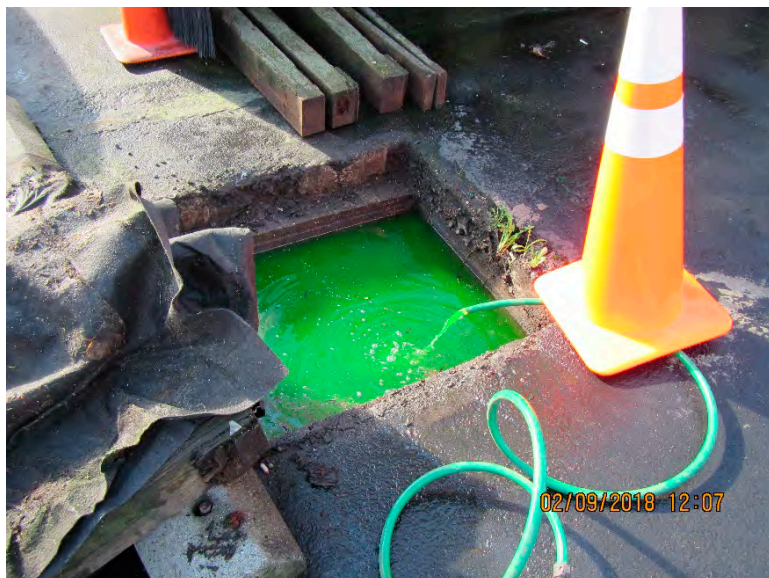
Photograph 5: Pumping fluorescein dye solution into CB-05.
