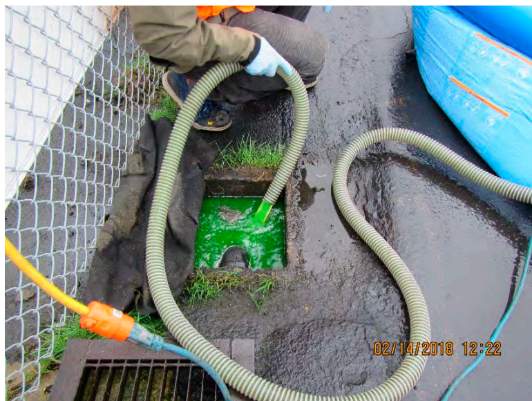
Photograph 1: Pumping fluorescein dye solution into catch basin CB-01.
