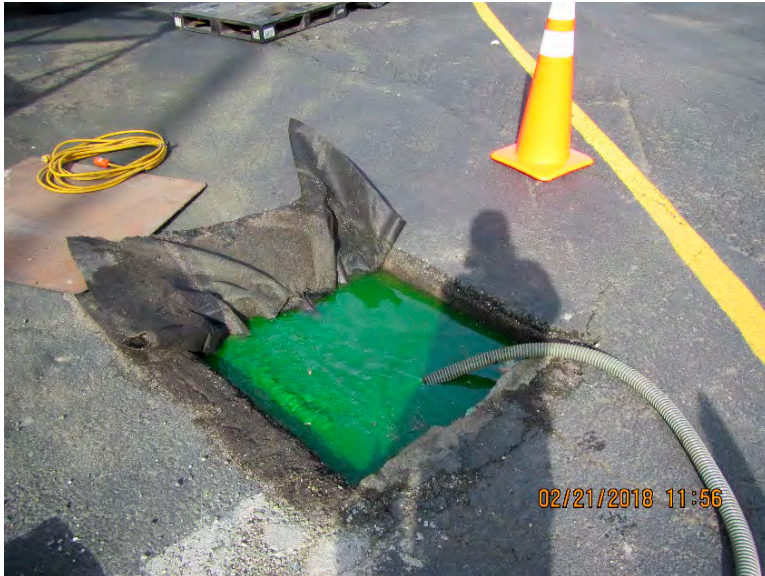
Photograph 3: Pumping fluorescein dye solution into CB-02.
