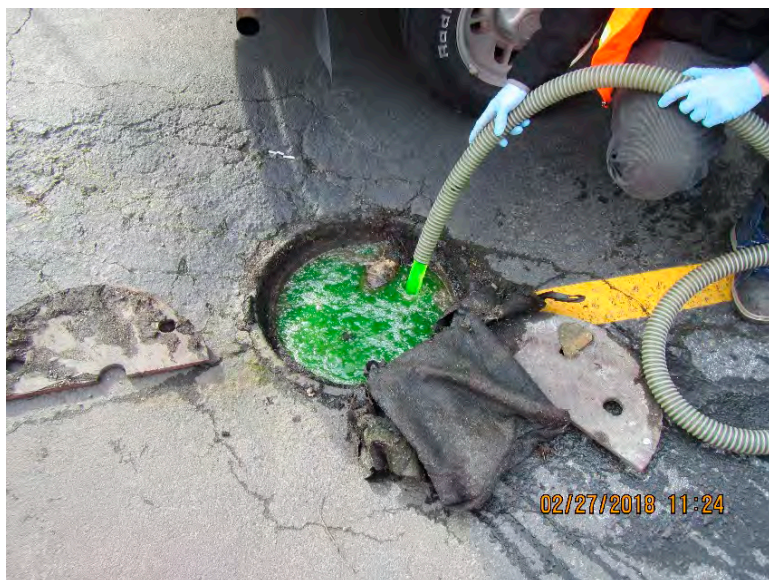
Photograph 7: Pumping fluorescein dye solution into CB-06.
