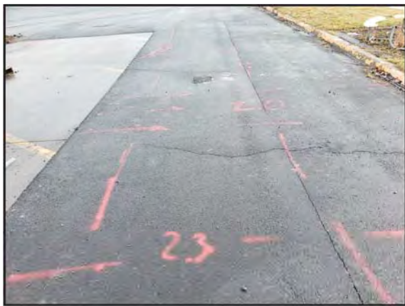
Marked Subsurface Utilities South of UST Basin in the Vicinity of AB4
