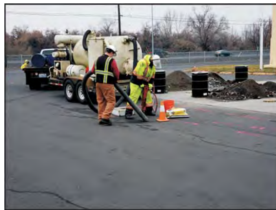
Air-knife Operations at Soil Boring AB1
