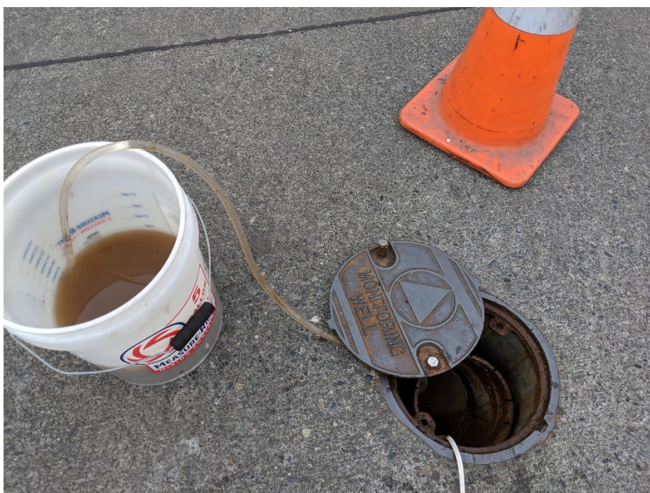
Photo 2. Turbid water being pumped out of well DW-3.
