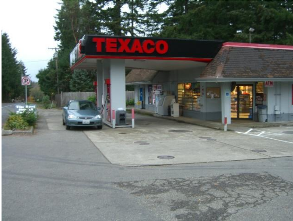
Photo 1: Canopy Above Excavation Area - from the south
