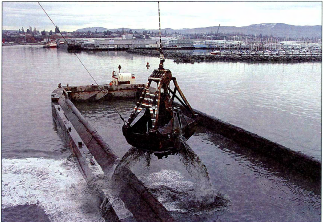
18. U.S. Army Corps of Engineers dredging of Squalicum Creek Waterway.
