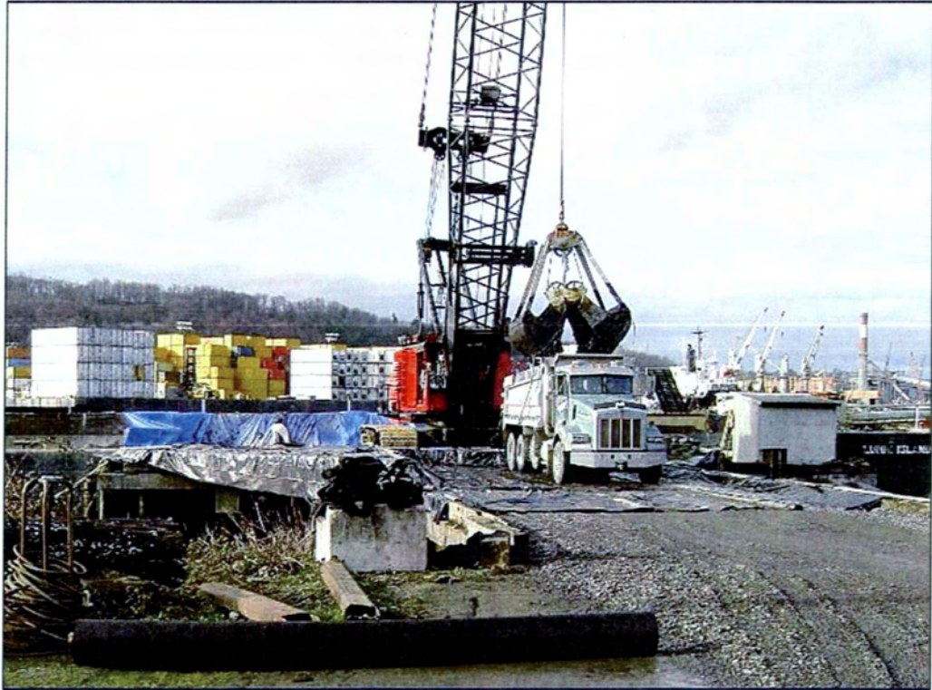
13. Sediment offloading at Alaska Logistics facility.
