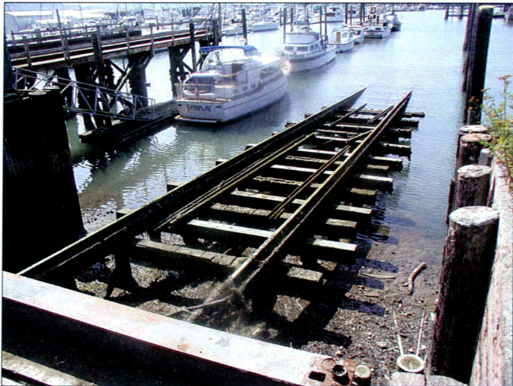
4. Former marine railway.
