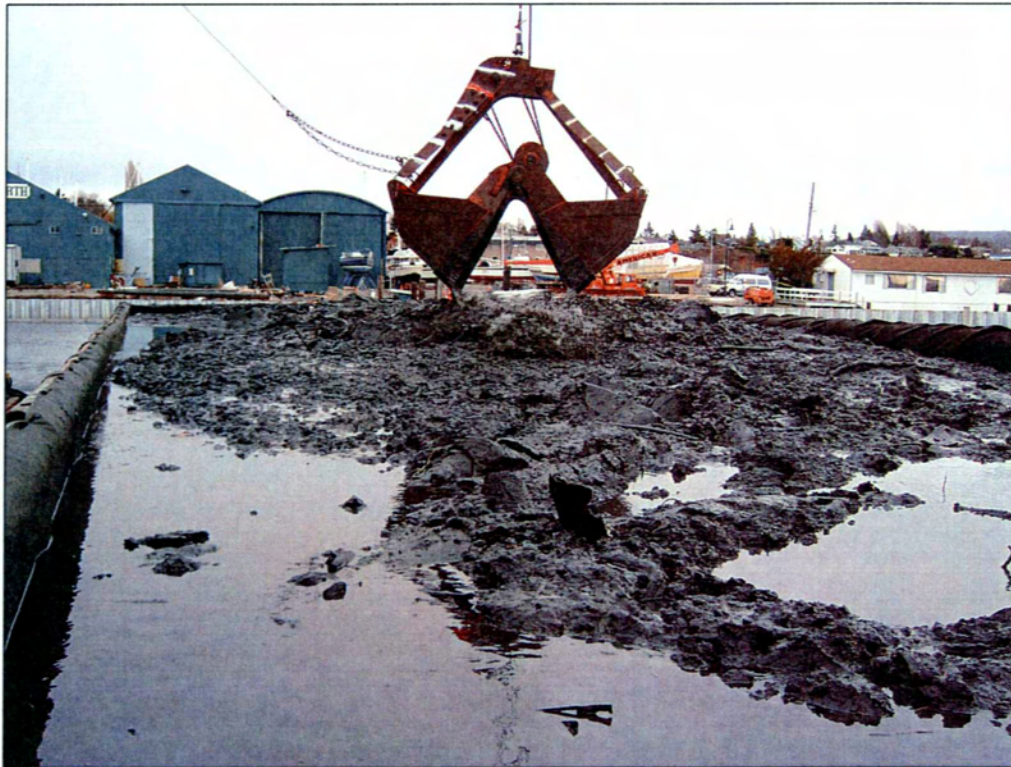
10. Initial barge load of dredge spoils.
