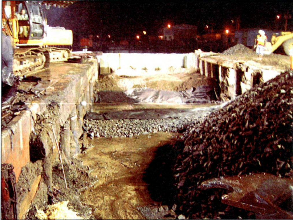
17. Marine railway well excavation/backfilling on January 21, 2004.
