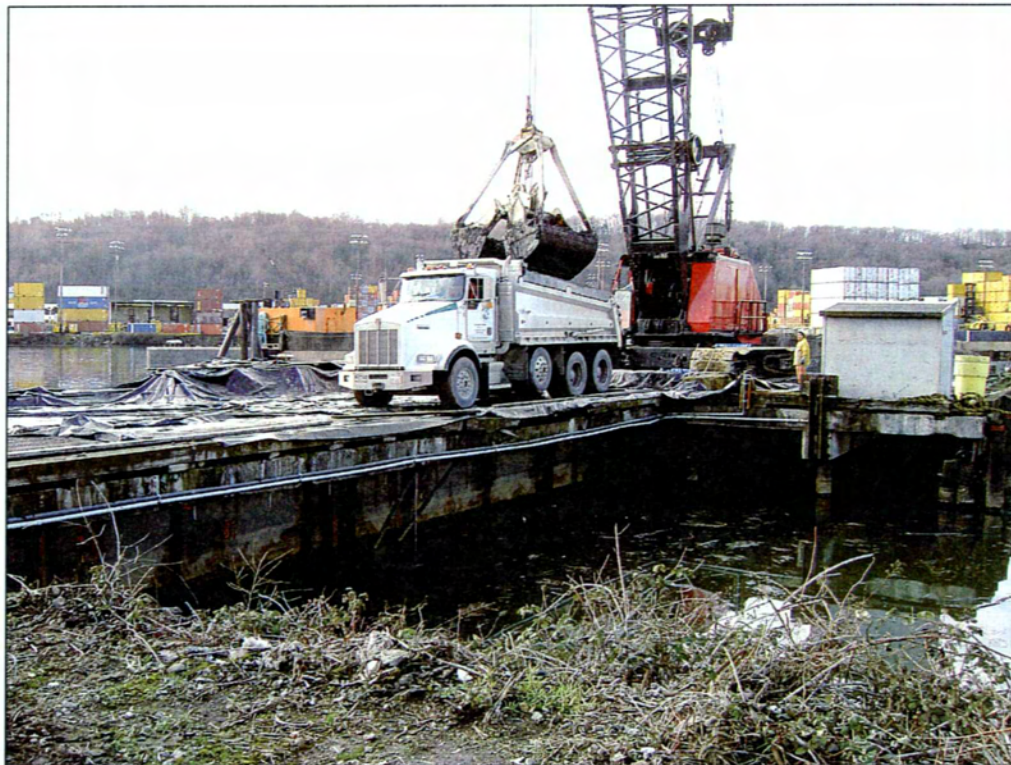
12. Sediment offloading at Alaska Logistics facility.
