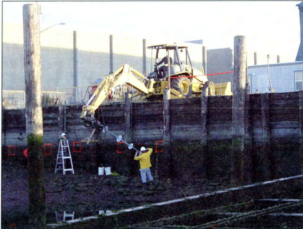
21. Helical tieback anchor installation for new bulkhead.
