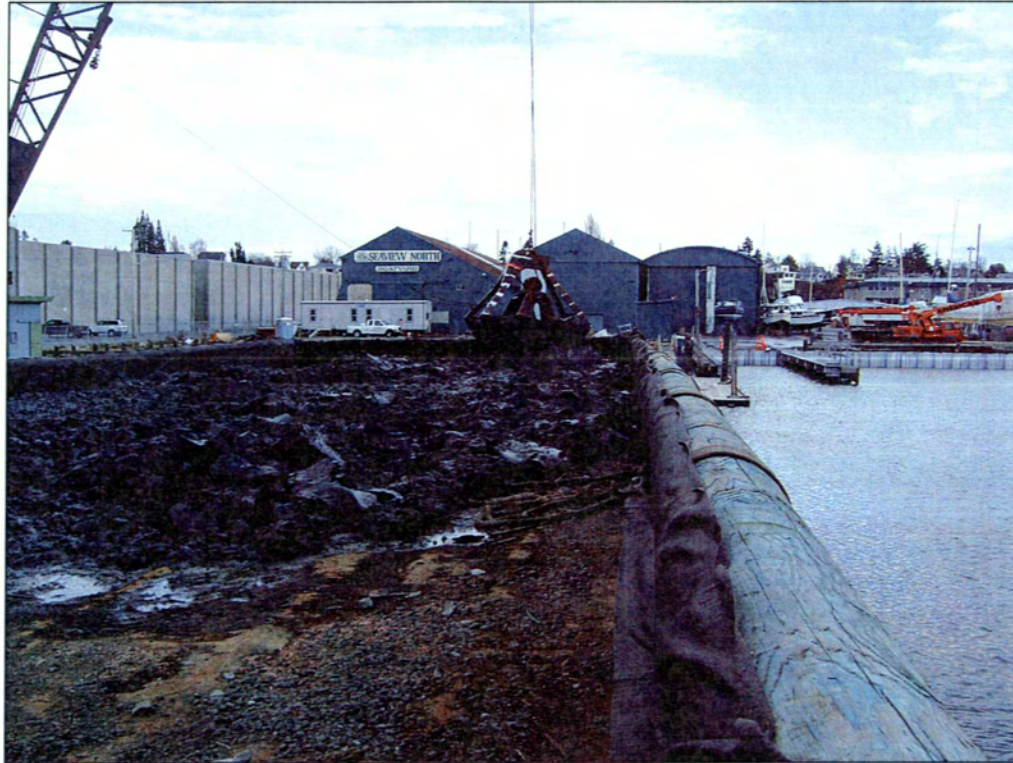
9. Initial loading of dredge spoils on flat deck barge.
