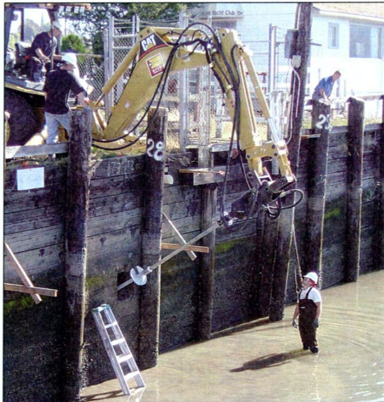
22. Helical tieback anchor installation for new bulkhead.
