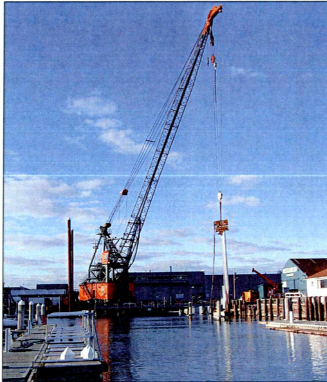
23. Installation of new sheetpile bulkhead.
