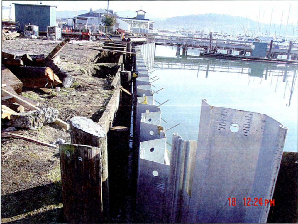
25. New sheetpile bulkhead installed in front of old timber bulkhead.
