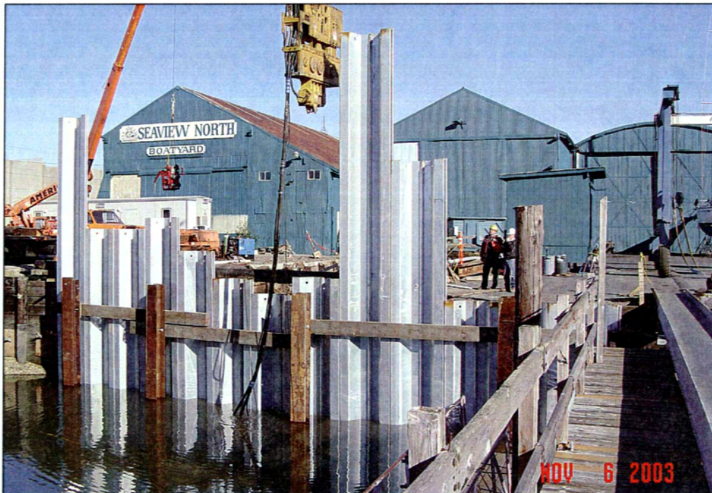
24. Installation of new sheetpile bulkhead across marine railway well.
