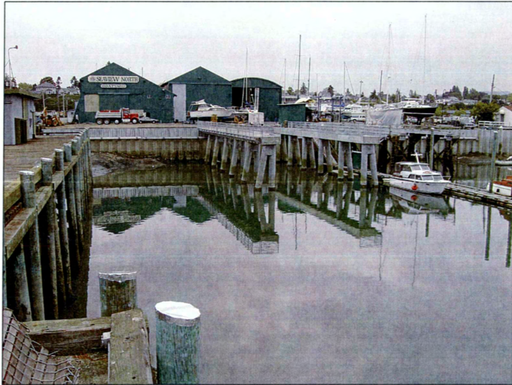
33. Post-construction view of redeveloped Gate 2 Boatyard with new 150-ton travel lift piers.
