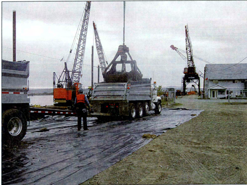
15. Sediment offloading at American Construction's south yard.
