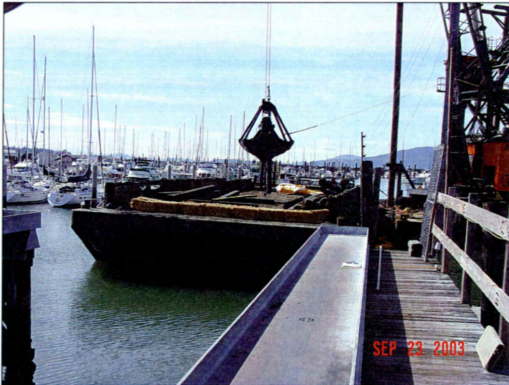
6. Marine railway demolition debris.
