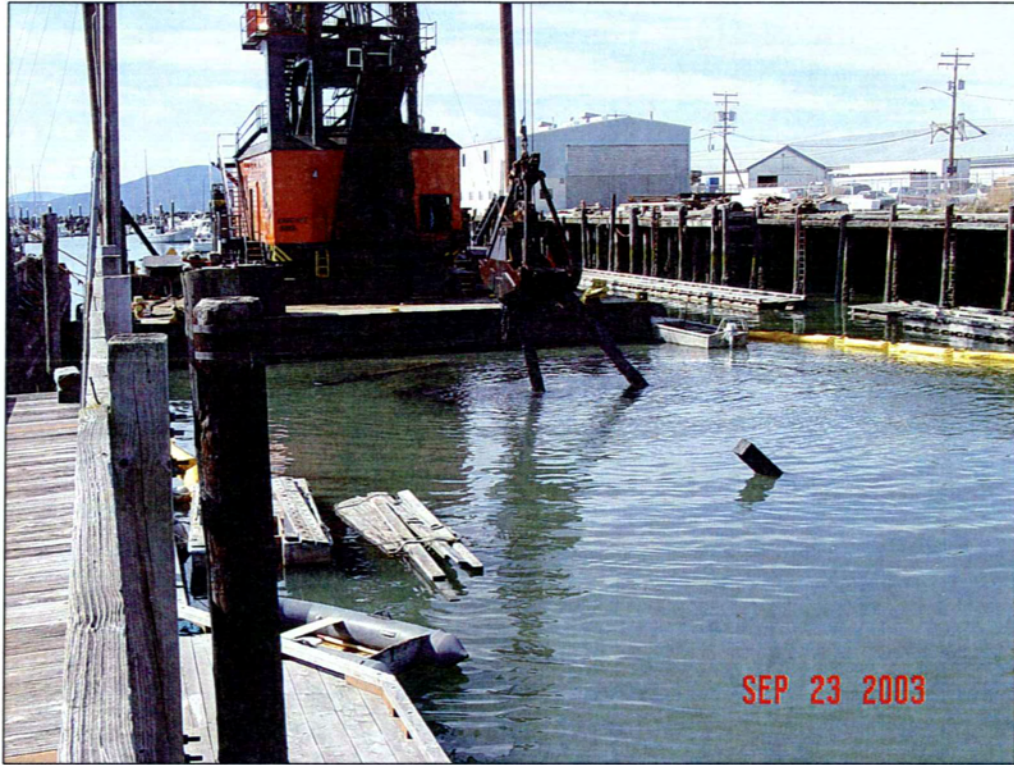
5. Marine railway demolition.
