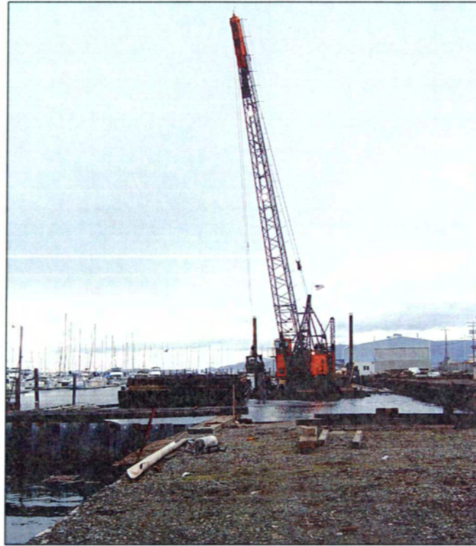
7. Initial sediment dredging on December 24, 2003.
