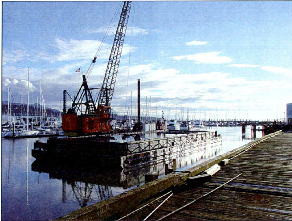
11. Barge with dredge spoils.
