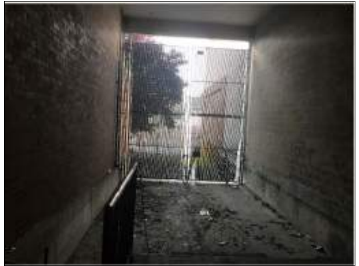
14. View of loading bay
