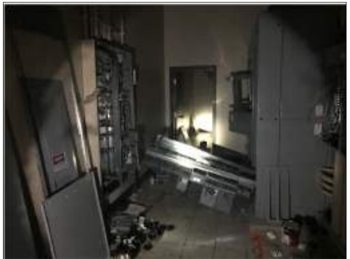
10. View of former electrical room
