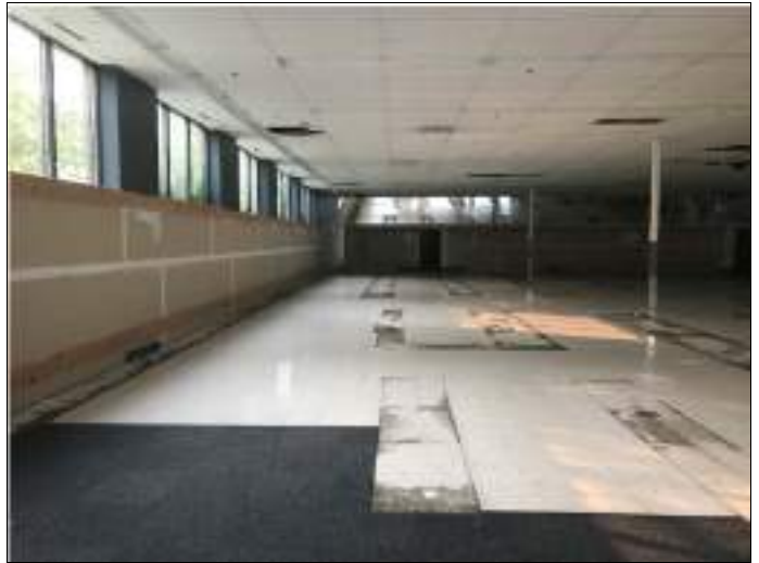
8. View of former retail area
