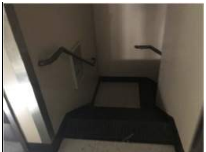
24. View of staircase
