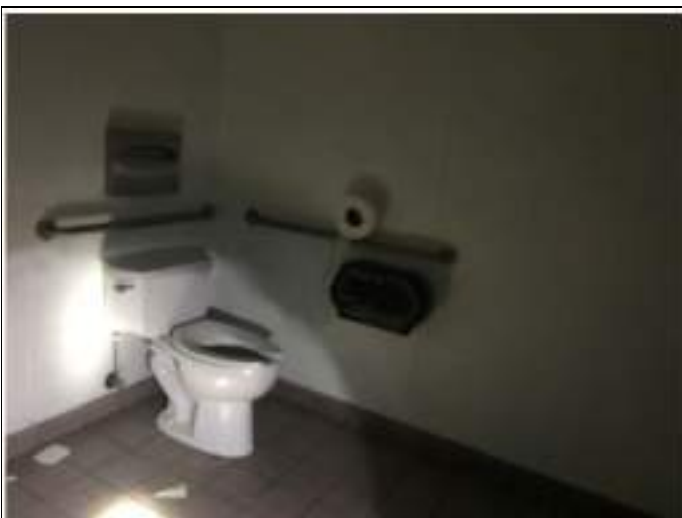
23. View of restroom
