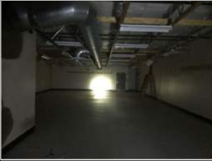
13. View of mezzanine area
