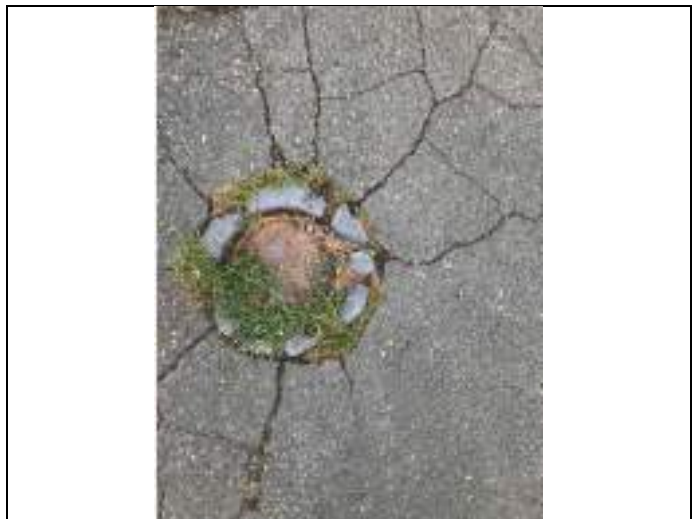
6. View of monitoring well on southwestern portion of subject property
