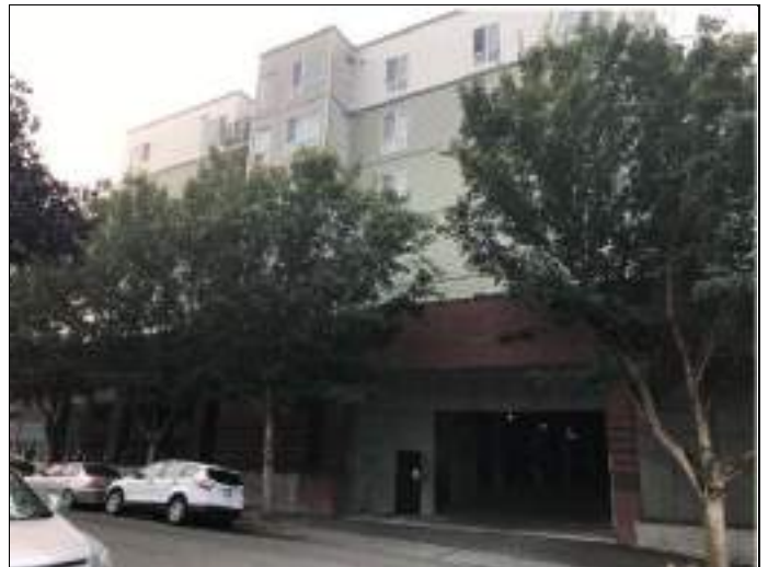
16. View of southern adjacent property
