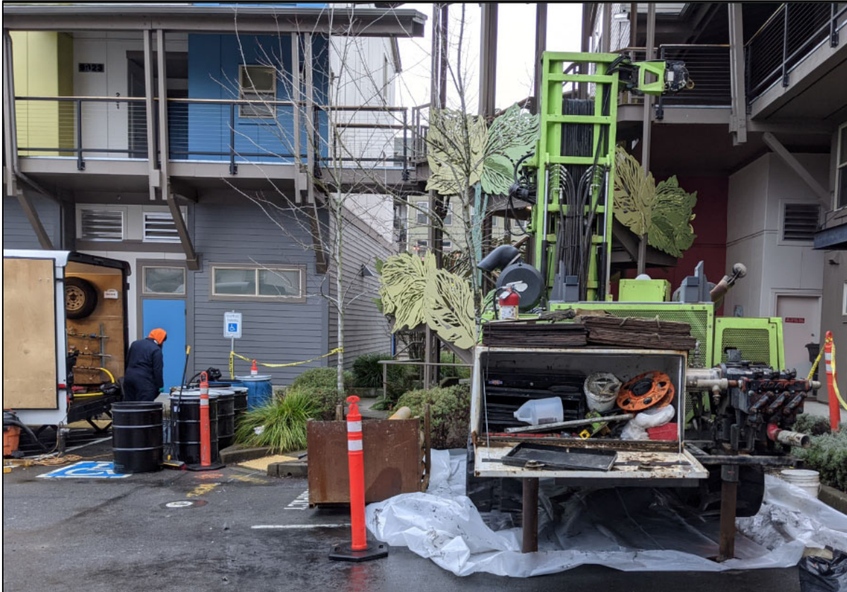
Photo 1: Sonic rig setup during injection activities. Photograph illustrates secondary containment and designated work zone in the parking lot area.
