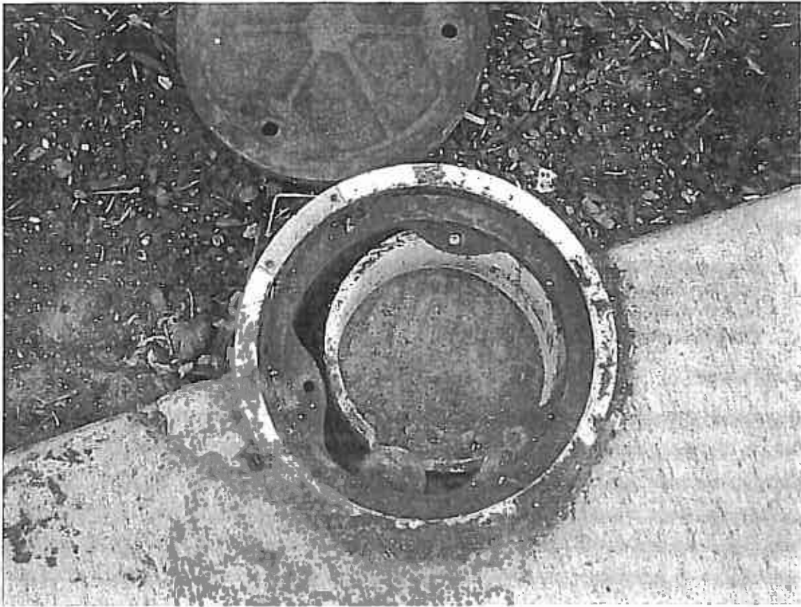
Treatment well MW-12 closed with concrete April 17, 2008
