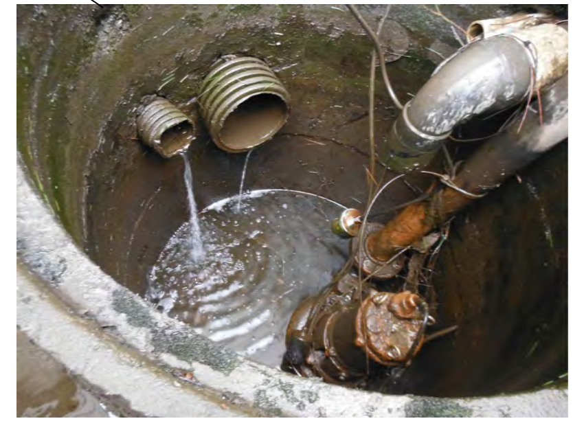
PHOTO OF THE NORTH TRUCK BAY SUMP
