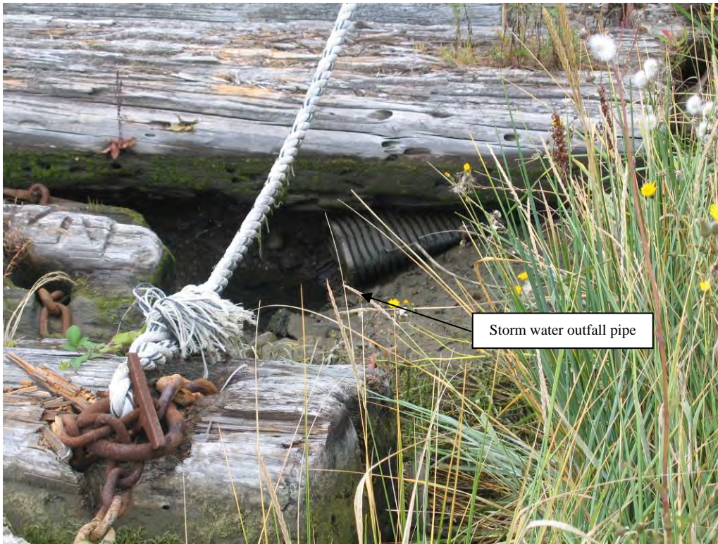
3. View of the storm water outfall 002 - proposed sediment sample location 3SED2-P
