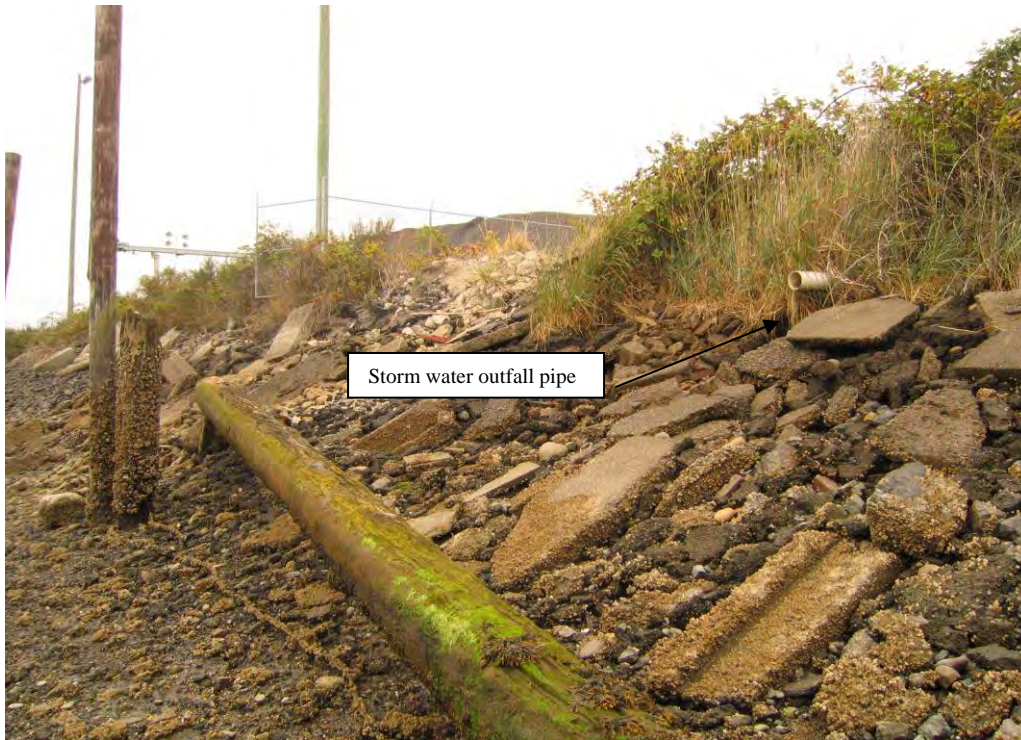
9. View storm water outfall 0X2 – proposed sediment sampling location 3SED5-P
