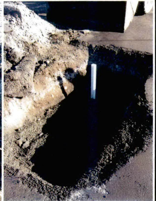
Photos 2-3: Example of typical installation of slotted pipe in test pit
