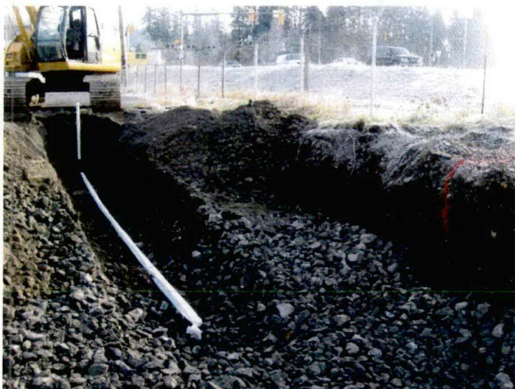
Photo 3: Eastern infiltration pipe. Installed atop quarry spalls, backfilled with visible pea gravel/pit run.
