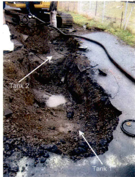
Photo 2: View of top of tanks 1 and 2 after excavation of overlying soils.
