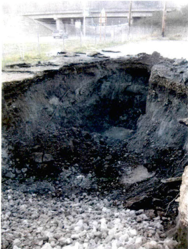
Photo 3: Western limits of excavation at end of day 1/19/09. Quarry spalls used to backfill excavation visible in foreground of photo.
