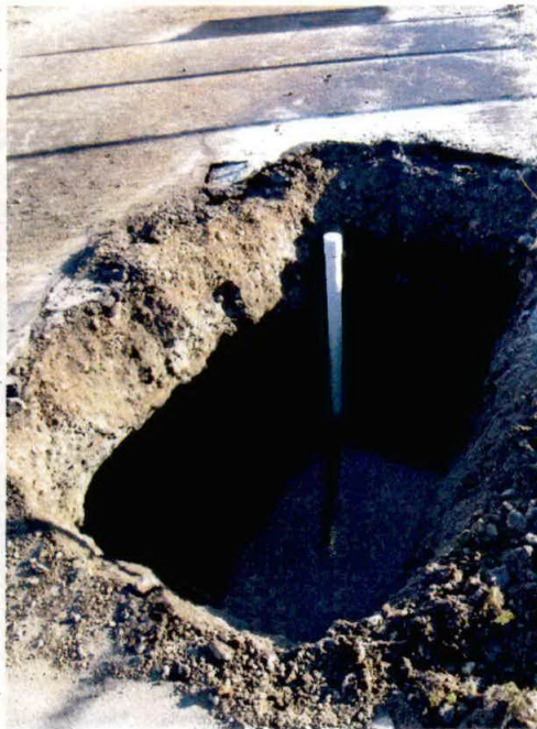
Photos 2-3: Example of typical installation of slotted pipe in test pit
