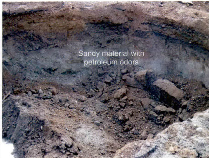
Photo 2: West/southwest limits of excavation (1/20/09). Grey soil on two visible sidewalls had strong petroleum odors and resulted in high PID readings.
