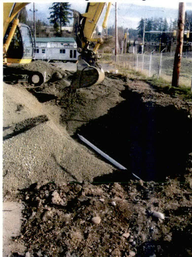
Photo 4: Western infiltration pipe. Eastern pipe is located behind excavator bucket.
