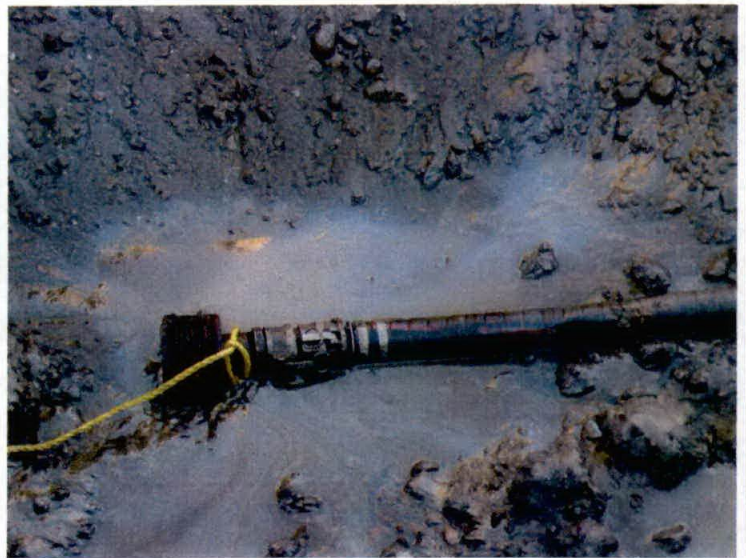
Photo 2: Example of sheen noted on water pumped from excavation on 1/19/09.
