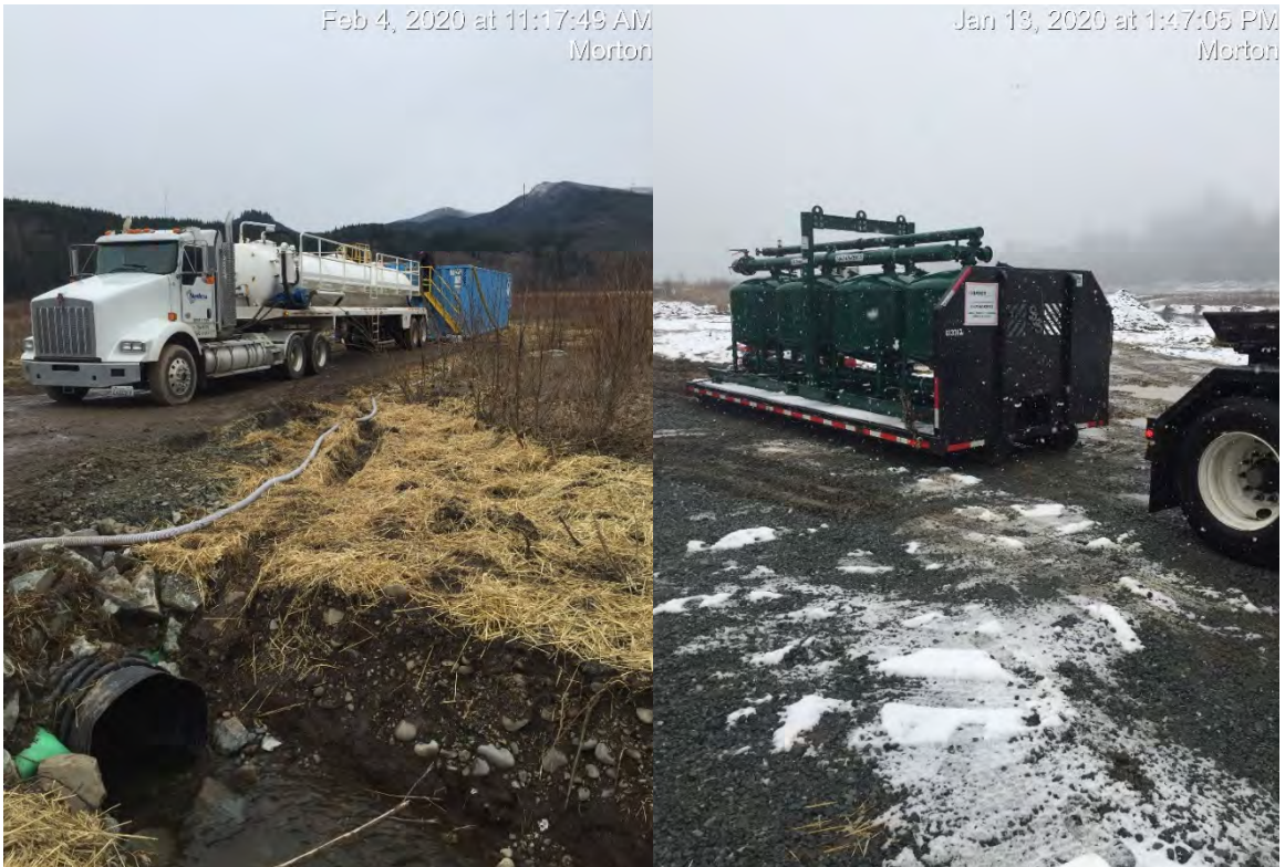
Photographs 9 and 10: On-site dewatering system.
