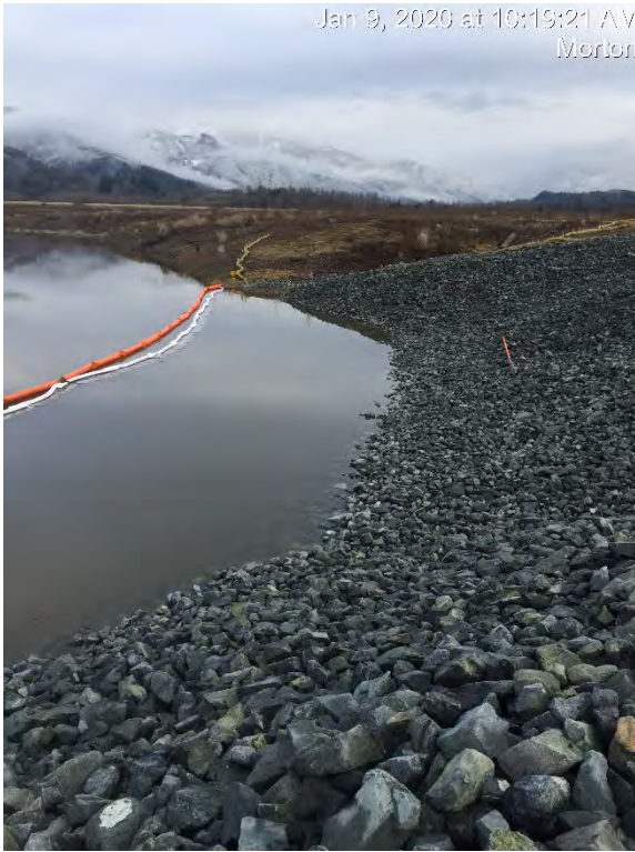
Photograph 21: Completed cap and elevated water level. View looking east.
