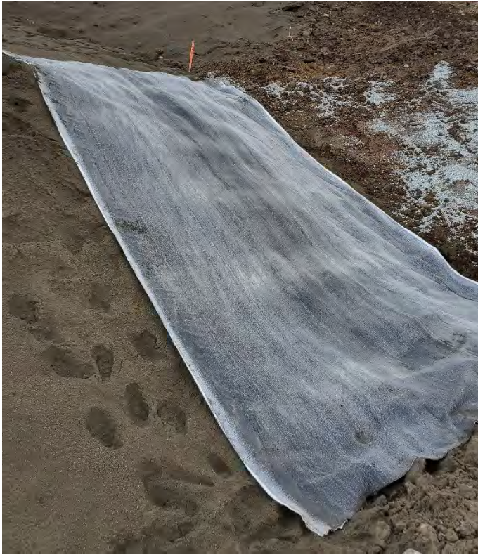
Photograph 15: Installing RCM over clean sand layer.
