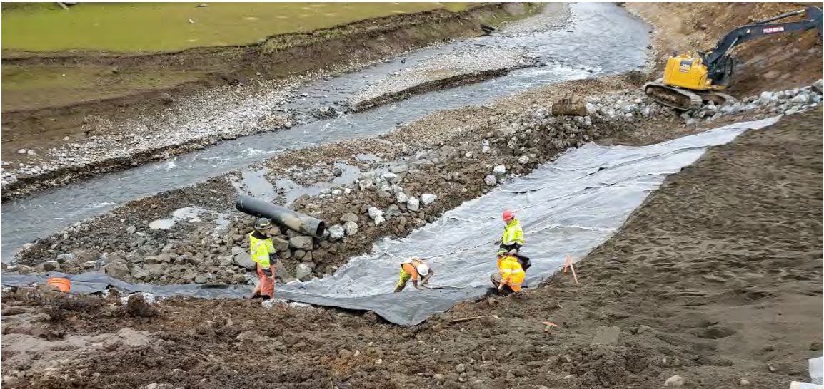
Photograph 16: Installing RCM over clean sand. View looking north/northeast.
