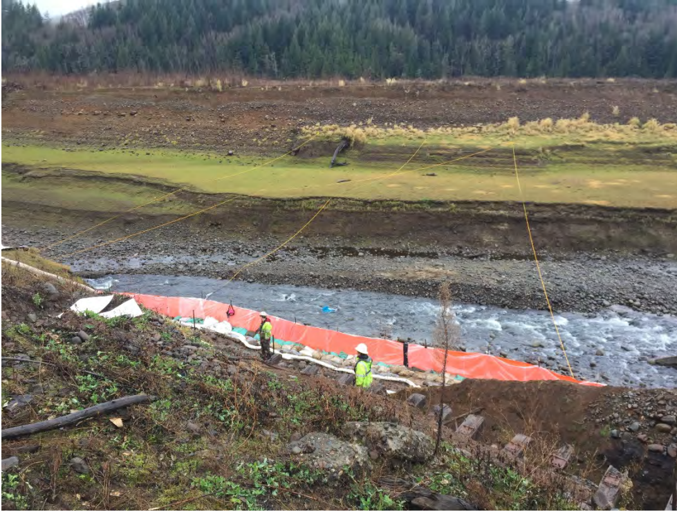
Photograph 1: Sea curtain at the bottom of the cap excavation area.
