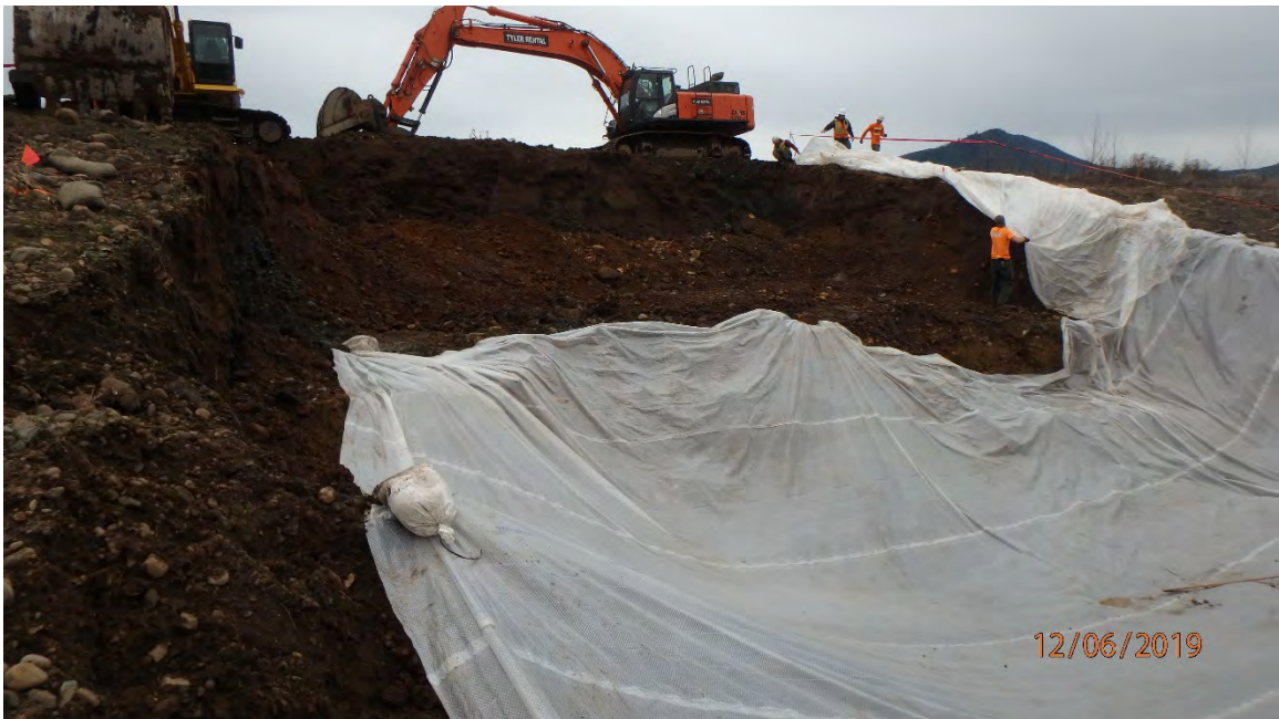
Photograph 11: Completed excavation for the cap installation.
