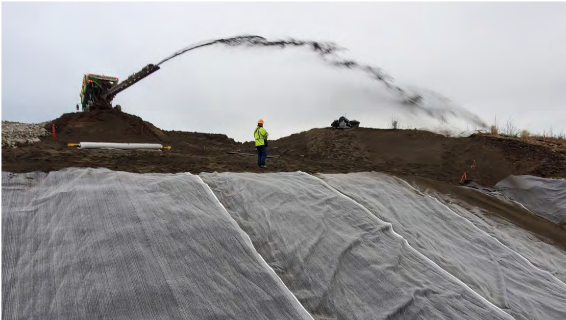
Photograph 17: Placing clean sand over the RCM.
