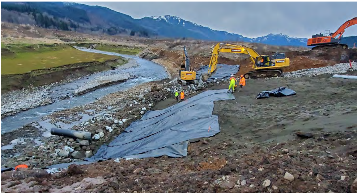
Photograph 18: Placing high-strength geotextile over the clean sand layer.
