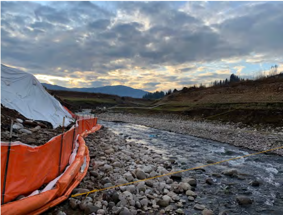
Photograph 2: Sea curtain lining creek at the bottom of cap excavation area.
