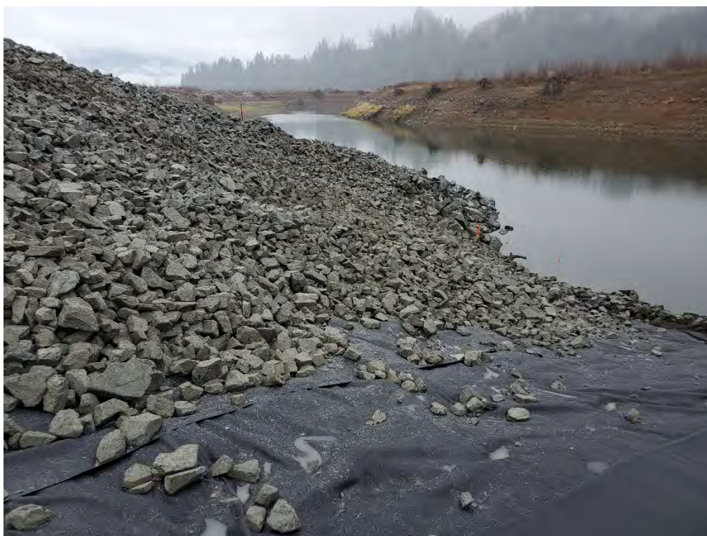
Photograph 20: Placing large quarry spalls over the geotextile.
