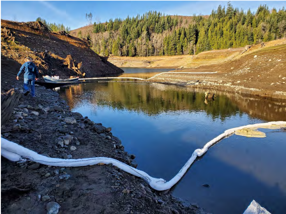
Photograph 3: Booms placed downstream of excavation area.
