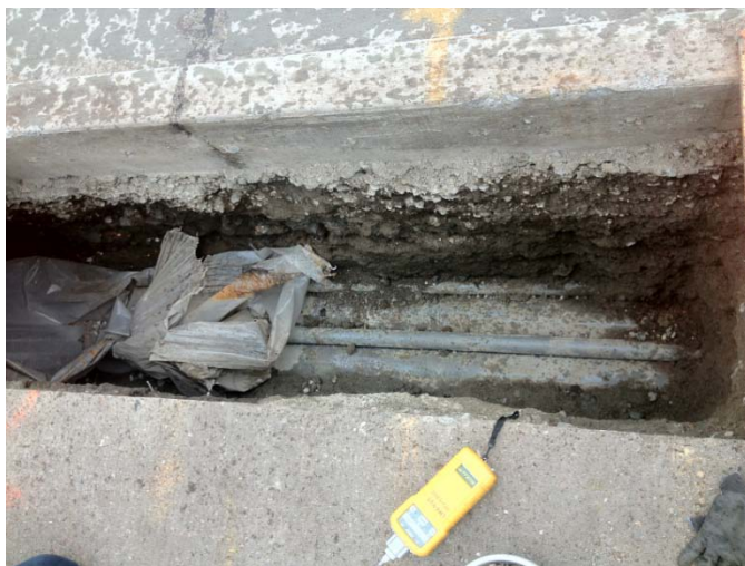
West Wall Final Excavation Depth of 3 feet on June 26, 2012
