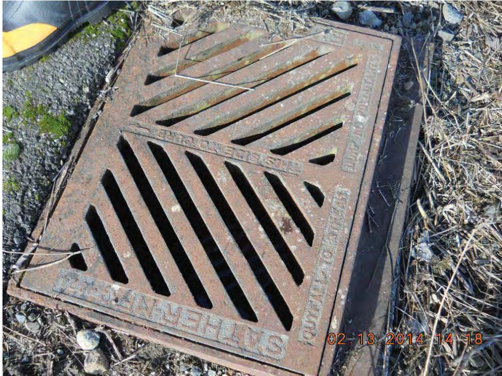
2. Middle catch basin; unable to open during site visit.
