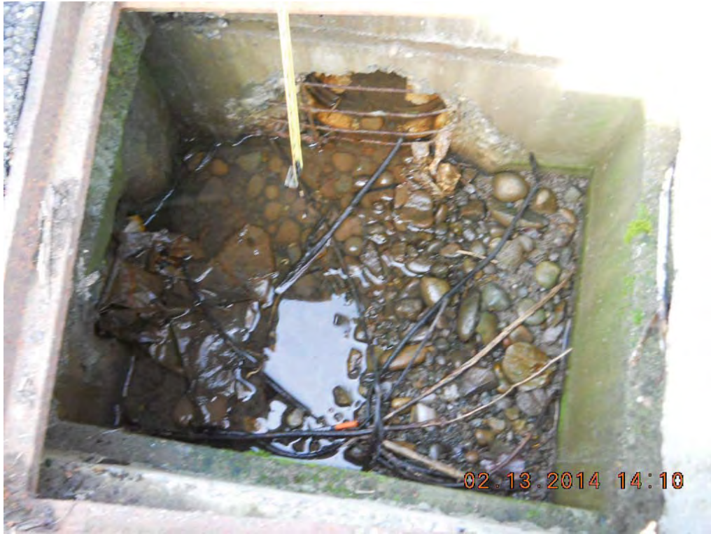
1. South catch basin
