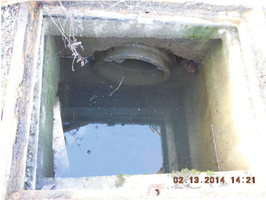
3. North catch basin.
