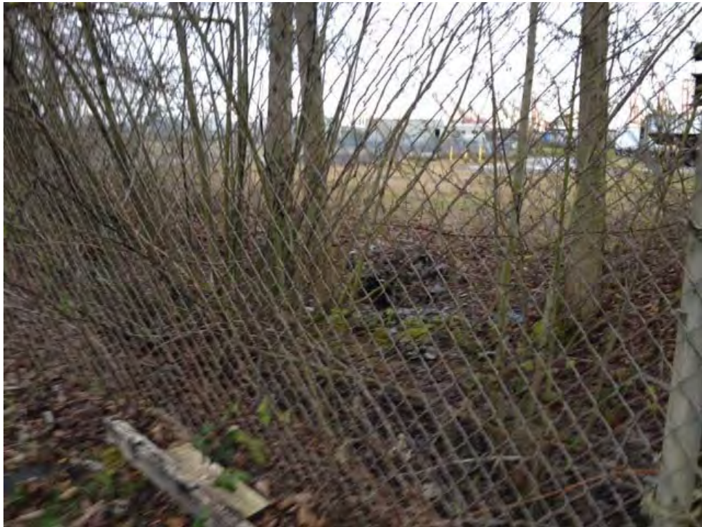
4. East ditch; shows inlet culvert from the north catch basin.
