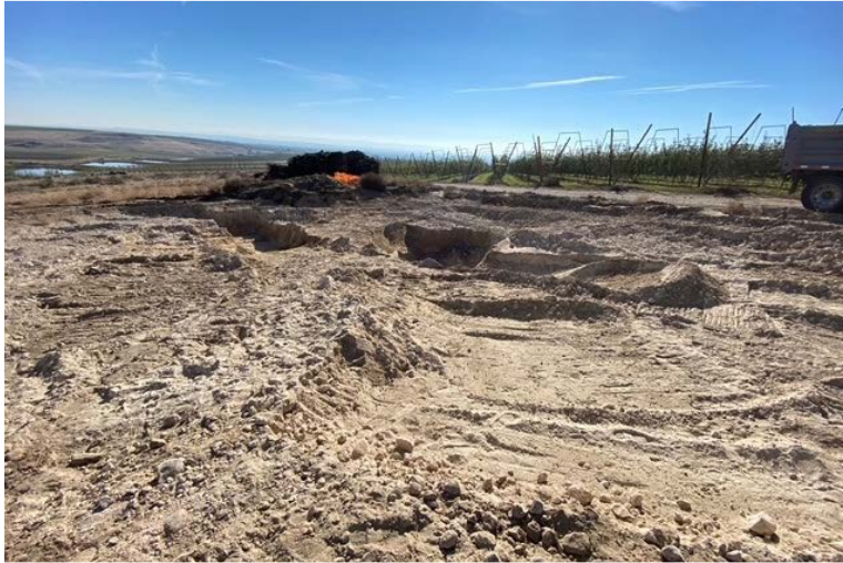
Looking southeast - excavation extent with average excavation depth of approximately 1 to 2 feet bgs.
