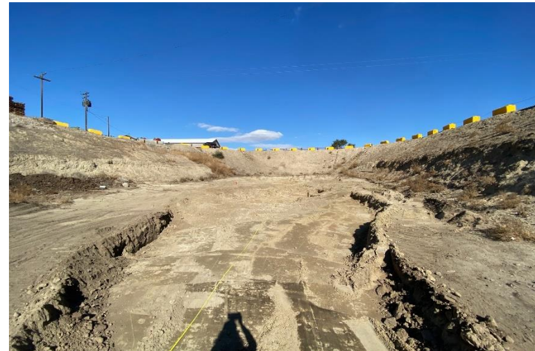
Looking north - final excavation extent.
