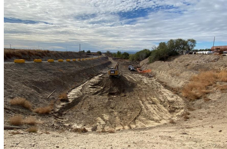
Looking south - excavation extent within embankment.
