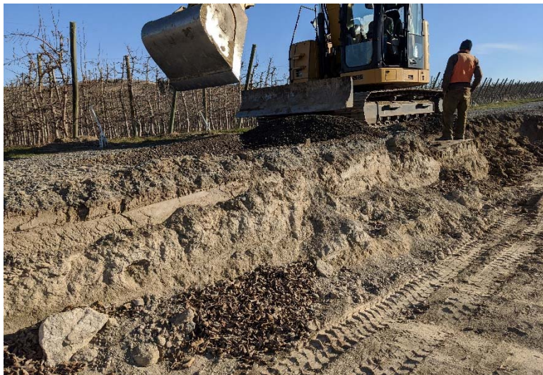
Looking northeast – View of north sidewall with maximum depth of 5-feet (03/18/20)
