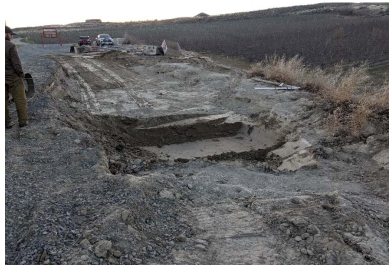
Looking east – Start of continued site remediation (03/18/20)
