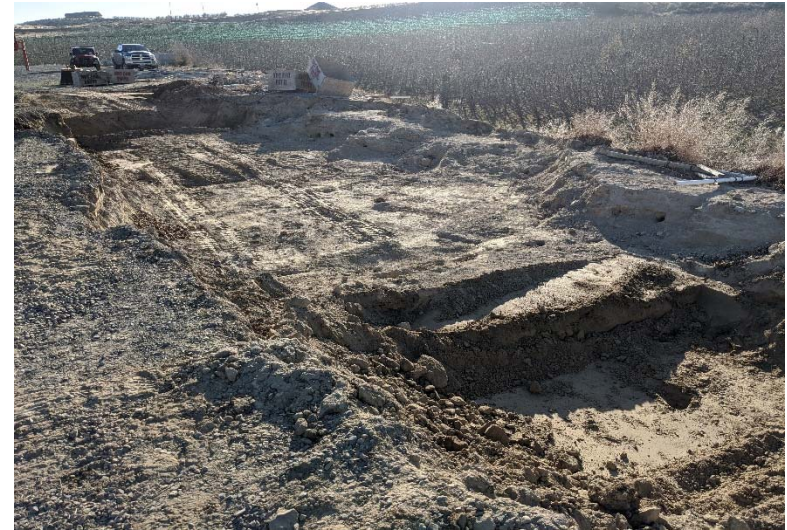
Looking southeast – View of south and east sidewalls (03/18/20)
