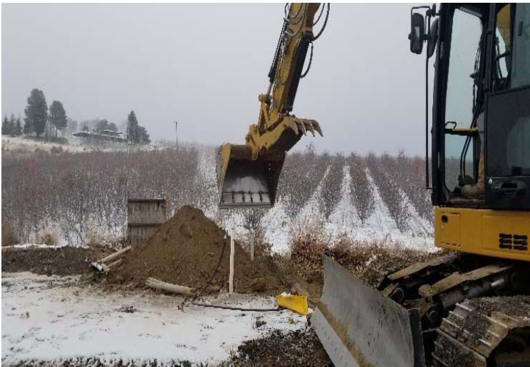
Looking south – Excavator removing water piping after disconnection. (12/03/19)
