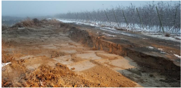
Initial Excavation Extents – December 3, 2019
