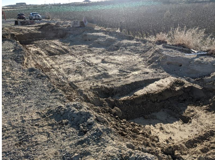
Final Excavation Extents – March 18, 2020
