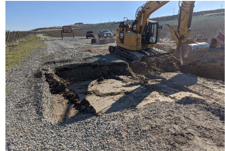
Looking east – Access road scraping for extent of petroleum contamination (03/18/20)
