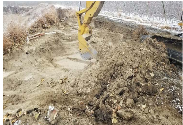
Looking west – Continued excavation towards the east. (12/03/19)
