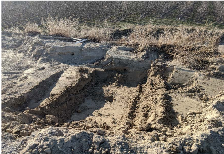
Looking south – View of excavated soils from the west portion (03/18/20)
