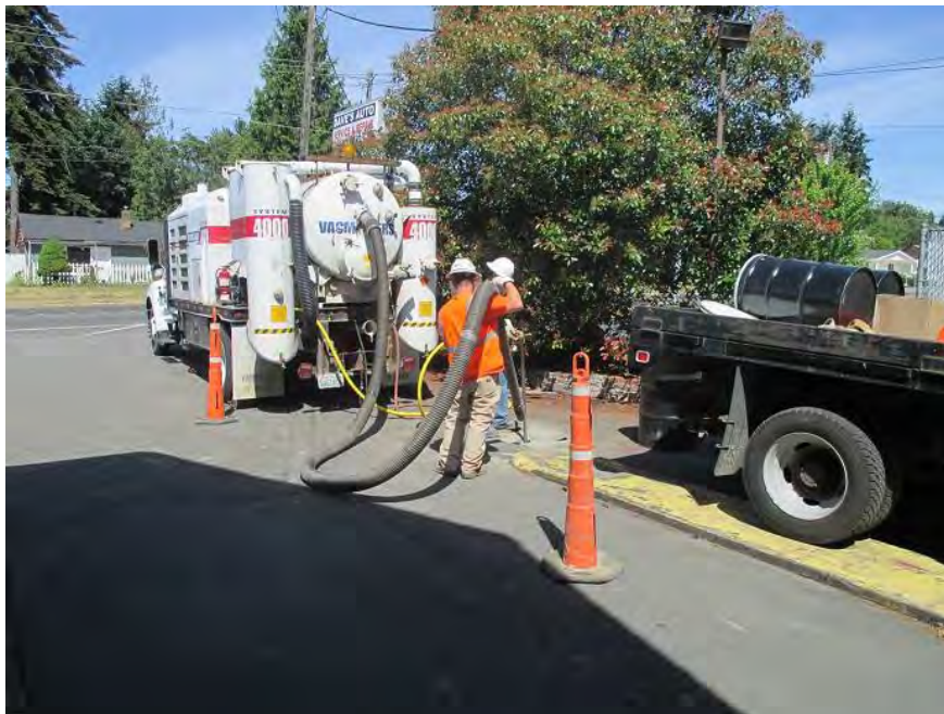
Photograph 2: Looking northwest at Vactor truck clearing well MW109
