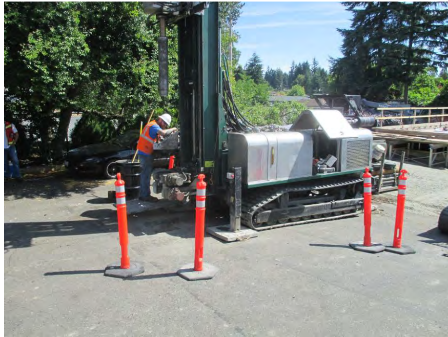
Photograph 1: Looking southeast at drill rig set up on well MW108
