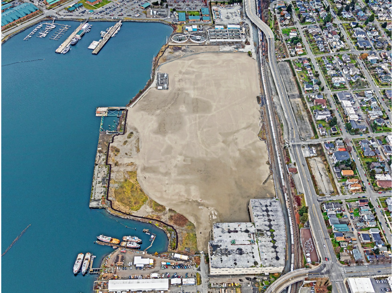
Figure 3: The Kimberly-Clark Worldwide, Inc. site facing north, December 2020
