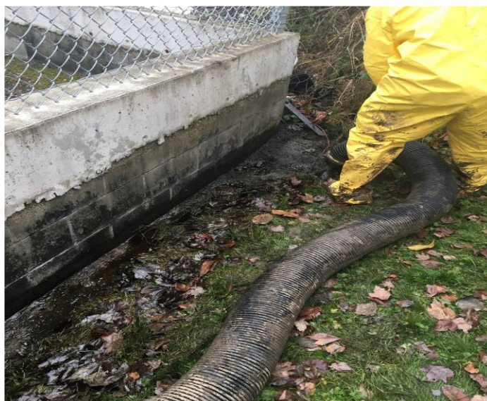
Photo 7: USE personnel removing impacts.
