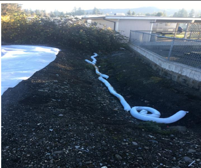
Photo 3: Site secured pending excavation operations.
