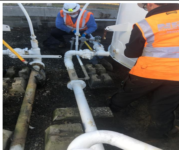
Photo 4: USE personnel removing impacts.
