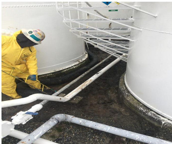
Photo 6: USE personnel removing impacts.
