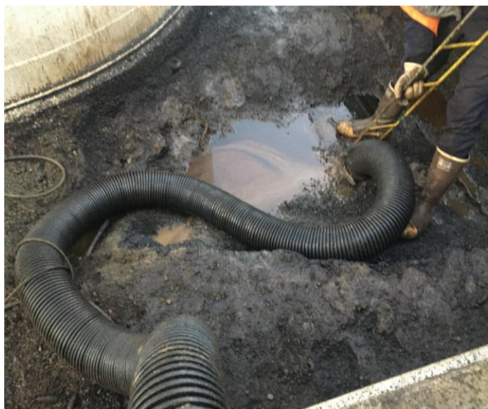
Photo 5: USE personnel removing impacts.
