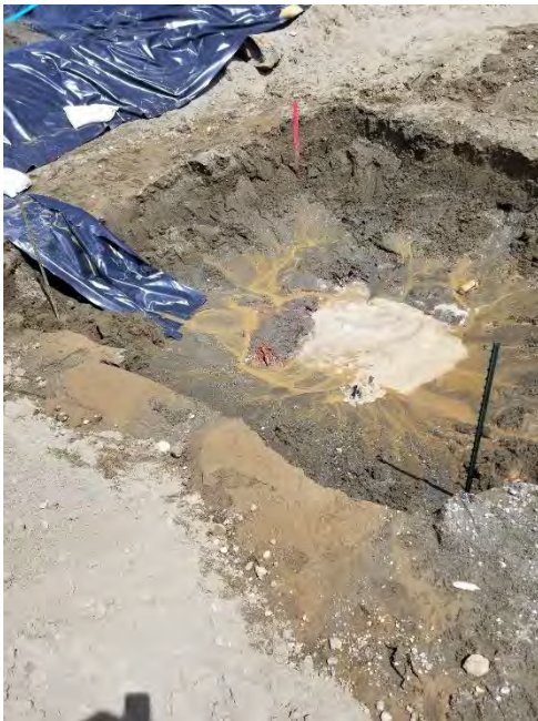
Photograph 2. CN-West initial excavation, dewatering turned off.
