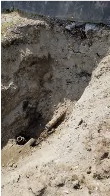
Photograph 1. Pipe G exposed near bulkhead, preplugging.
