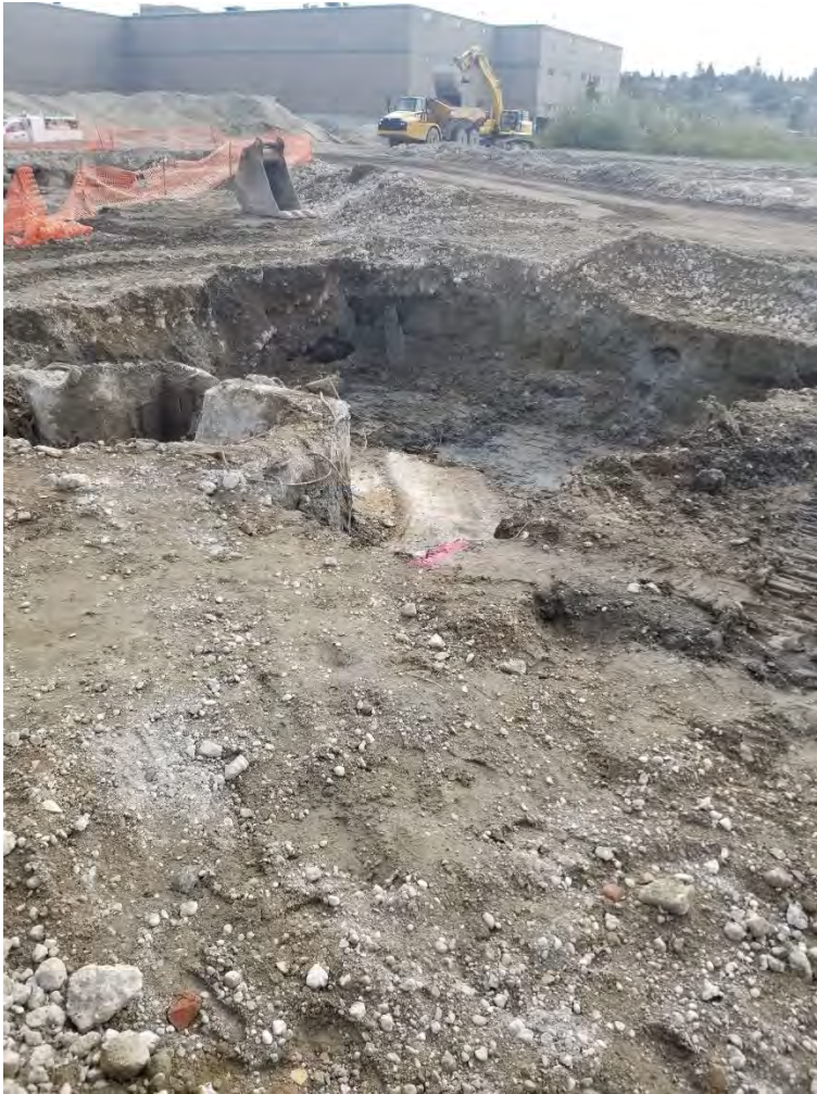
Photograph 1. Initial excavation limits, view to the southeast.
