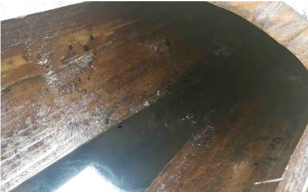
Photograph 4. Pipe C after vector cleaning (2).
