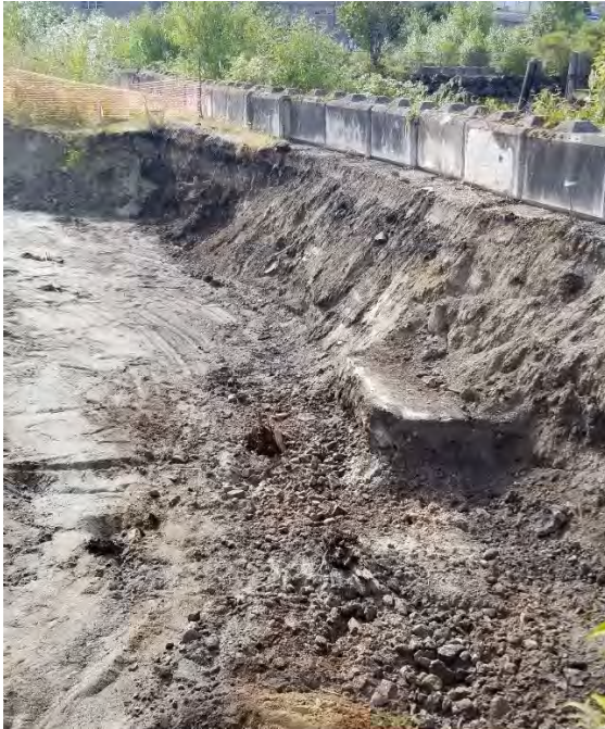
Photograph 5. South sidewall after ecology blocks moved back and first overexcavation performed.
