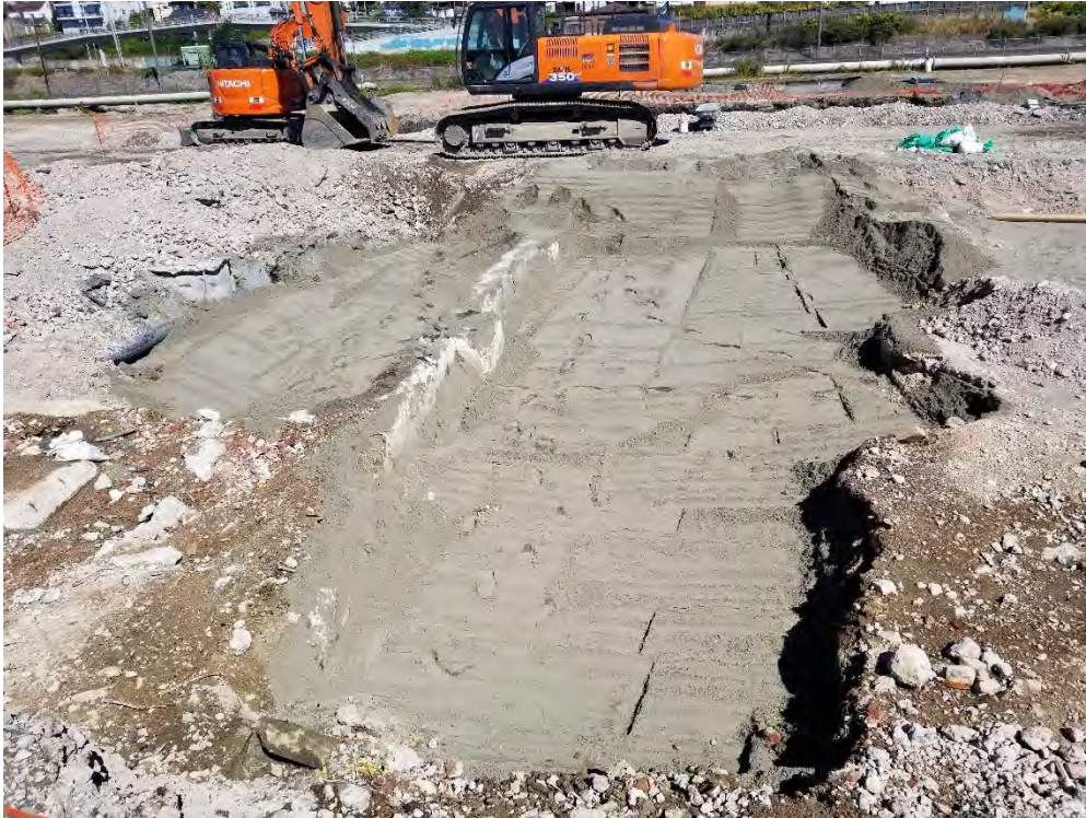
Photograph 9. PM-B-6 Area excavation backfilled.
