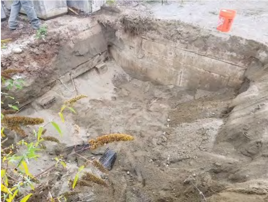
Photograph 1. Initial excavation above water table, 10/5/2020, view looking east-northeast.
