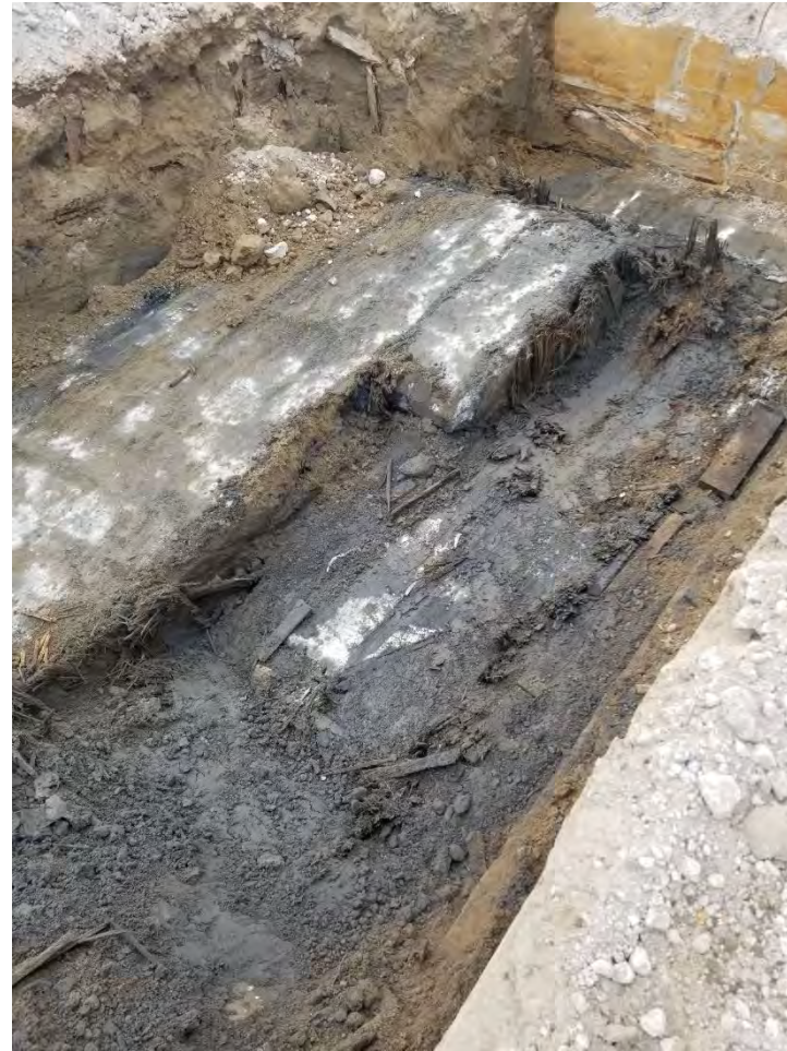
Photograph 6. Concrete slab in south sidewall of western excavation extension, beneath sidewall sample S-25 at approximately 5 feet bgs.
