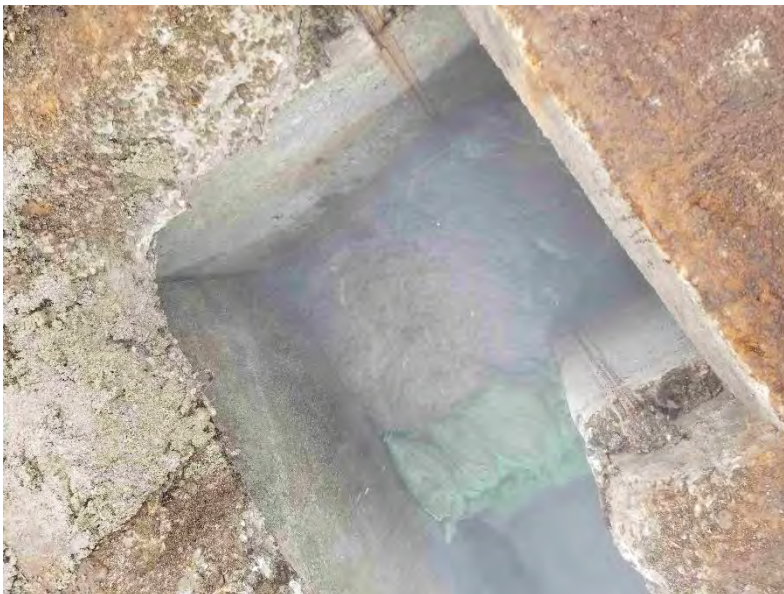
Photograph 6. CDF plug placed in bottom of vault covering pipe entry/exit points.
