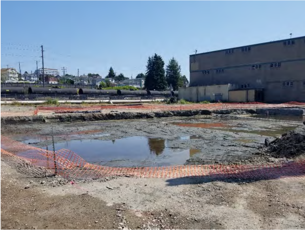
Photograph 11. Open excavation extent on 7/30/2020, view looking southeast.
