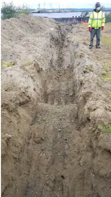
Photograph 2. Trench after Pipe G removal to ~78 feet inland.
