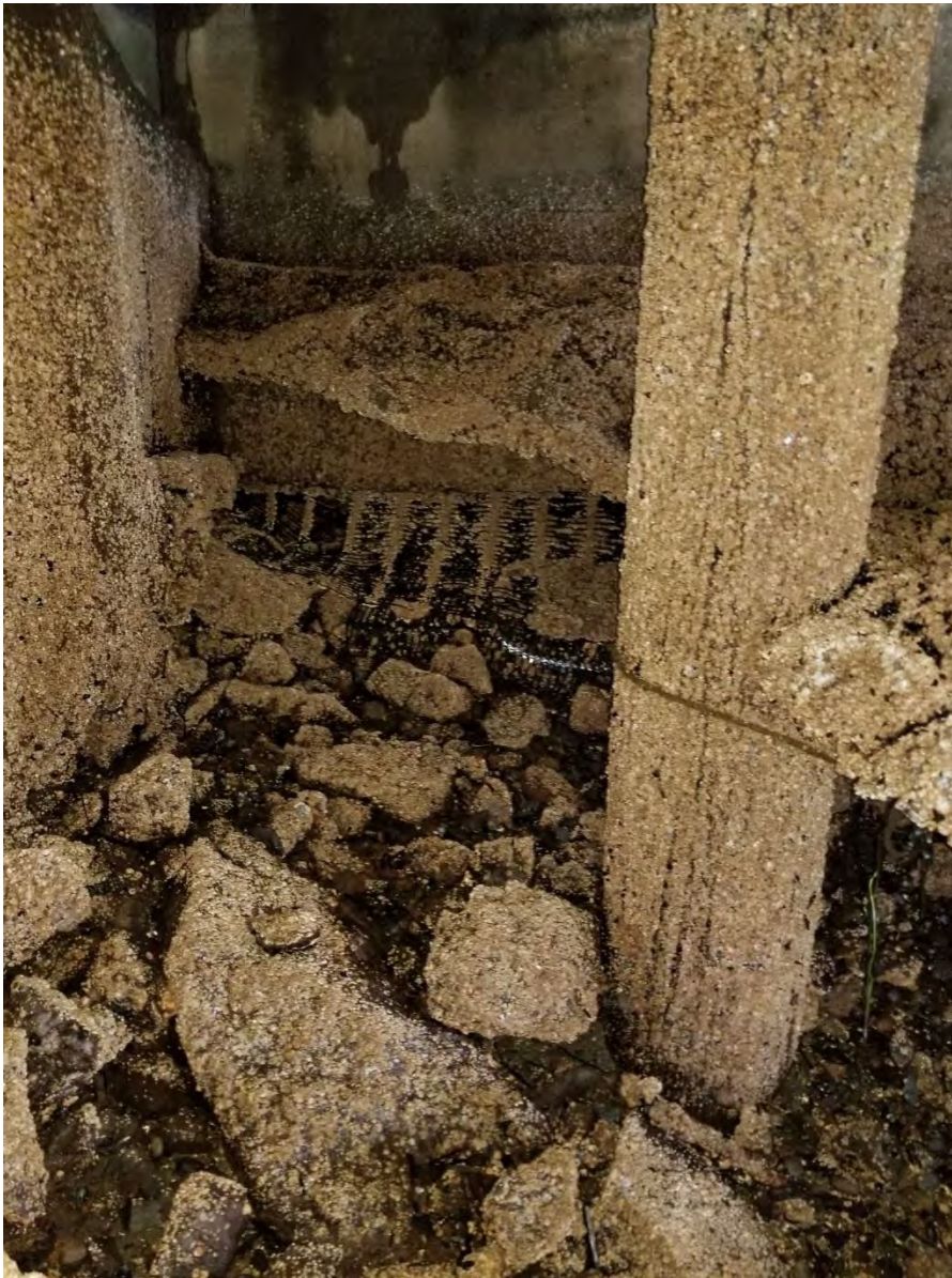
Photograph 5. View beneath wharf just west of BA-MW-7 excavation, looking east at concrete bulkhead. Black geotextile containing quarry spalls visible beneath bulkhead—same materials as in BA-MW-7 excavation immediately east of bulkhead, 10/12/2020.
