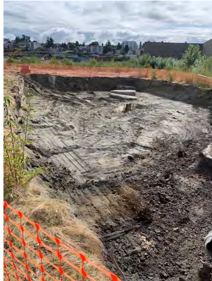
Photograph 4. Excavation looking east after first overexcavation.
