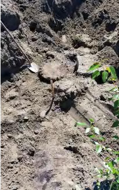
Photograph 1. Pipe C manhole adjacent to station 10+98.
