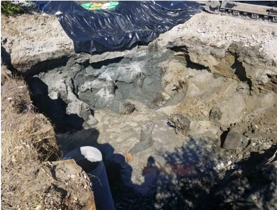
Photograph 1. Initial excavation limits on 8/28/2020, view looking northeast.
