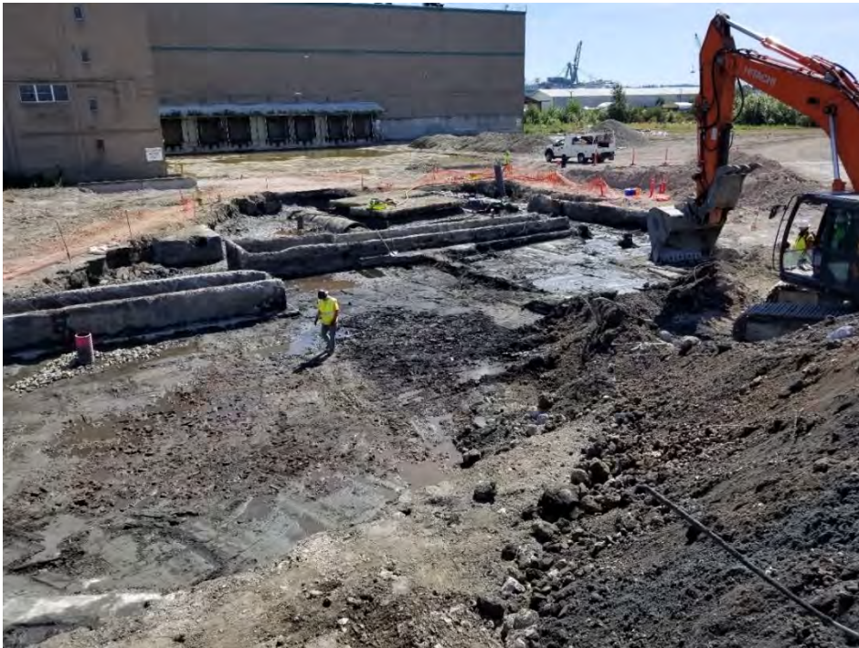
Photograph 9. South end of excavation, looking south.
