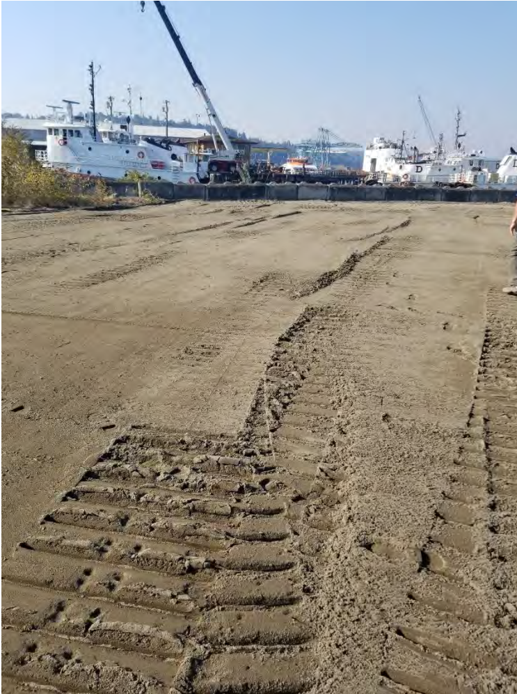
Photograph 14. Excavation backfilled, looking south, 9/14/2020.
