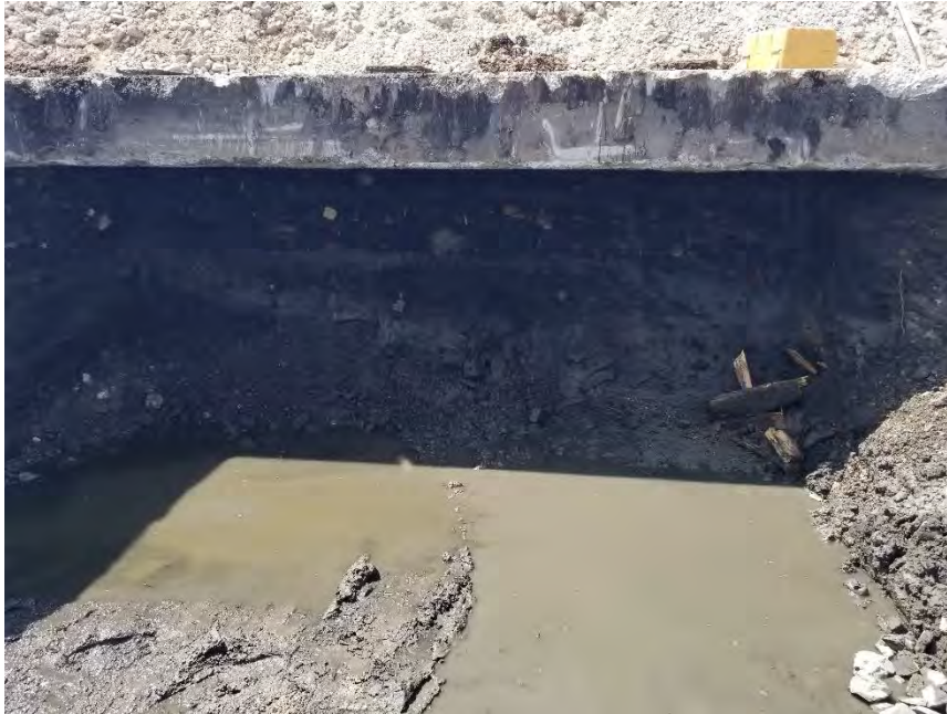
Photograph 3. West sidewall beneath foundation after second overexcavation, looking west.
