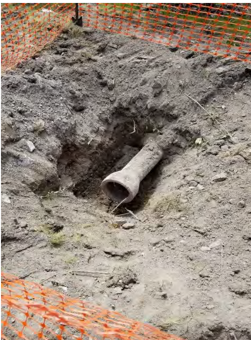
Photograph 6: Pipe B3 downstream of former catch basin, before being plugged.
