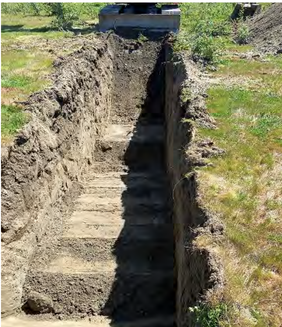
Photograph 4. Top of Pipe F exposed 75 feet east of bulkhead.
