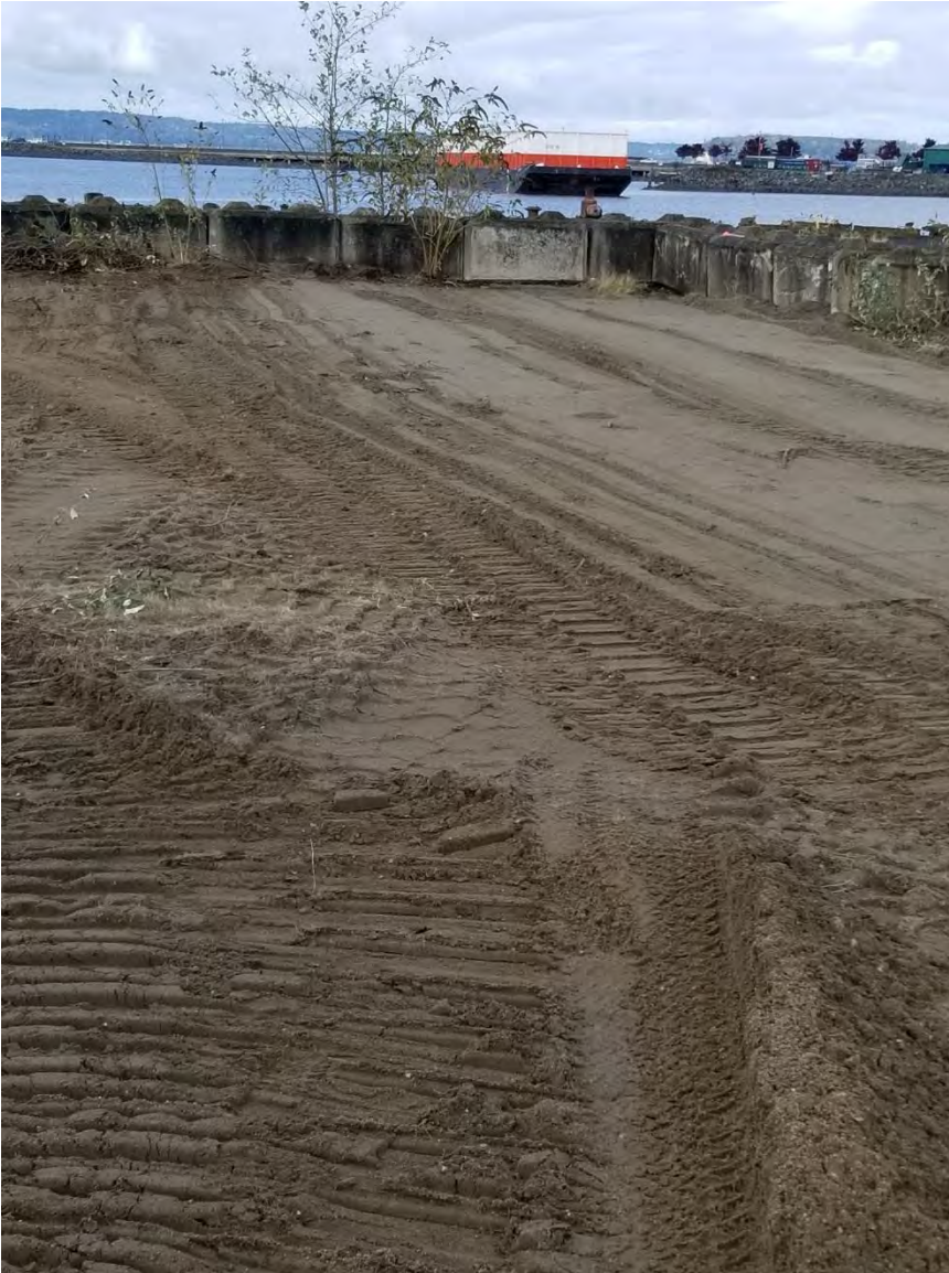
Photograph 6. BA-MW-7 excavation backfilled, 10/13/2020.
