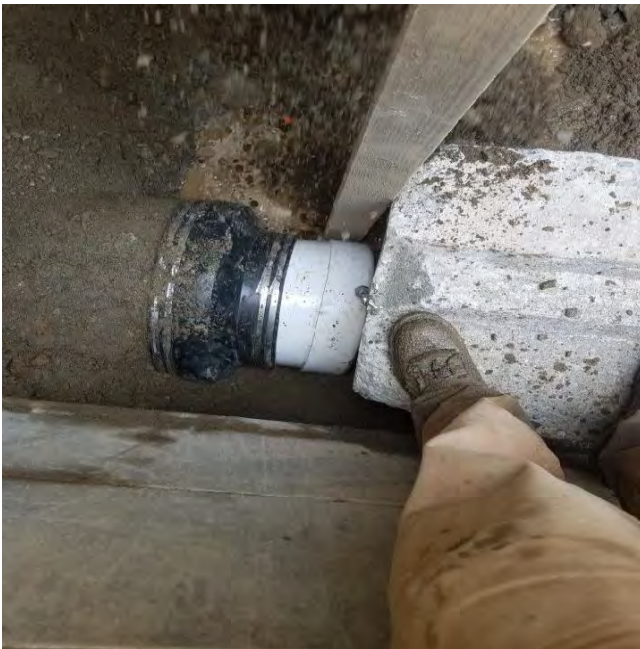
Photograph 4. Pipe K with “Fernco” plug and ecology block to brace the plug against tidal pressure.
