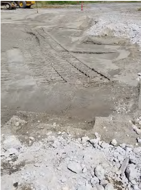
Photograph 6. CN-West excavation backfilled.
