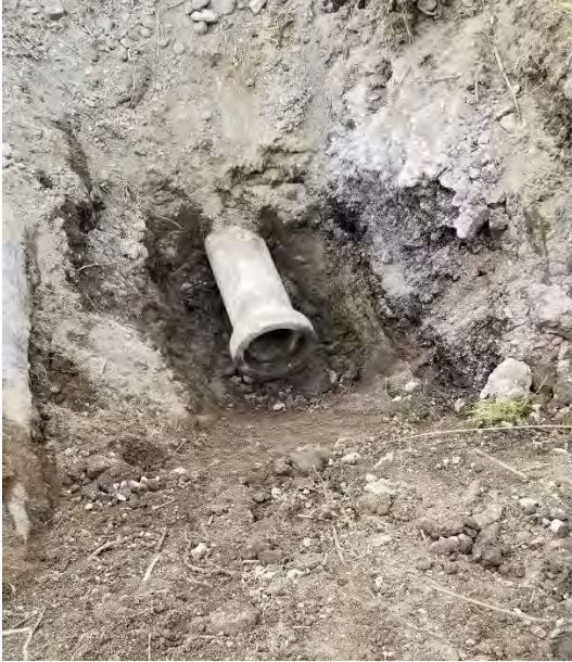
Photograph 3. Downstream Pipe B2 exposed, preplugging.
