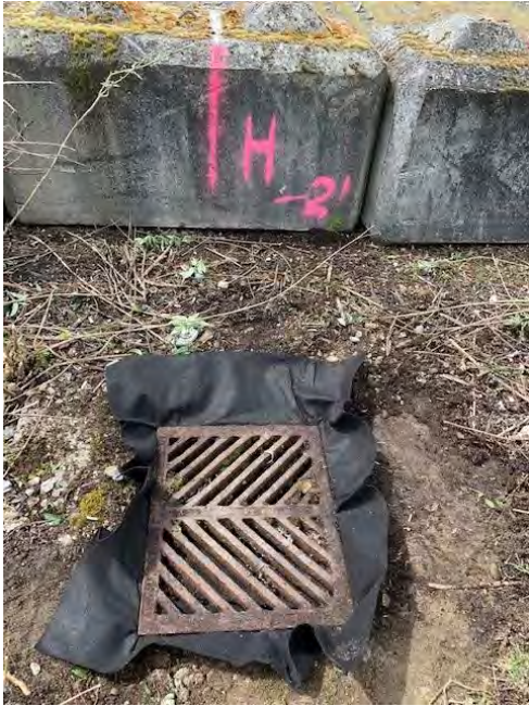
Photograph 1. Pipe H catch basin near bulkhead before excavation.
