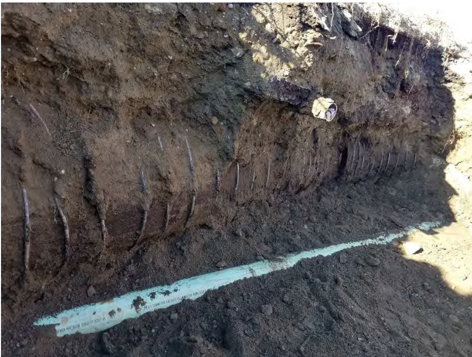
Photograph 11. Close up of wood stave Pipe C in southeasternmost sidewall.
