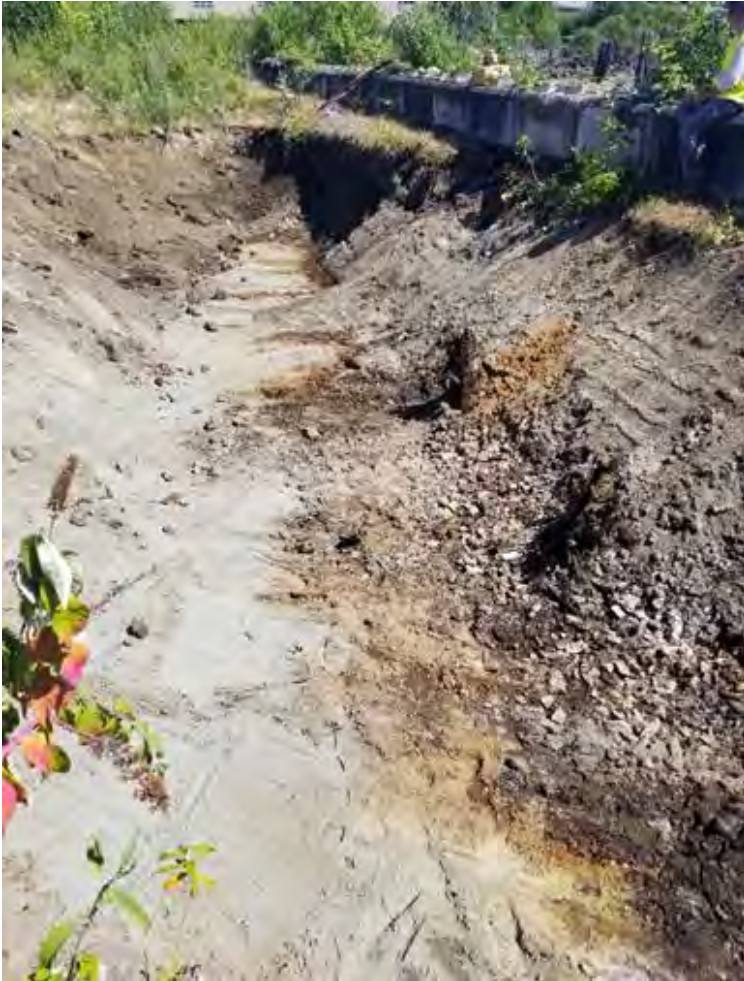
Photograph 3. South sidewall, start of excavation, looking east.
