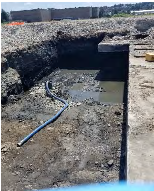
Photograph 4. Looking south in excavation after second overexcavation.
