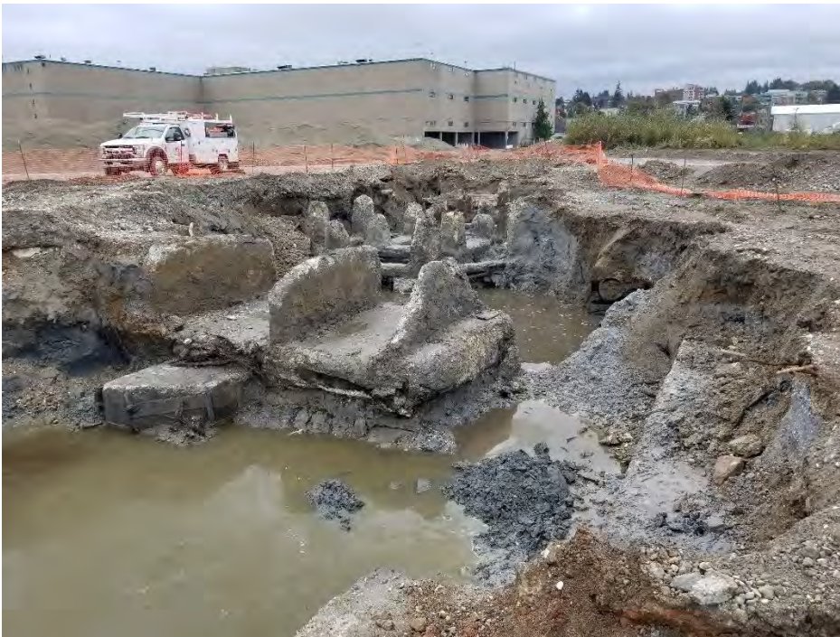
Photograph 17. View of south leg, looking south-southeast.
