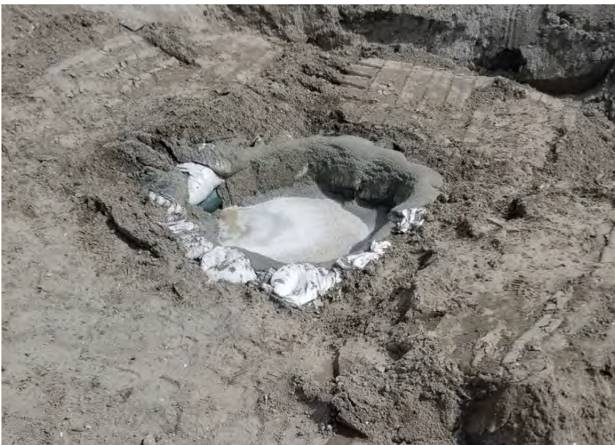
Photograph 12. Top of CDF plug at bulkhead.
