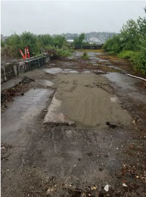
Photograph 7. Vault backfilled with Parcel O sand.
