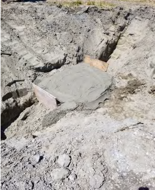
Photograph 7. Pipe C CDF plug at station 11+31.
