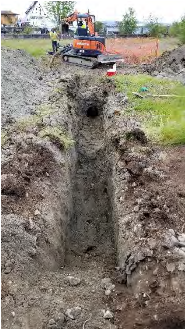
Photograph 2. Fuel oil pipe trench, after pipe removal.
