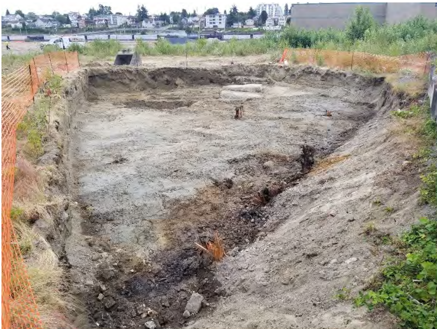
Photograph 2. Excavation looking east prior to overexcavation.
