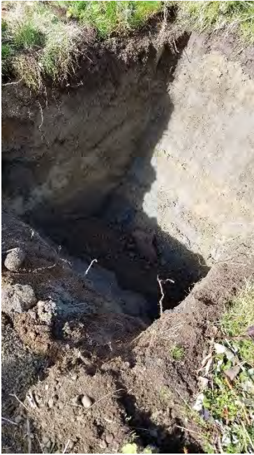
Photograph 1. Excavation for pipe Q, ~7 feet east of bulkhead, no pipe found.
