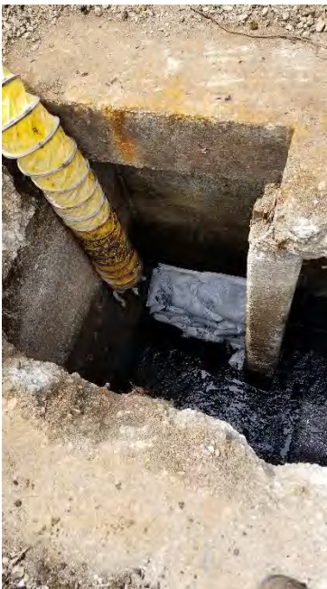
Photograph 4. Jet set concrete in Pipe M placed downstream of vault.
