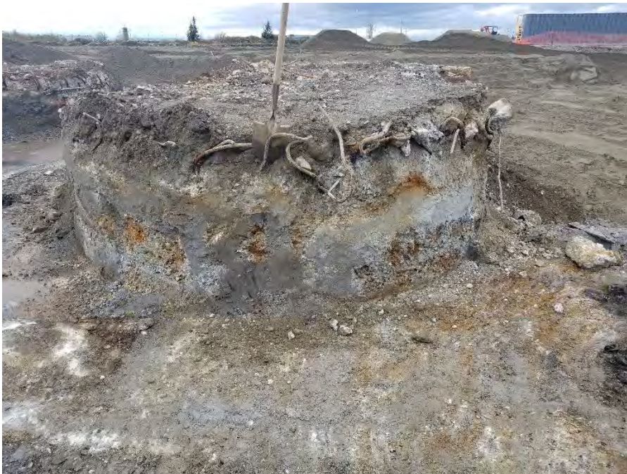
Photograph 6. North sidewall of extension between south leg of BBH Area and GFB12 Area, view looking north.
