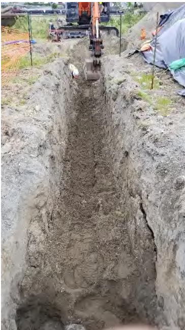
Photograph 2. Trench after removal of pipe E.
