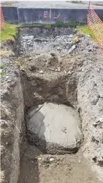
Photograph 4. Pipe E plugged with CDF ~7 feet east of bulkhead.
