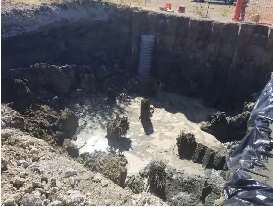
Photograph 3. Final excavation limits on 8/28/2020, view looking southwest.
