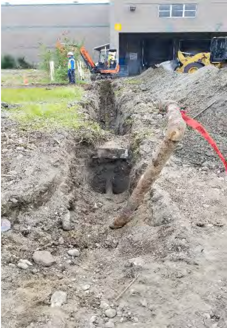
Photograph 1. Fuel oil pipe exposed, in place.
