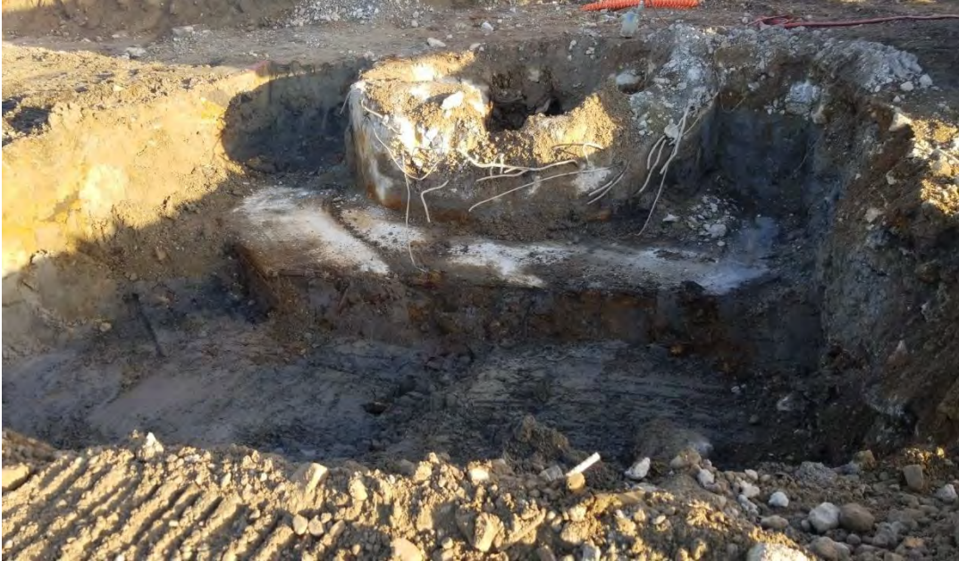
Photograph 3. Limits after first overexcavation, view looking north.
