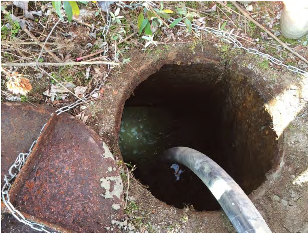
Photo 2: Typical CDF Fill of Pipes and Manhole
