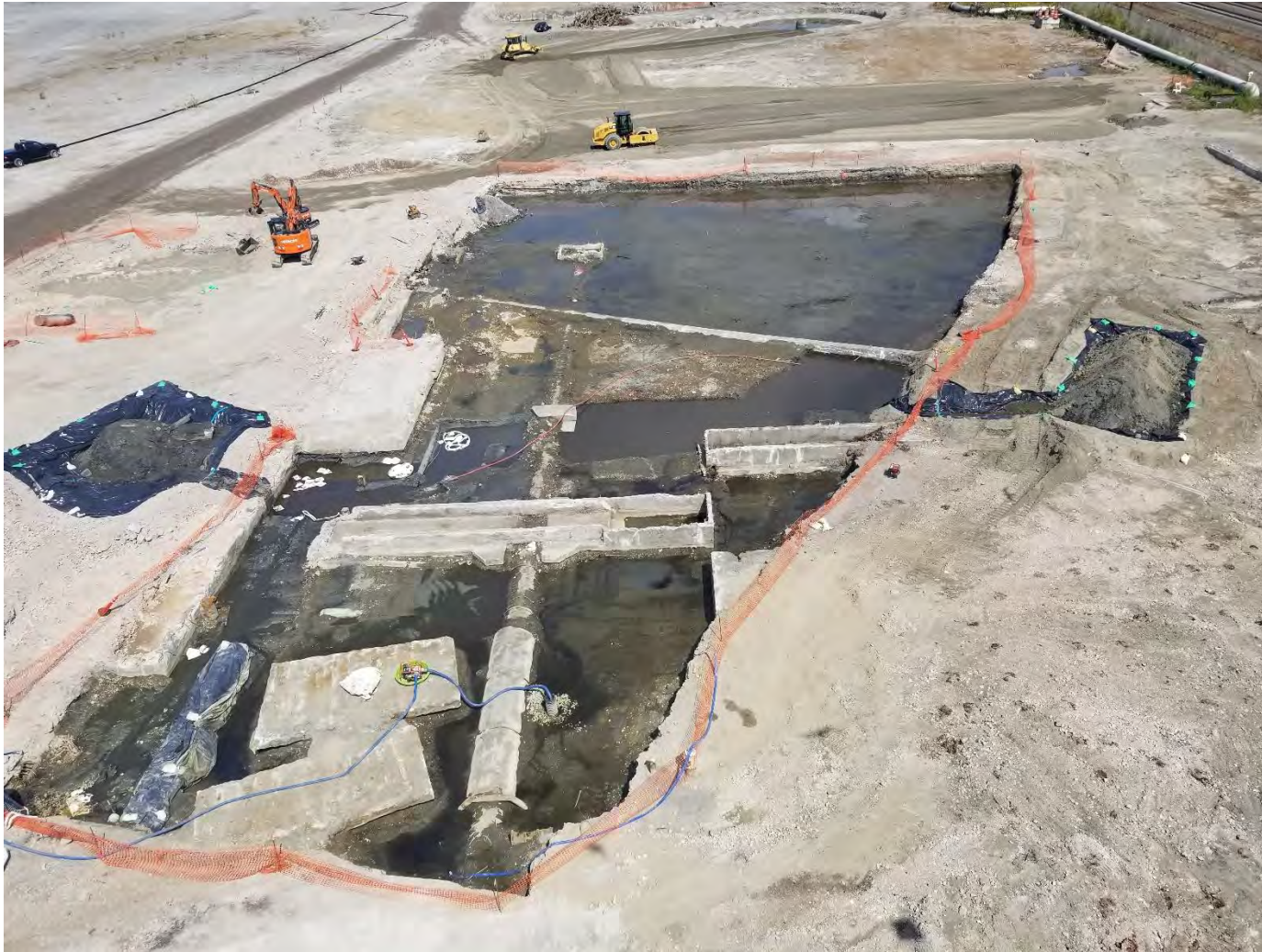
Photograph 13. Aerial view of excavation taken on 8/12/2020, view looking north.
