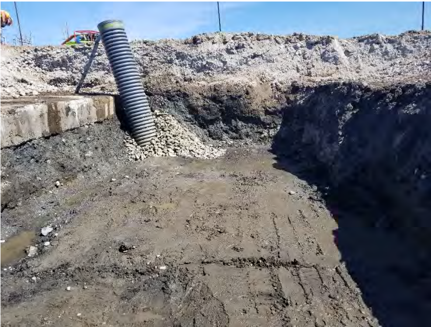
Photograph 2. Initial dewatered excavation, conveyor foundation on left, looking north.
