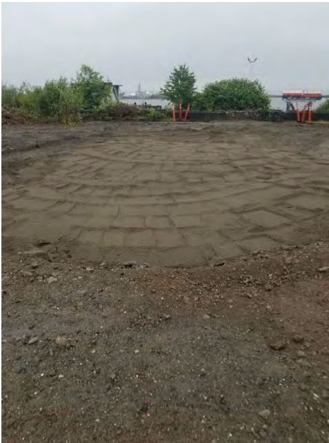
Photograph 8. Backfilled trench from removed pipe inland from vault.
