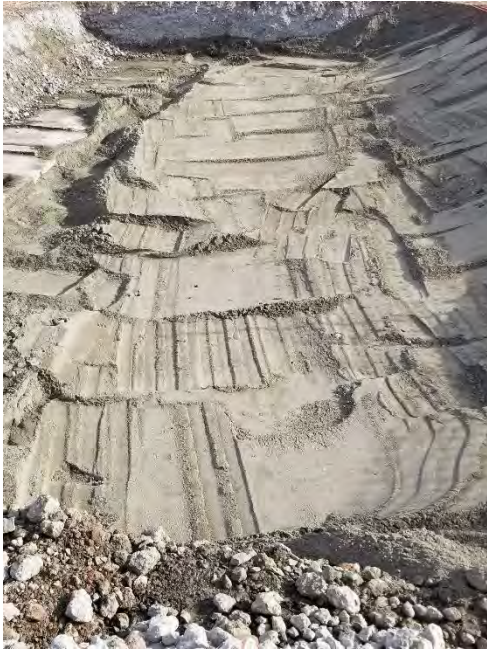
Photograph 5. Log Pond Chip Conveyor excavation being backfilled, 7/14/2020.
