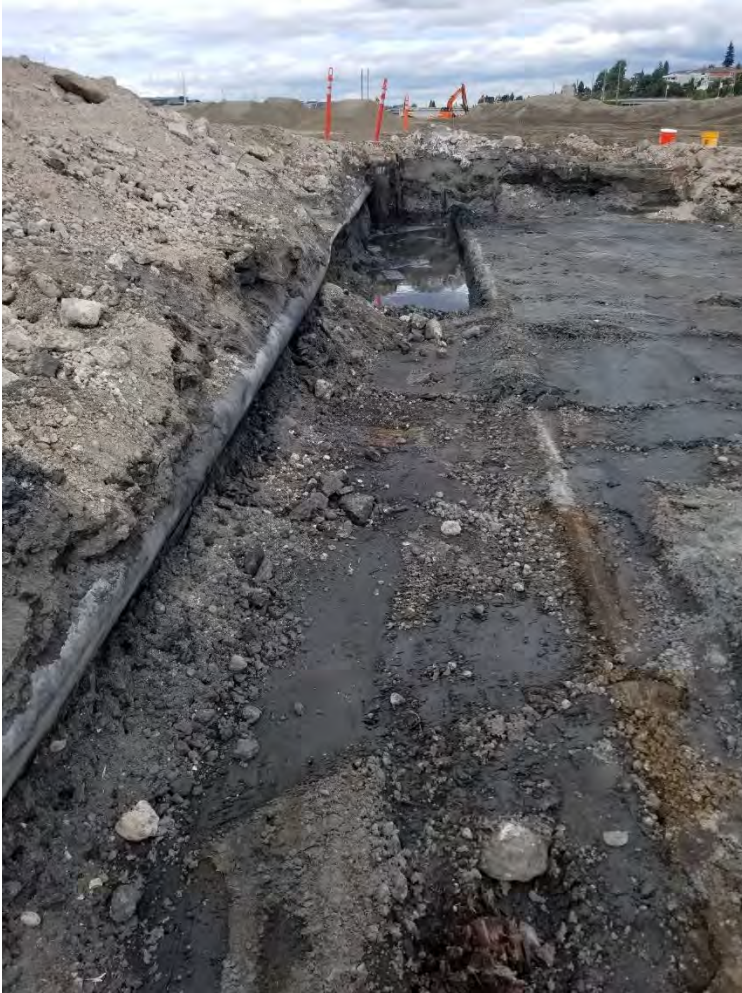
Photograph 16. Limits of excavation on 8/20/2020 for removal of NW bunker fuel pipes.
