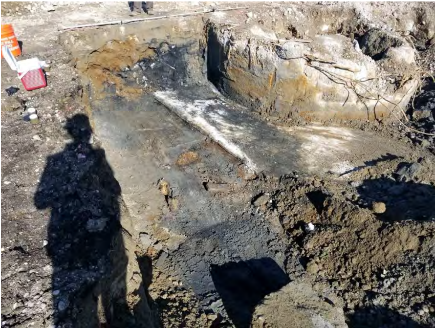
Photograph 4. Limits after first overexcavation, view looking northwest.
