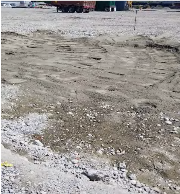
Photograph 5. CN-East excavation backfilled.
