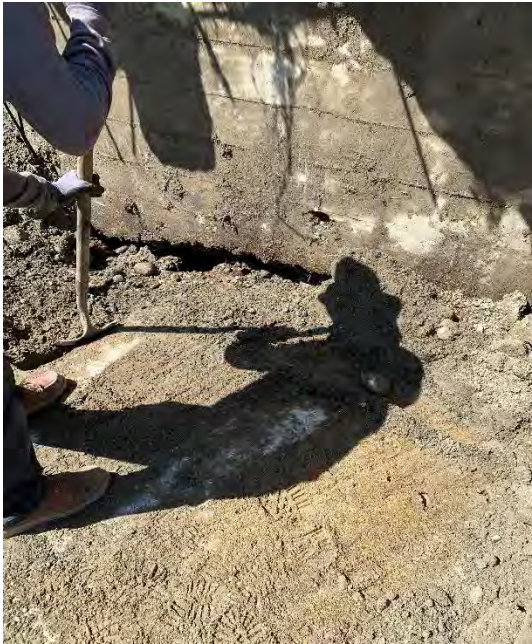
Photograph 1. Exposing top of Pipe F, east side of the bulkhead.
