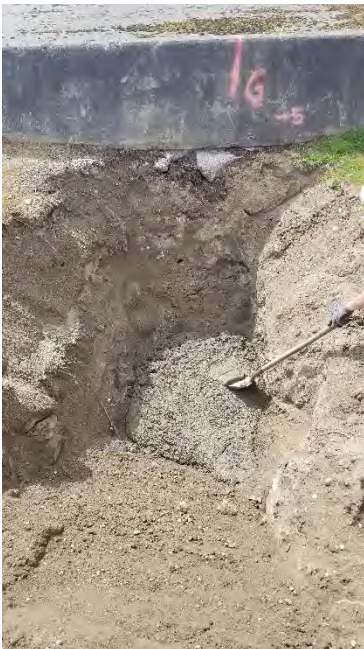
Photograph 4. Pipe G CDF plug at bulkhead .
