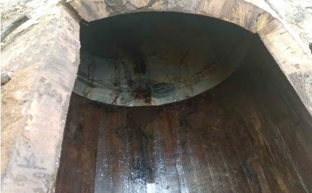
Photograph 3. Pipe C after vector cleaning (1).
