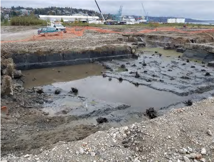
Photograph 14. View across main BBH Area, looking southwest towards the south leg of the excavation area.
