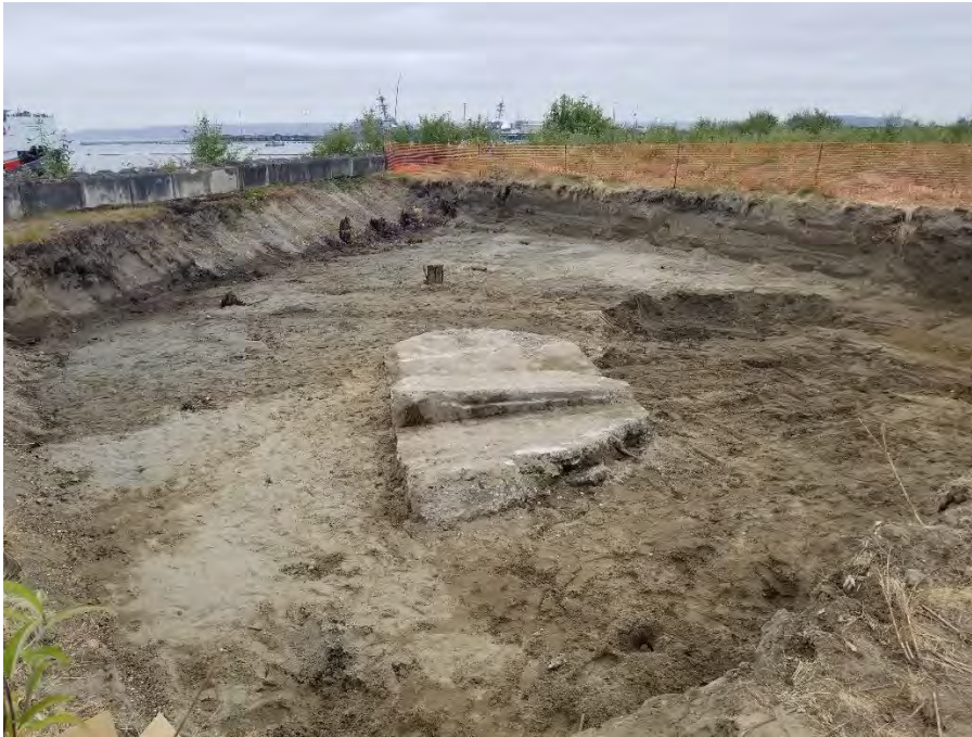
Photograph 1. Large concrete foundation elements extending beneath excavation base, looking west.
