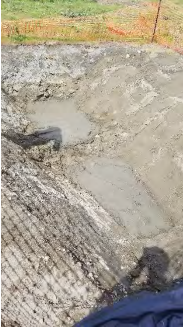
Photograph 5. Pipe E T-joint (at 45 feet) plugged on both ends with CDF.
