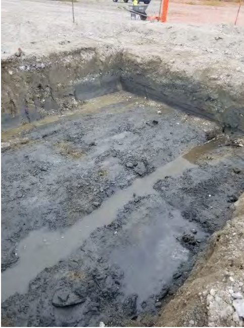
Photograph 3. CN-East excavation, dewatering turned off.
