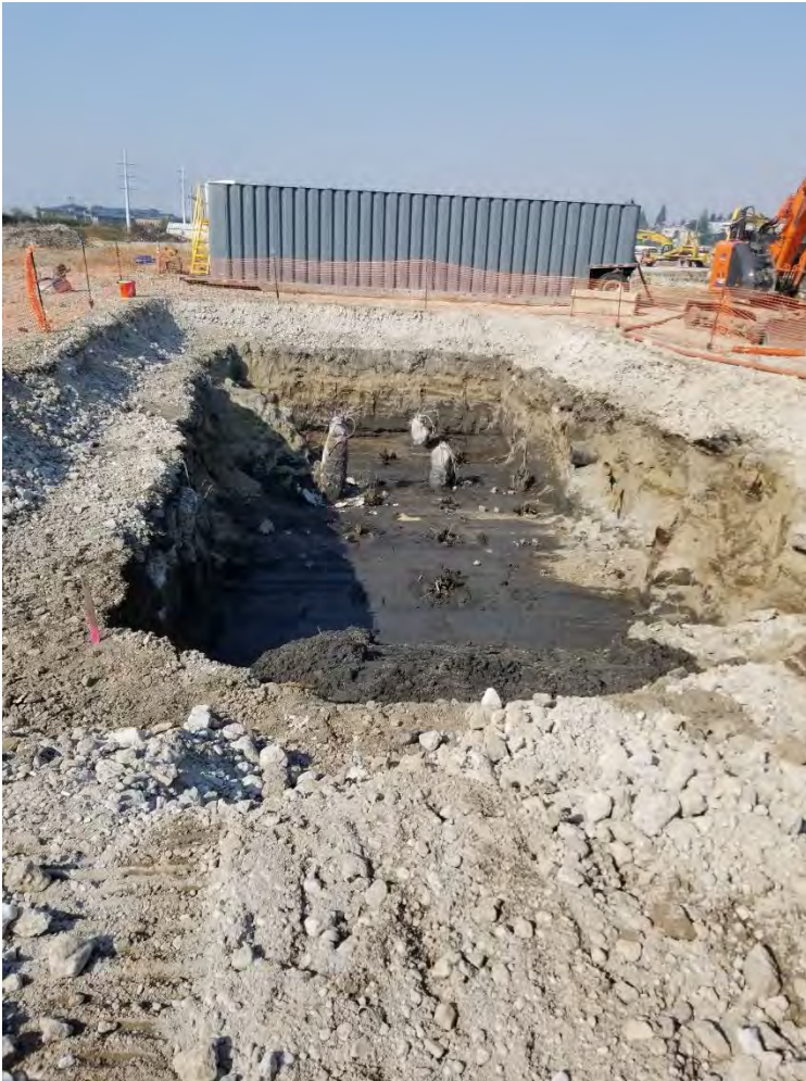
Photograph 5. Northern leg of BBH Area excavation, view looking north.
