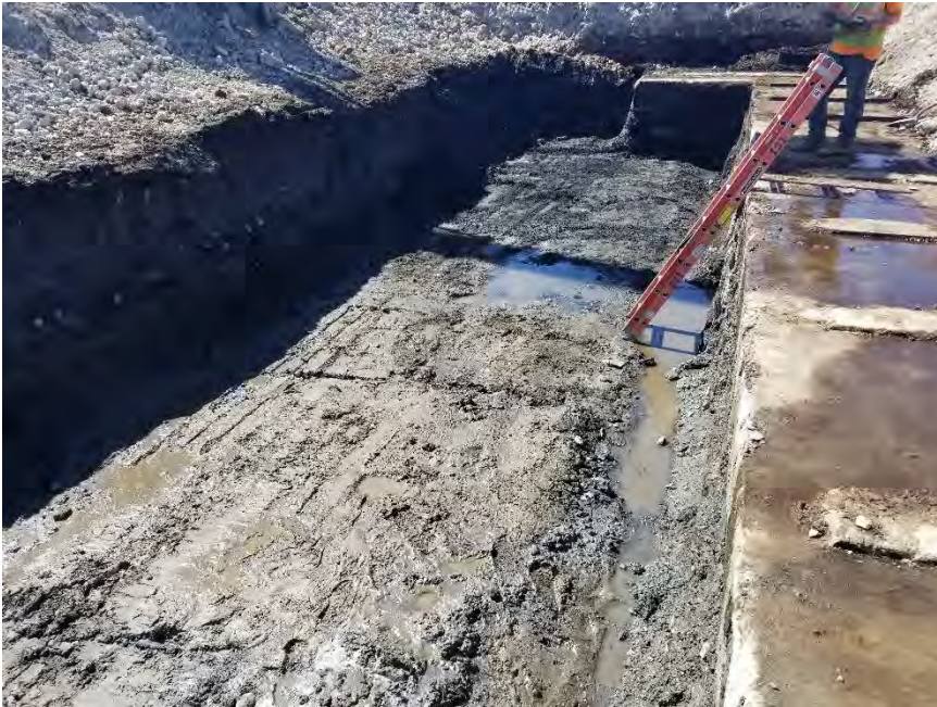
Photograph 1. Initial dewatered excavation, conveyor foundation on right, looking south.
