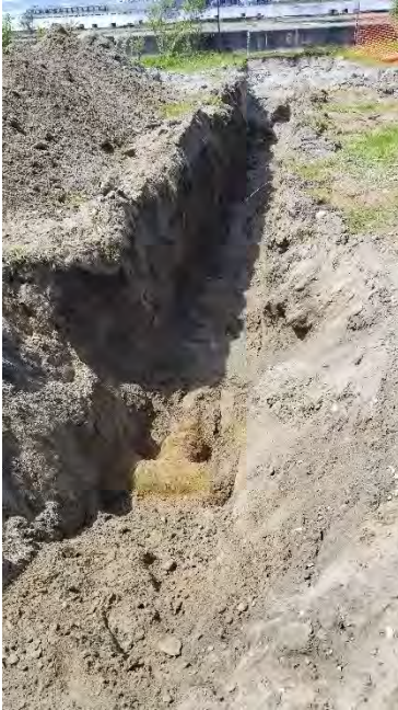
Photograph 1. Pipe E, uncovered. T-junction at ~45 feet inland shown.
