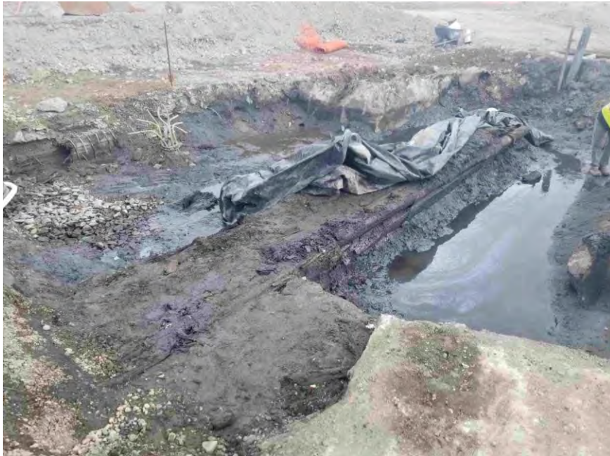
Photograph 7. One Bunker C fuel pipe encountered within wooden conduit, looking north.
