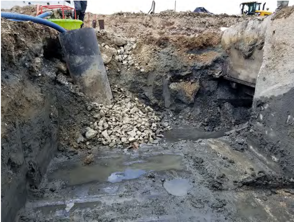
Photograph 5. West sidewall on south side of concrete wall, view looking west.
