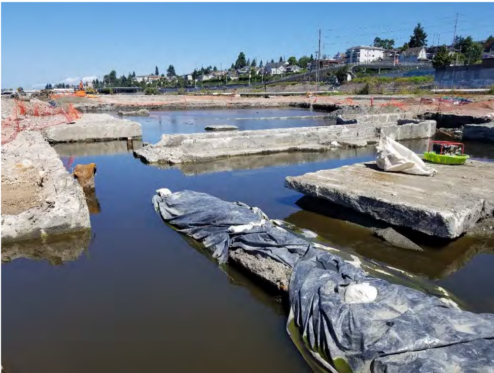
Photograph 12. Open excavation prior to dewatering on 8/10/2020, view looking northeast.
