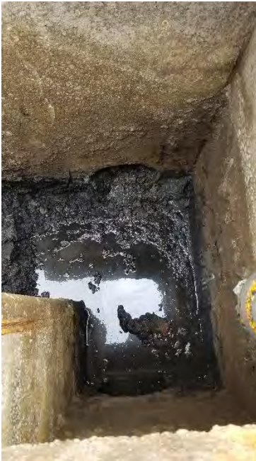
Photograph 3. Pipe M entering/exiting vault near shoreline.
