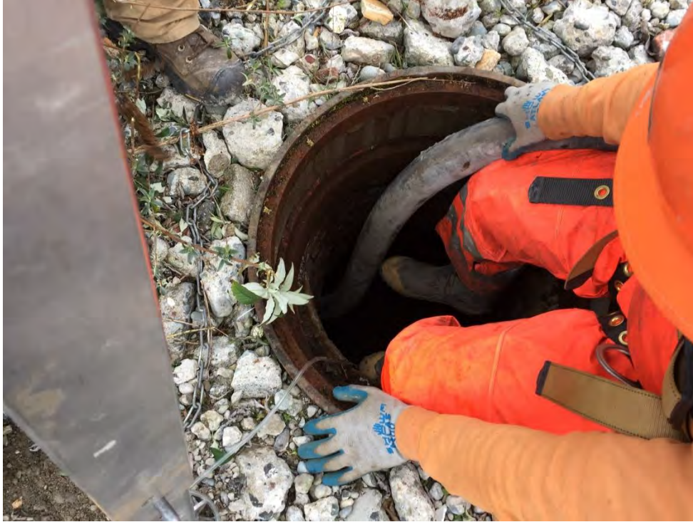
Photo 1: Preparing a manhole for CDF Fill
