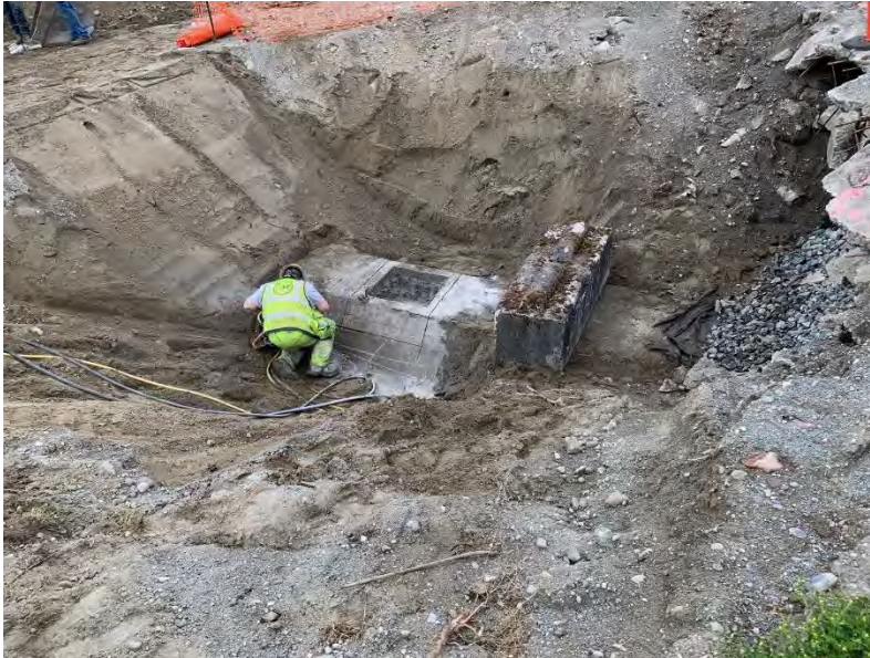
Photograph 5. Saw cutting 16+ inches of concrete 15 feet east of bulkhead.
