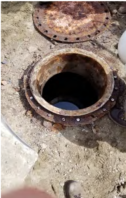
Photograph 2. Open Pipe C manhole (adjacent to station 10+98).
