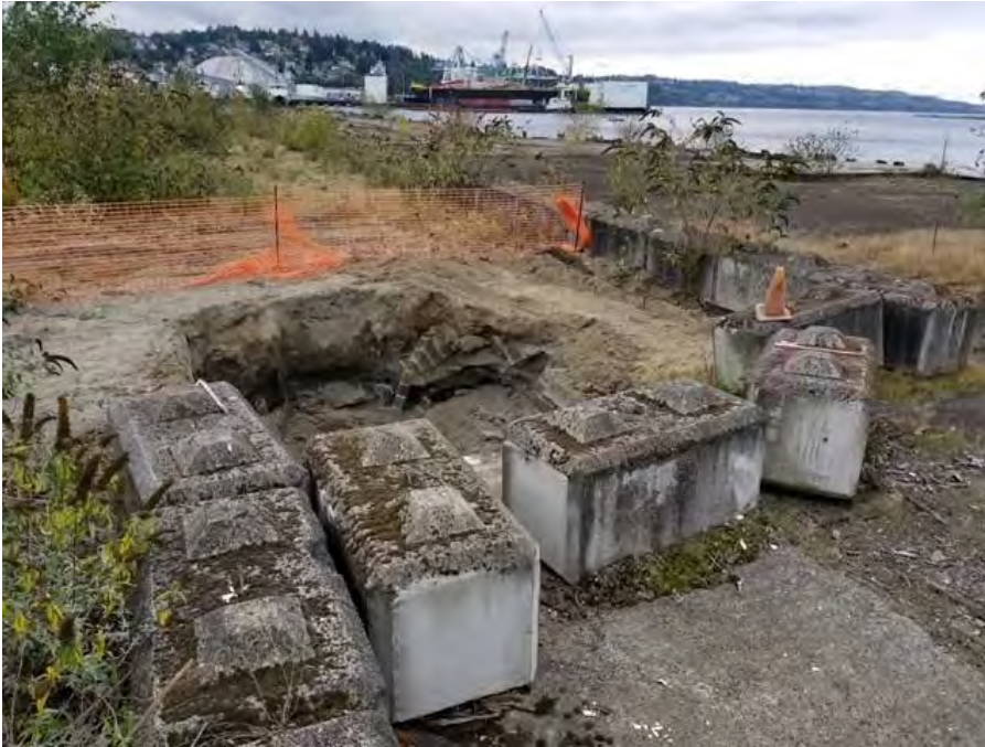
Photograph 3. Initial excavation, 10/5/2020, view looking southwest.
