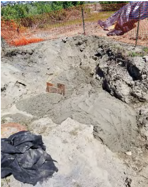
Photograph 6. Pipe C CDF plug at station 10+98.
