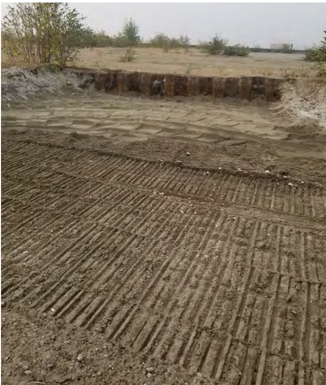
Photograph 4. Excavation backfilled, 9/16/2020, view looking west.
