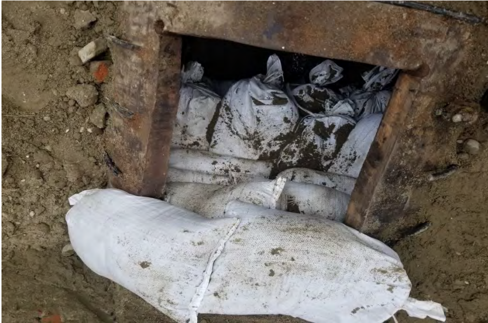
Photograph 5. One Pipe C sandbag dam prior to placing CDF between dams.
