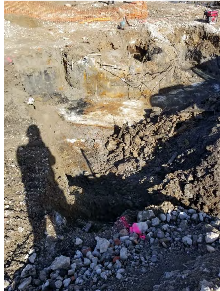
Photograph 2. Initial excavation limits, looking northeast.
