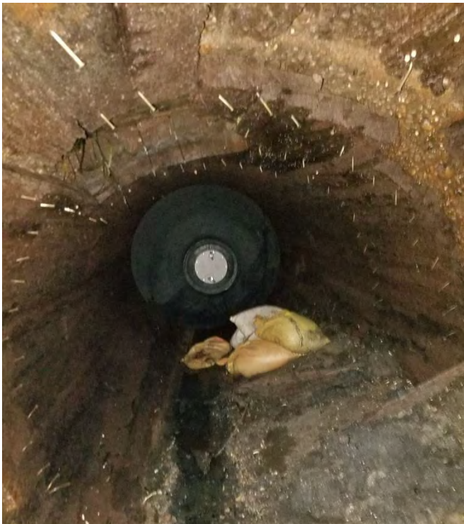
Photograph 10. Pneumatic plug in place at bulkhead.
