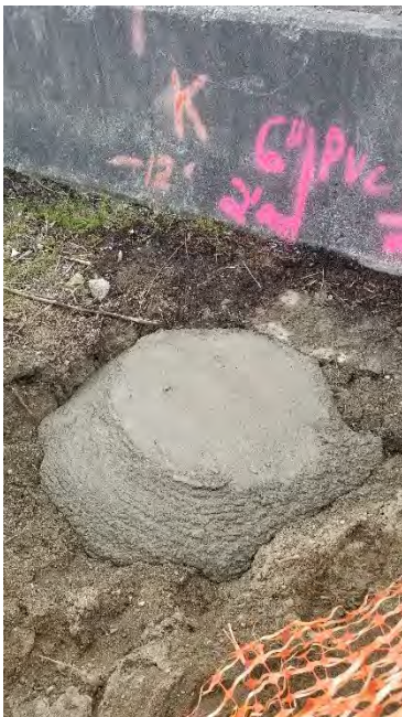
Photograph 2. Pipe L plugged with CDF adjacent to bulkhead.
