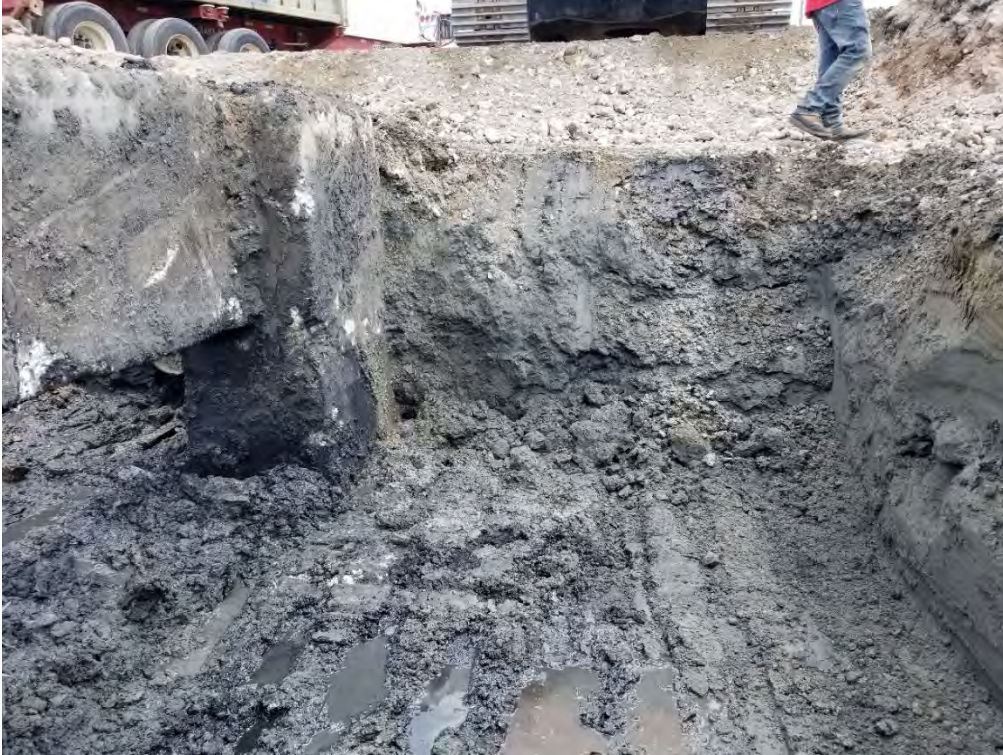
Photograph 7. East sidewall on south side of concrete wall, view looking east.
