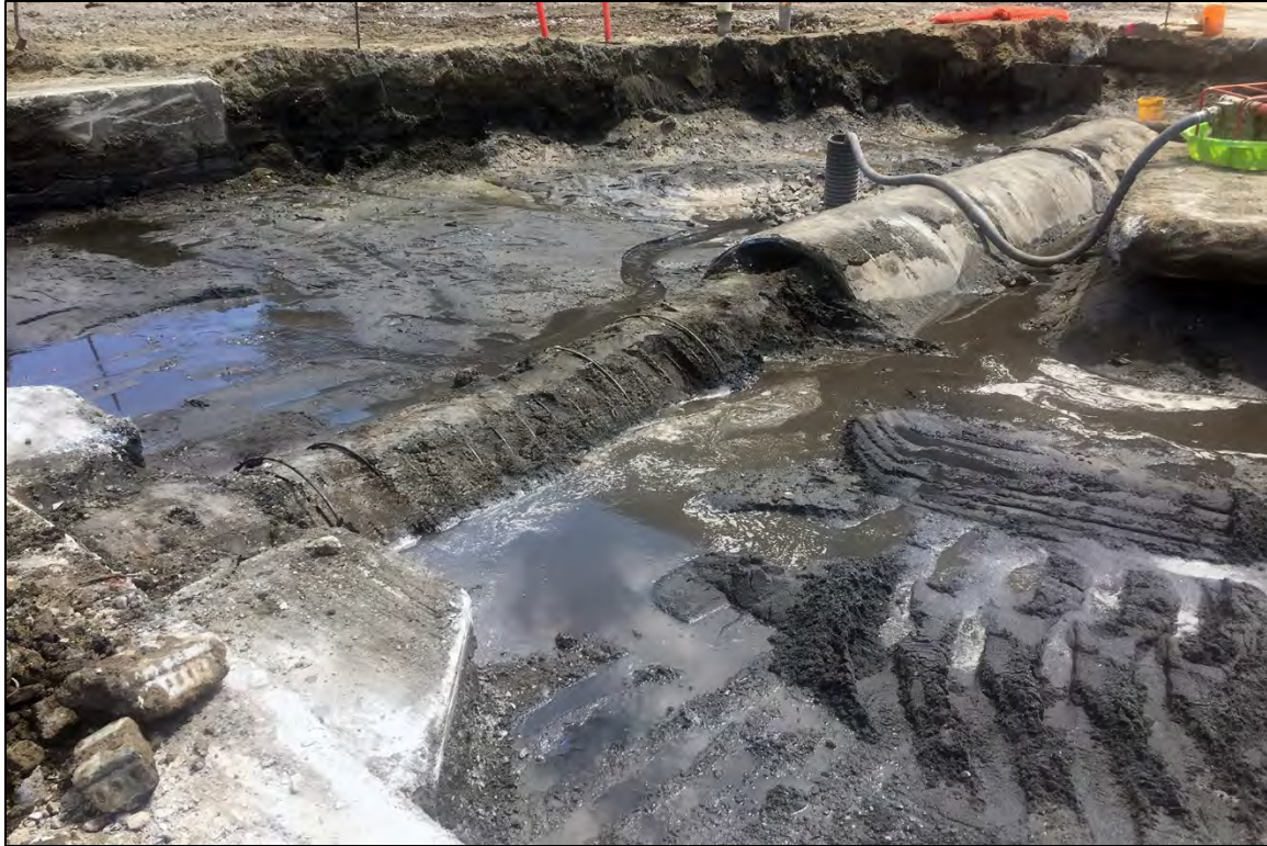
Figure 9. Overview of wood-stave pipe in the CMS Area.
