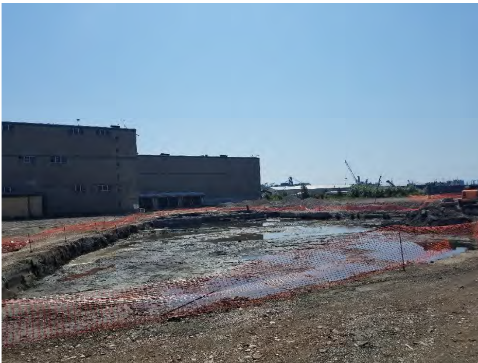
Photograph 10. Open excavation extent on 7/30/2020, view looking southwest.
