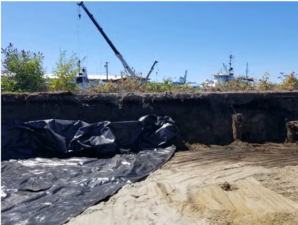
Photograph 6. South sidewall following removal of ecology blocks and second overexcavation.
