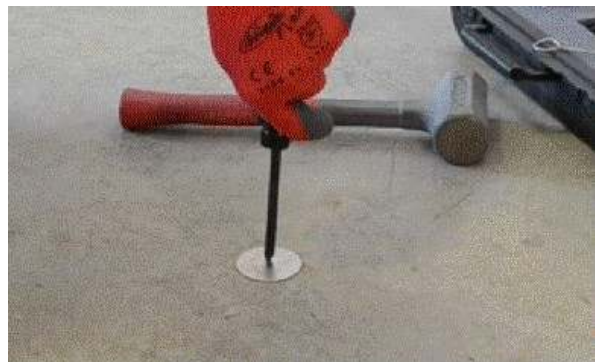
Figure 5. Tightening the Secured Cover.
